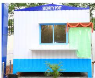
Security Post @ Entrance
