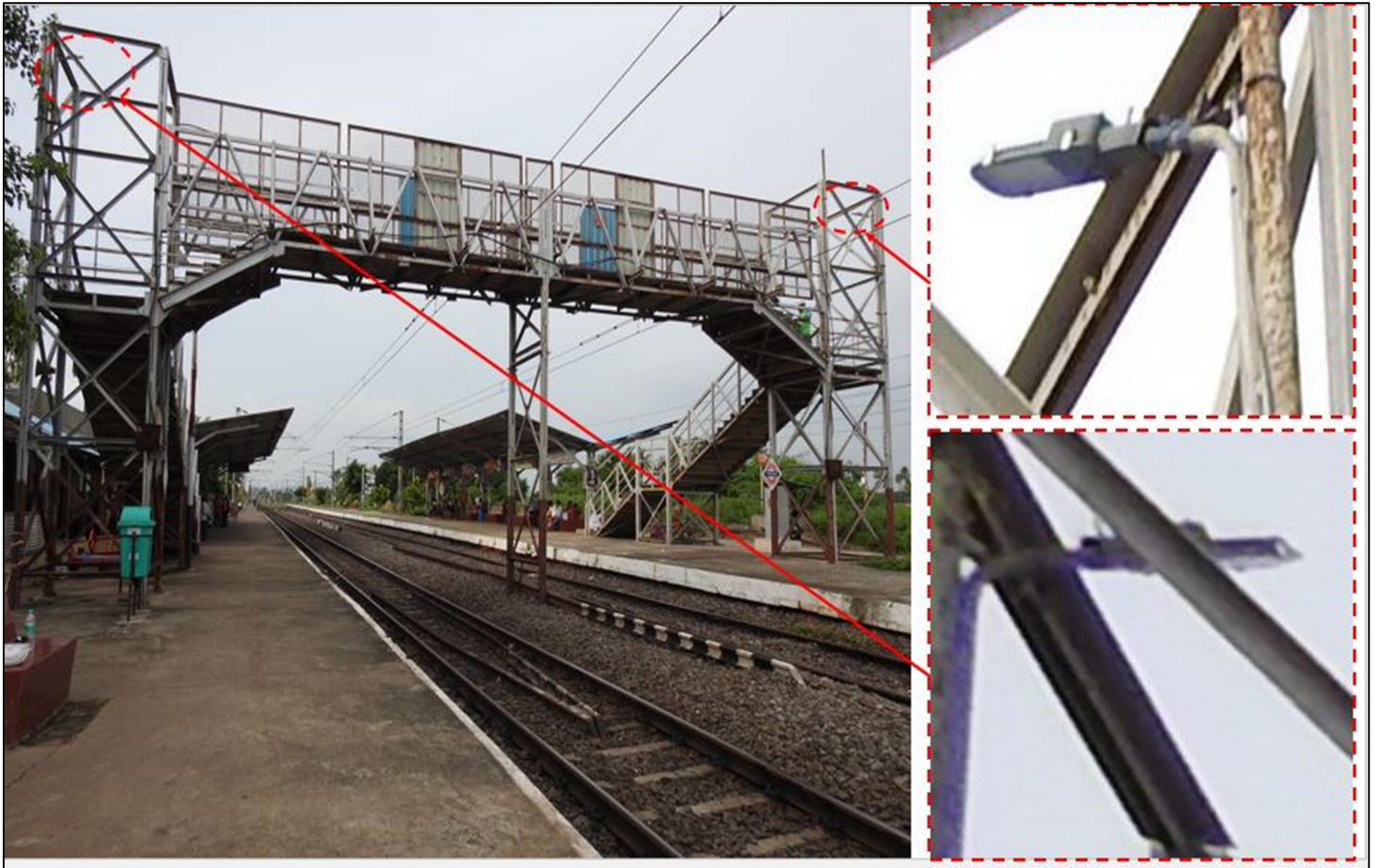
Fig 1: Light Post attached to landing Trestles Pf. 1
