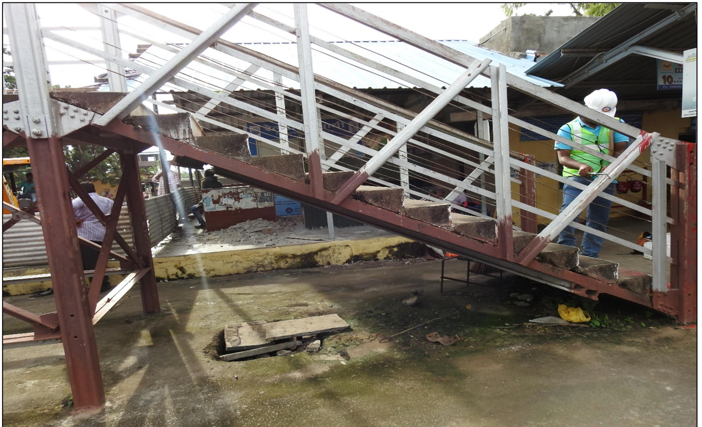
Fig 2: Red oxide coating observed at FOB
