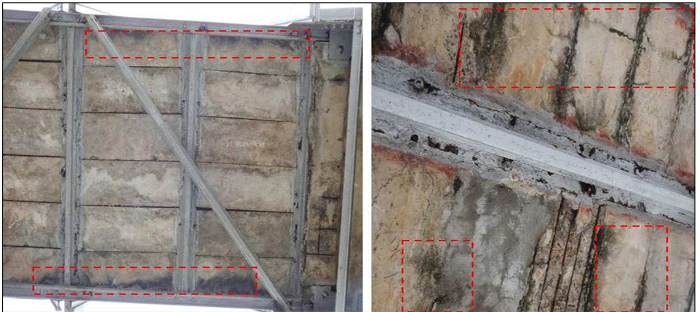
b) Spalling and Cracks Observed at Stair case 2
