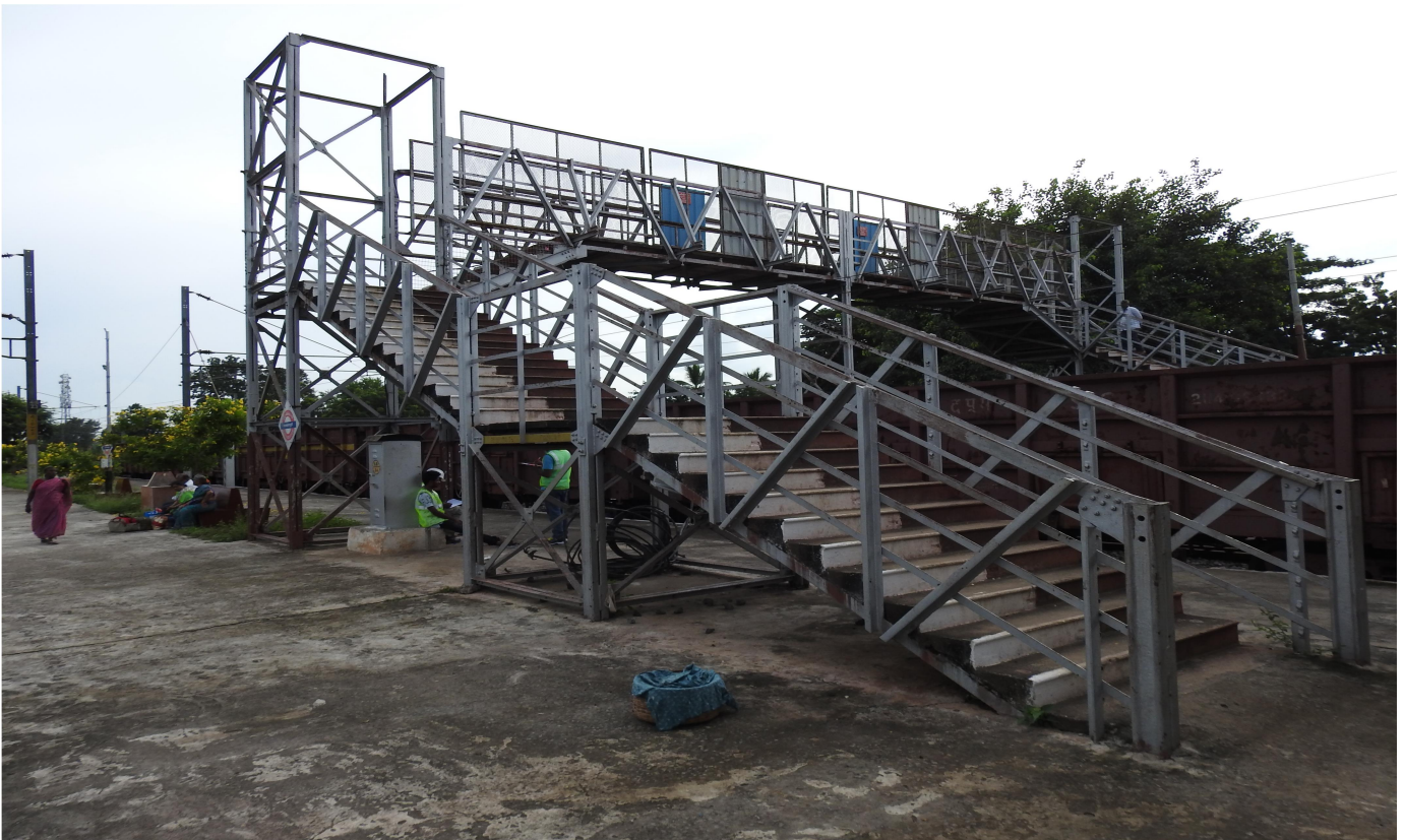
Fig 8: Railing, Trestle of FOB
