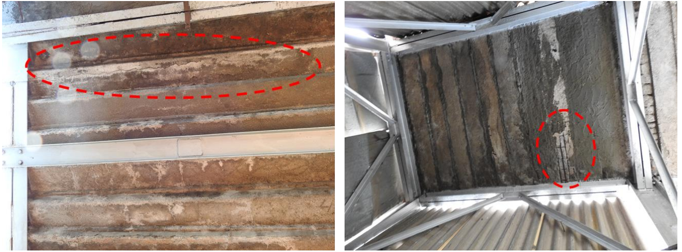
Fig 3.7: Rebar exposure under staircase
