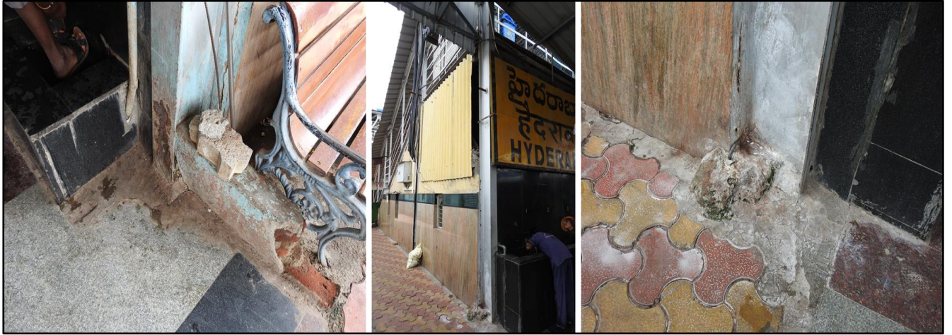
Fig 1.4: Column is merged in platform flooring
