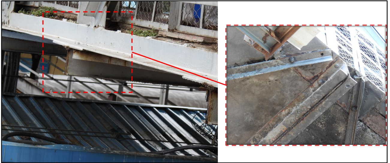
Fig 1.6: Main and Secondary girder with joint details
