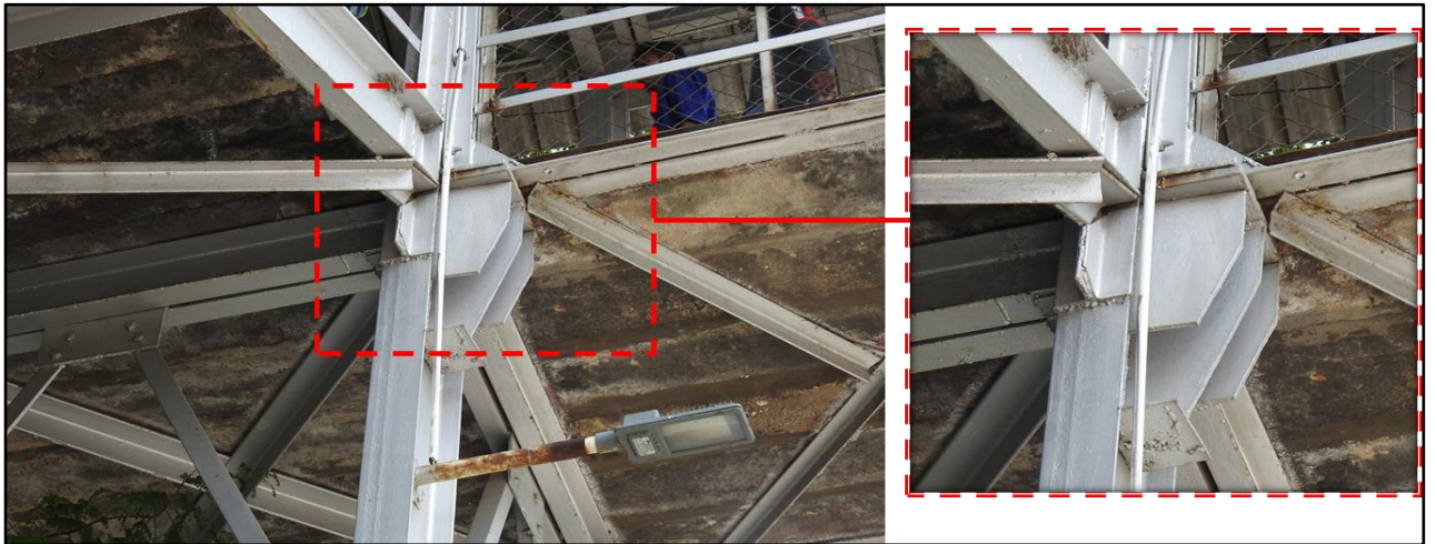
Fig 1.7: Beam- column joint
