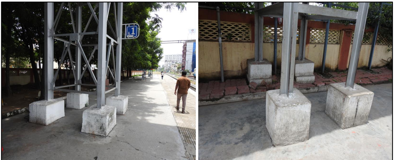
Fig 1.4: Concrete encasements
