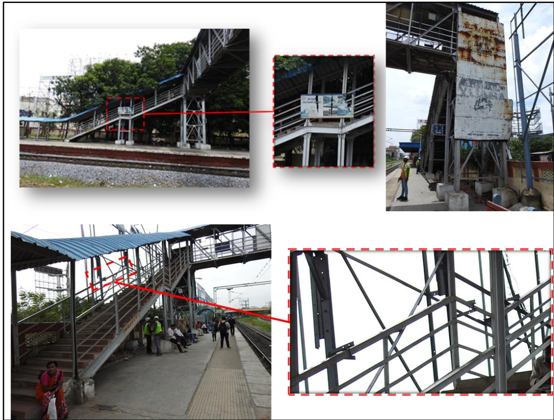
Fig 1.2: Load of Advertising Hoarding and staircase details
