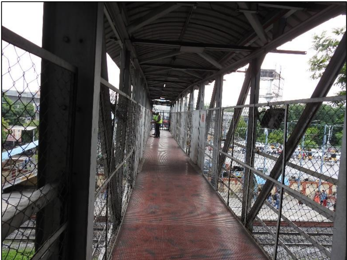
Fig 1.3(a): Galvanized wire mesh and Flooring
