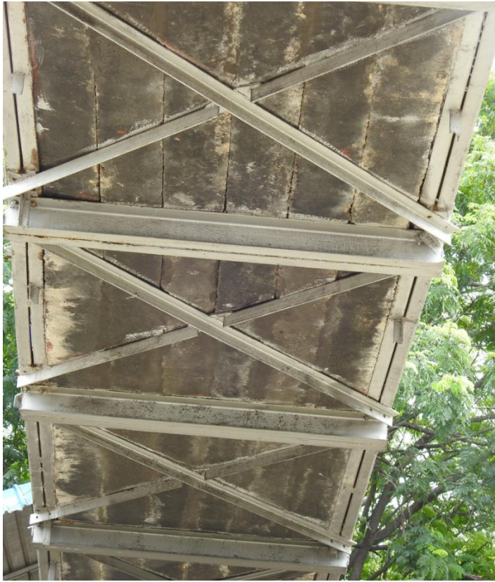
Fig 3.3 Leaching observed at precast panels
