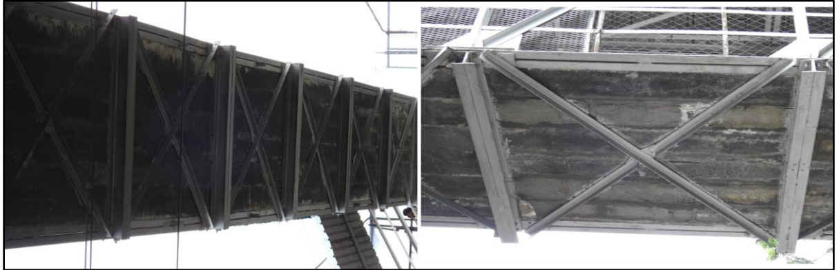
Leaching effect and minor cracks observed in Pre-cast slab panels
