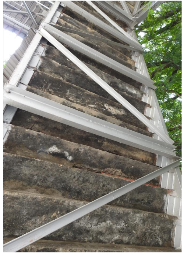
Fig 3.3 Leaching observed at precast panels
