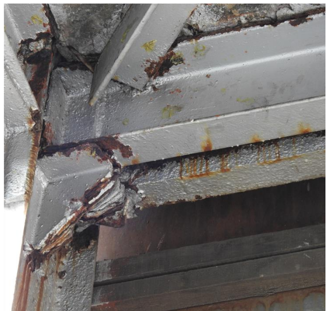
Fig 3.4 Corrosion of cleat angle at beam column joint
