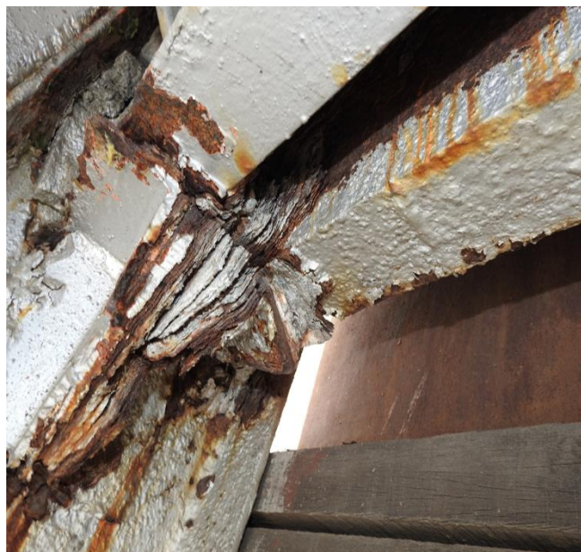
Fig 3.4 Corrosion of cleat angle at beam column joint
