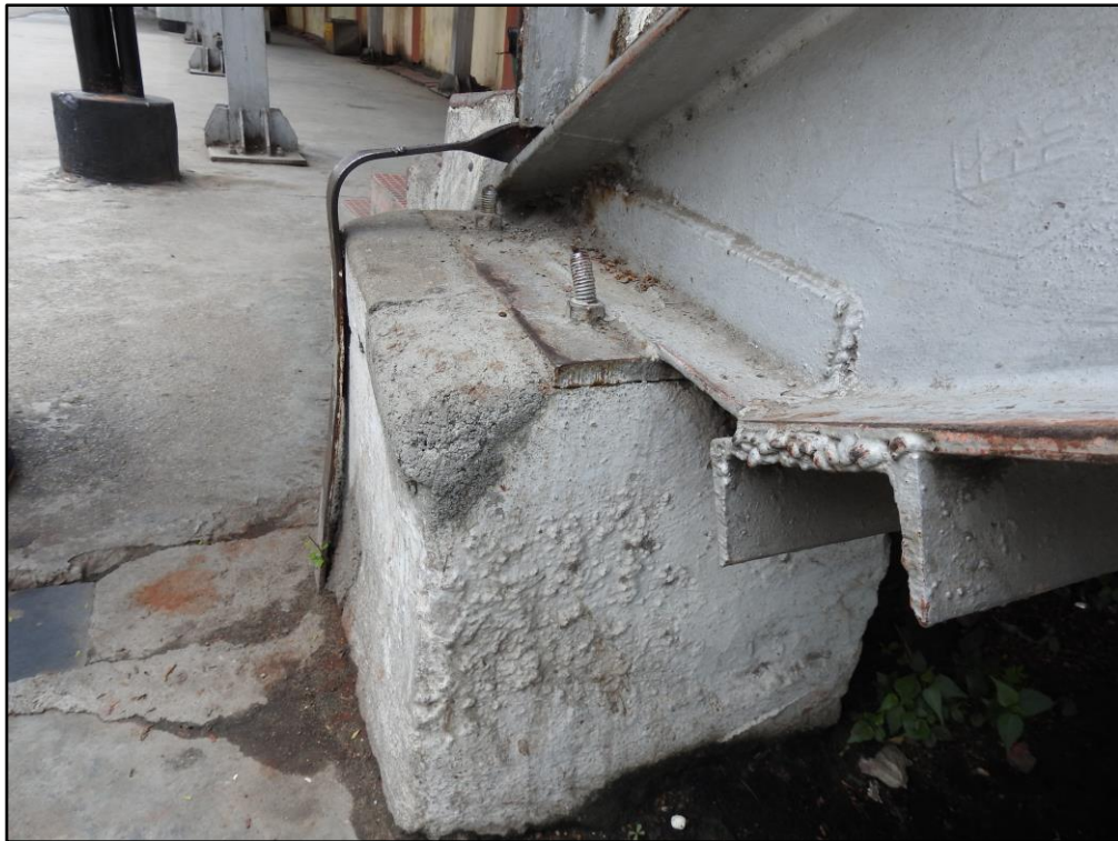
Fig 1.3(b): Base plate at staircase
