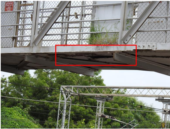
Fig 2.4: Locations of Sacrificial plate Deteriorations
