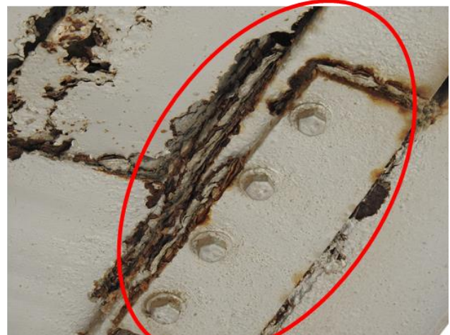
Fig 2.2: Locations of Splice joint and bottom chord Deteriorations
