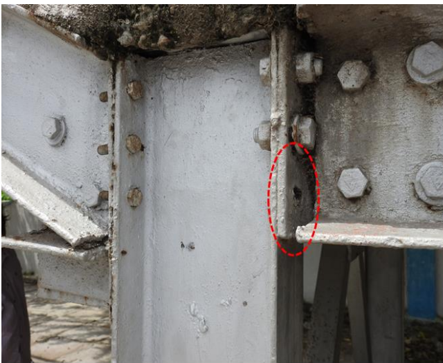
Fig: 2.5 missing of bolts at mid land at staircase stinger beam
