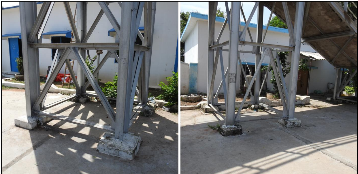
Fig 1.3: Trestles and their protection with concrete encasement
