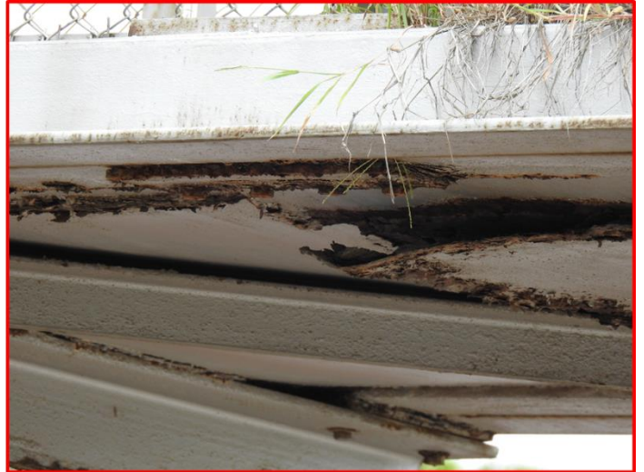
Fig 2.4: Locations of Sacrificial plate Deteriorations
