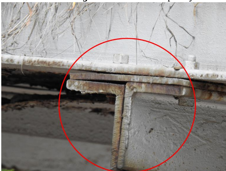
Fig 2.3: Locations of floor beam Deterioration
