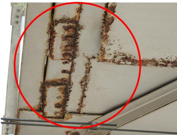
Fig 2.2: Locations of Splice joint and bottom chord Deteriorations
