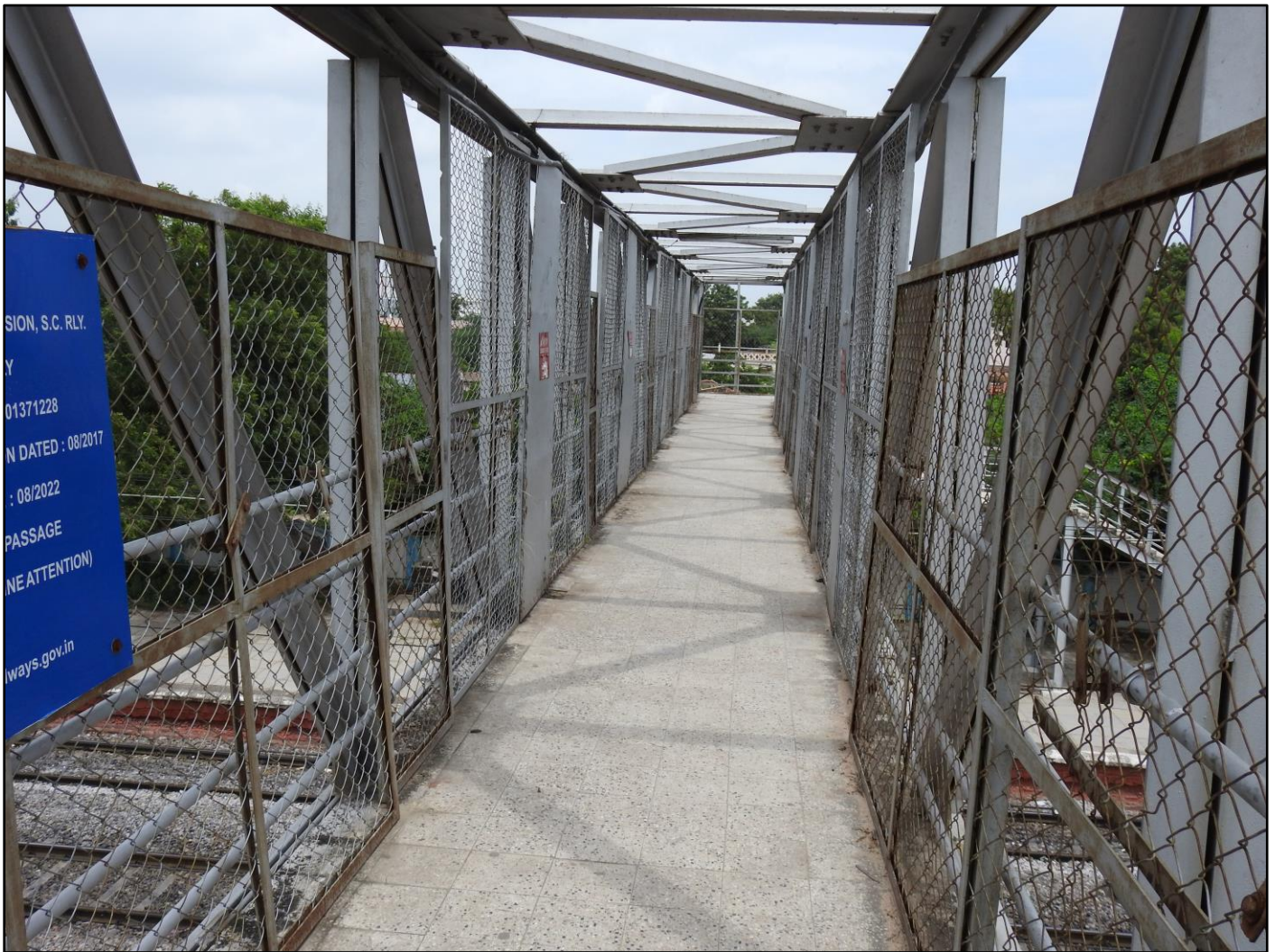
Fig 1.2: Protective screening mesh for passenger and flooring and roof elements
