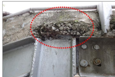
Fig: 2.5 missing of bolts at mid land at staircase stinger beam
