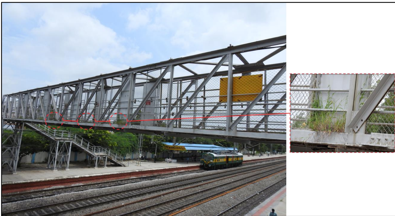
Fig 1.6: Vegetation at truss level and shape of truss
