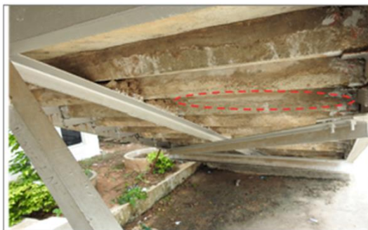
Fig: 2.5 missing of bolts at mid land at staircase stinger beam
