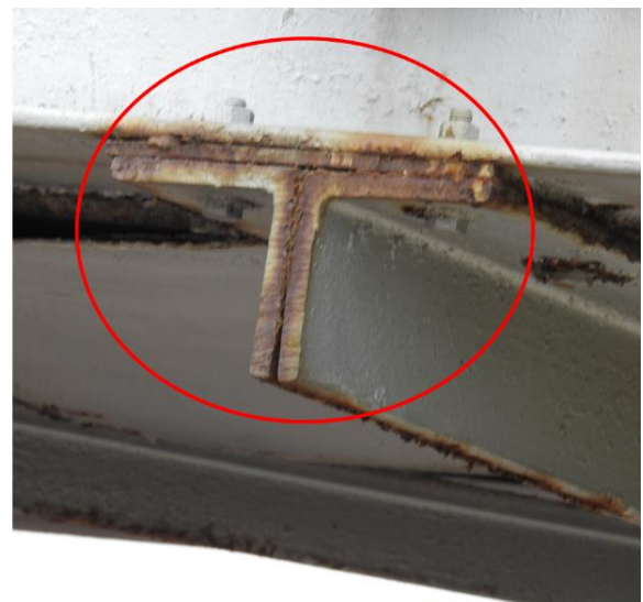
Fig 2.3: Locations of floor beam Deterioration
