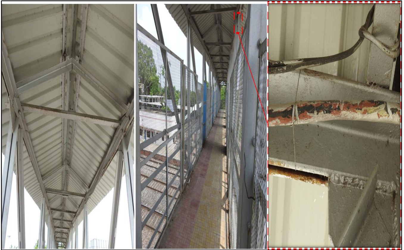
Fig 1.1: Cables, Roof truss, Flooring and Protective screen
