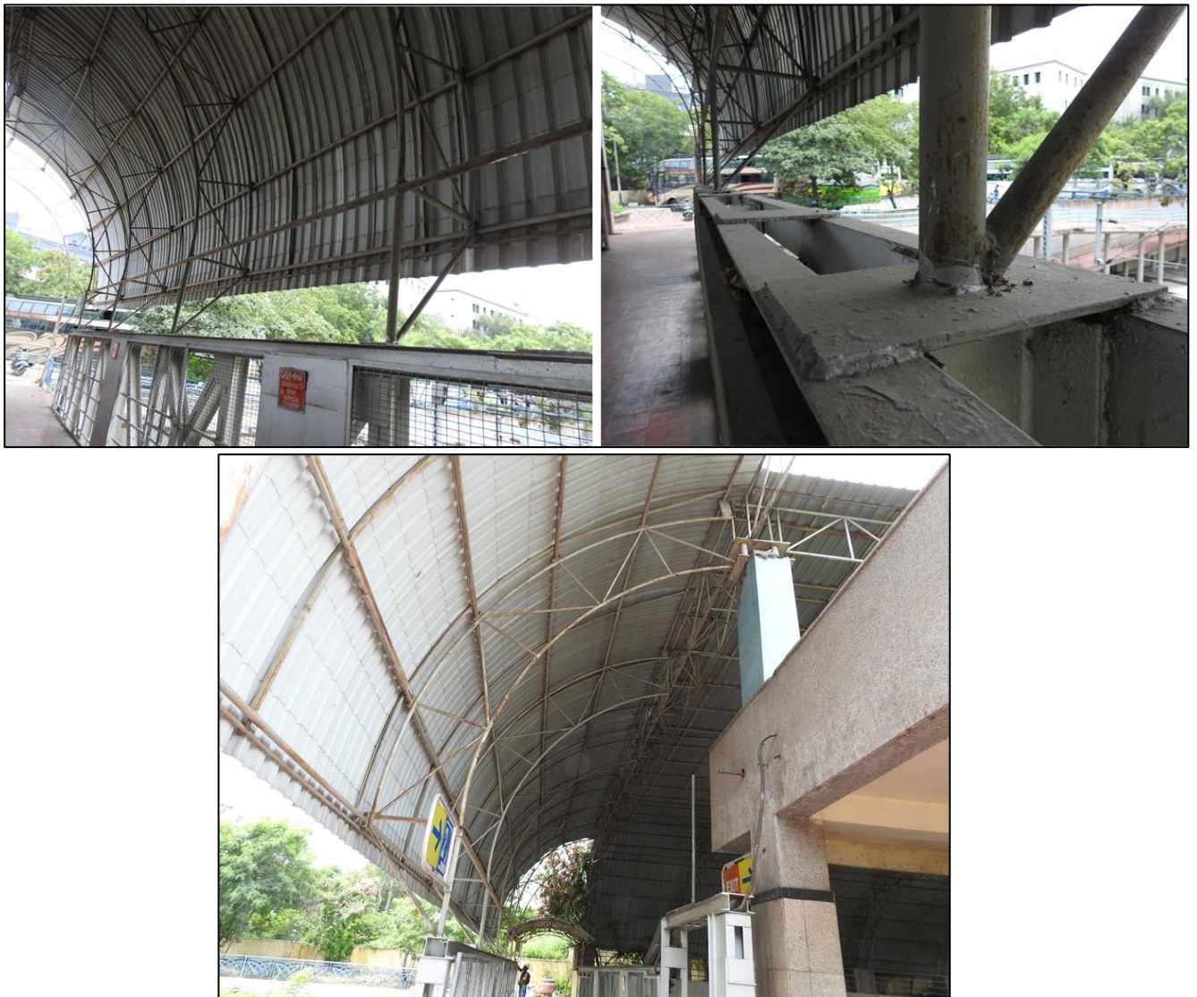
Fig 1.2: Roof Sheet and Roof truss
