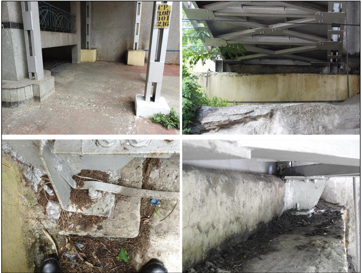
Fig 1.3: Trestles and their protection with concrete encasement
