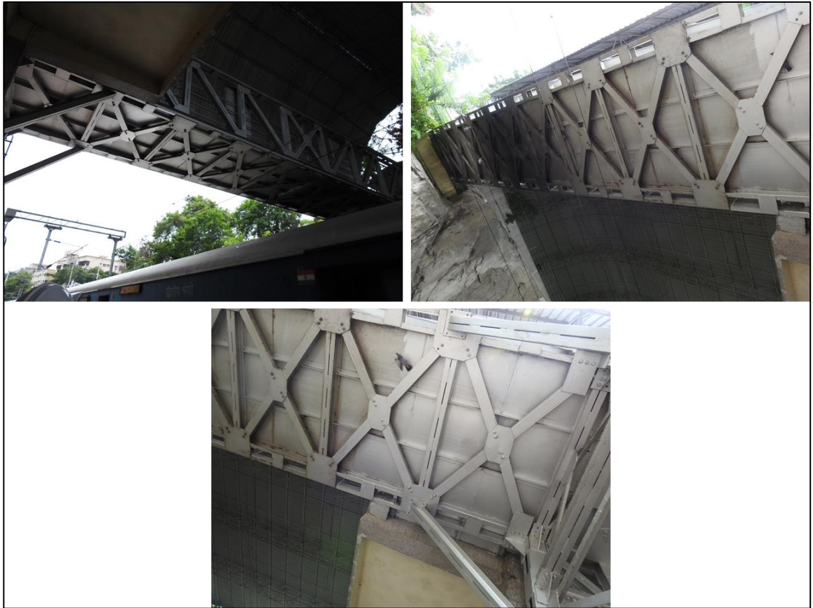
Fig 1.5: Slab is supported with sacrificial plate
