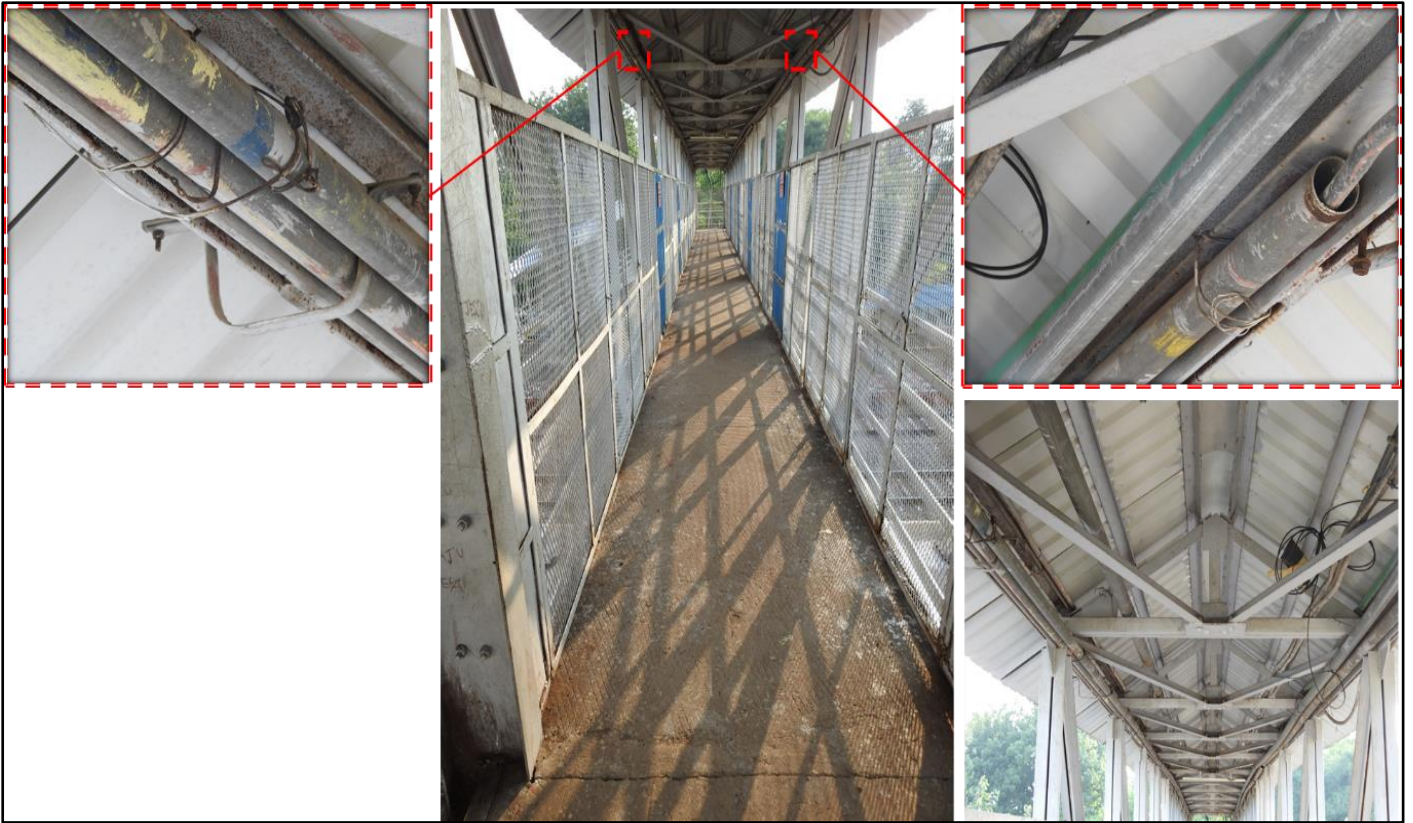
Fig 1.1: Cables, Roof truss, Flooring and Protective screen
