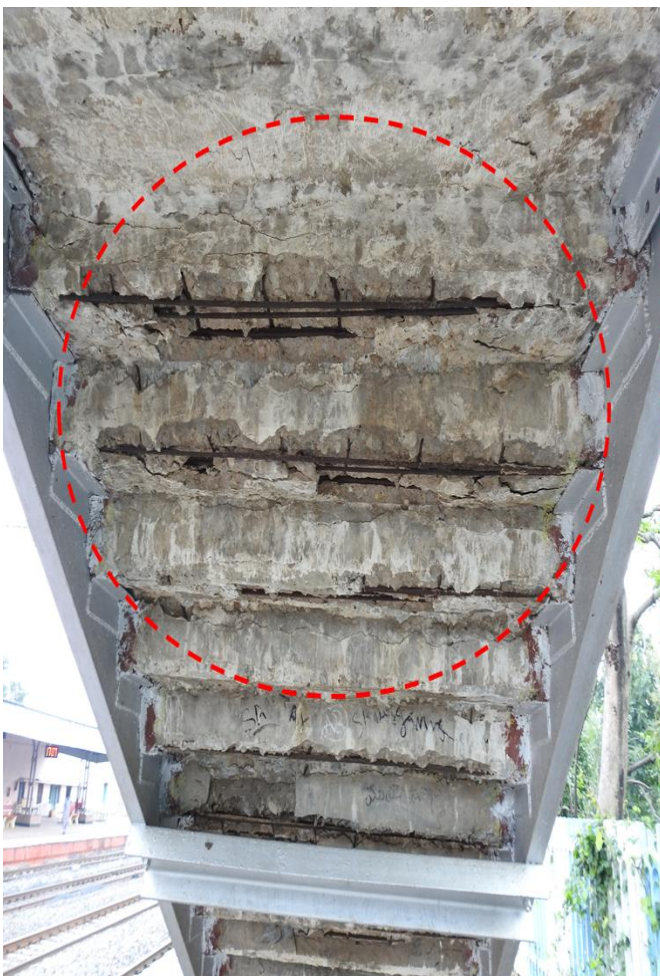
Fig: 2.4 spalling at Staircase 2 flight
