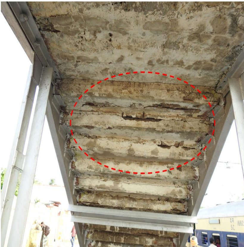
Fig: 2.3 spalling at Staircase 1 flight
