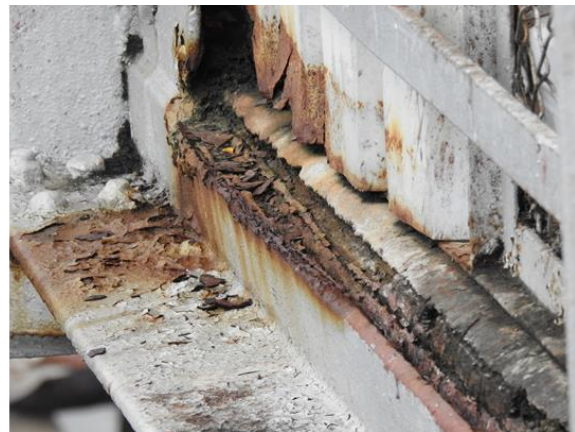
Fig 2.3: Bottom chord members are severely corroded along steel concrete joint
