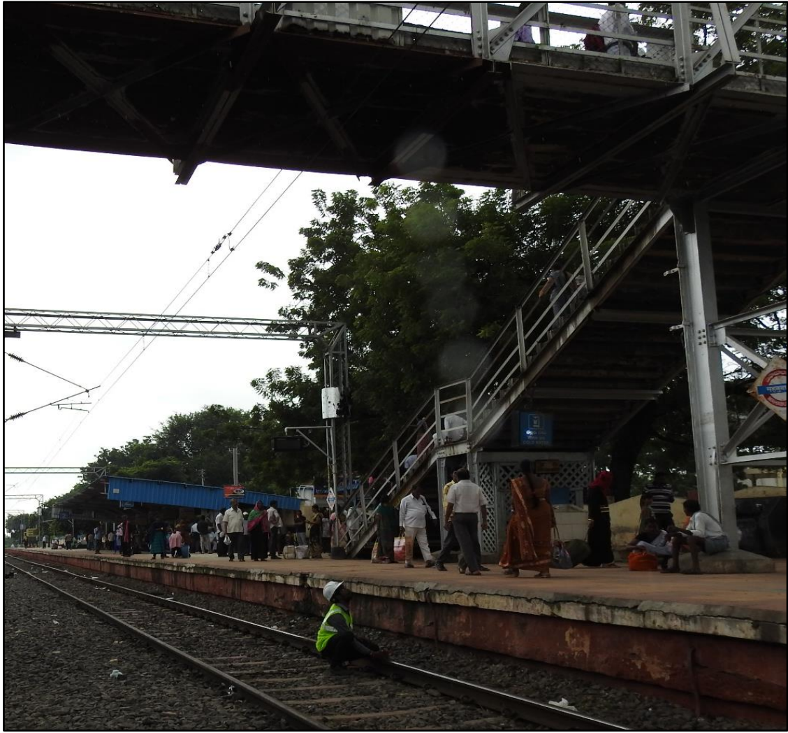
Fig 1.4: Measuring Vertical Clearance using laser meter (from rail top to girder bottom)
