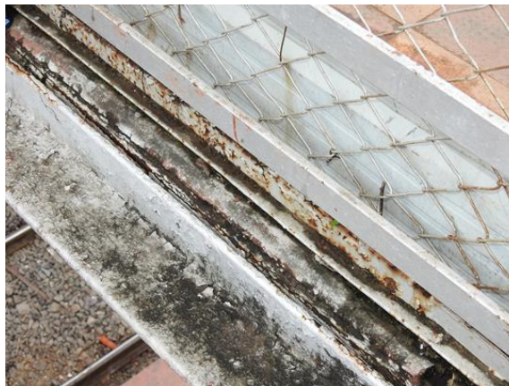
Fig 2.3: Bottom chord members are severely corroded along steel concrete joint
