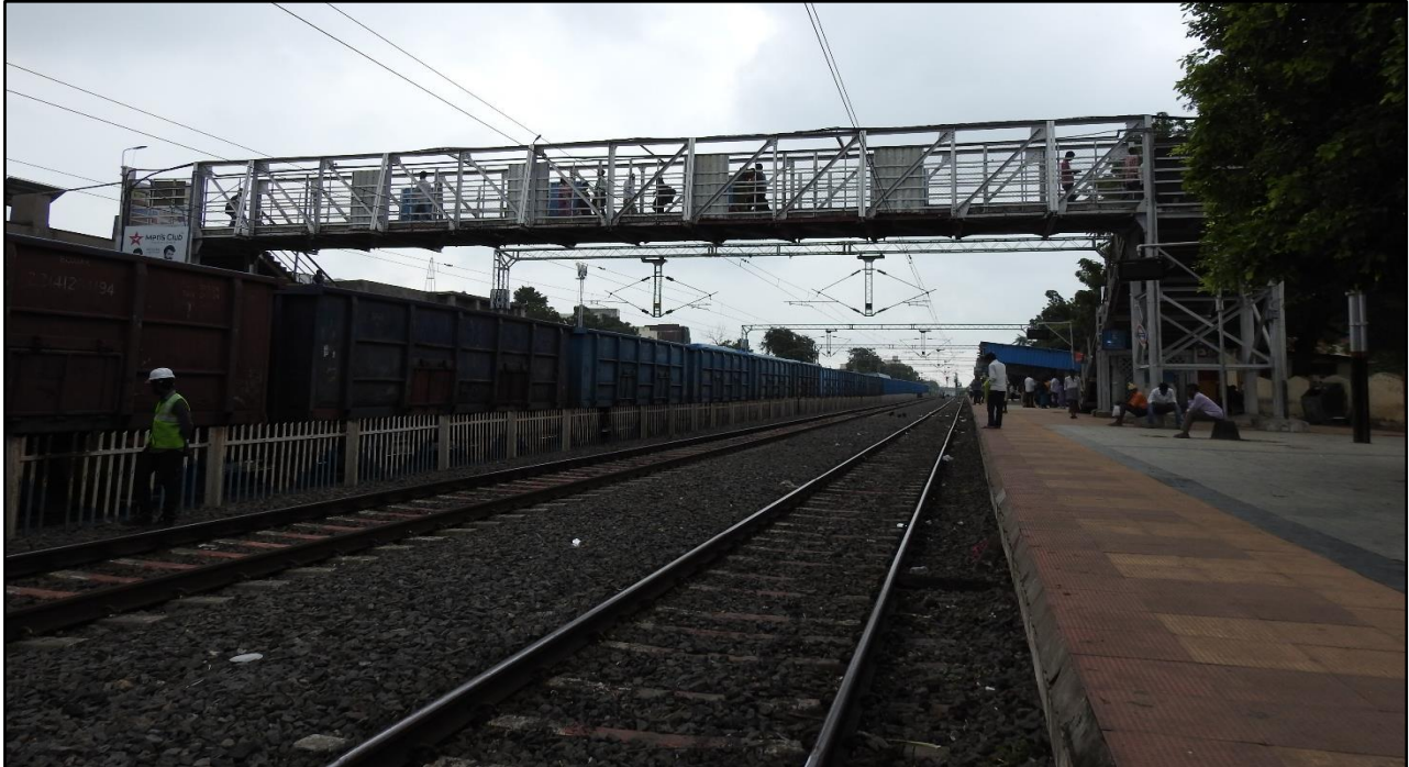
Fig 1.1: Front view of FOB towards Khammam Junction
