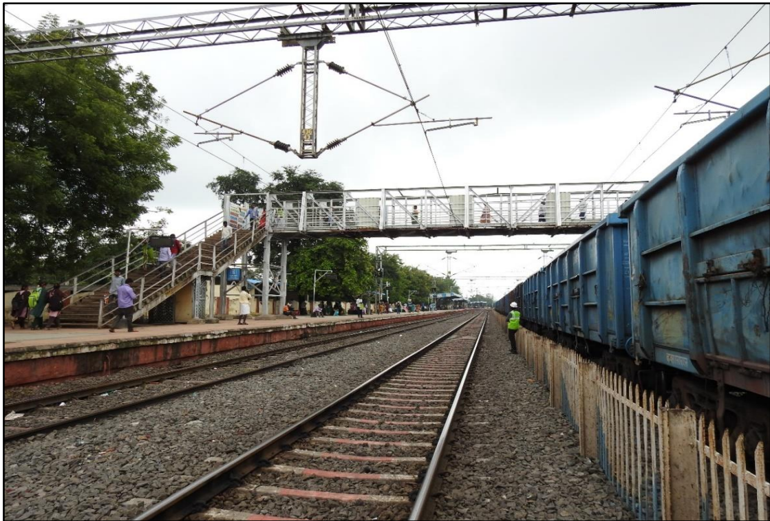
Fig 1.5: FOB view from platform 2 with staircase
