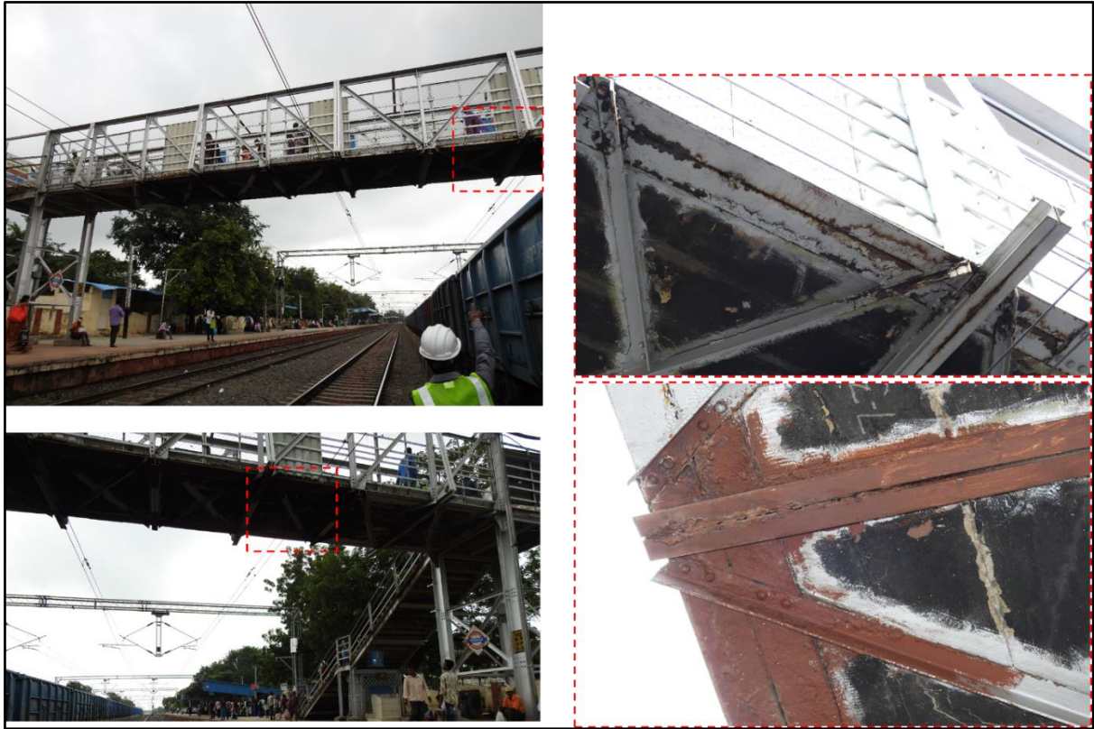
Fig 1.6: Red oxide has been applied at corroded joints and member
