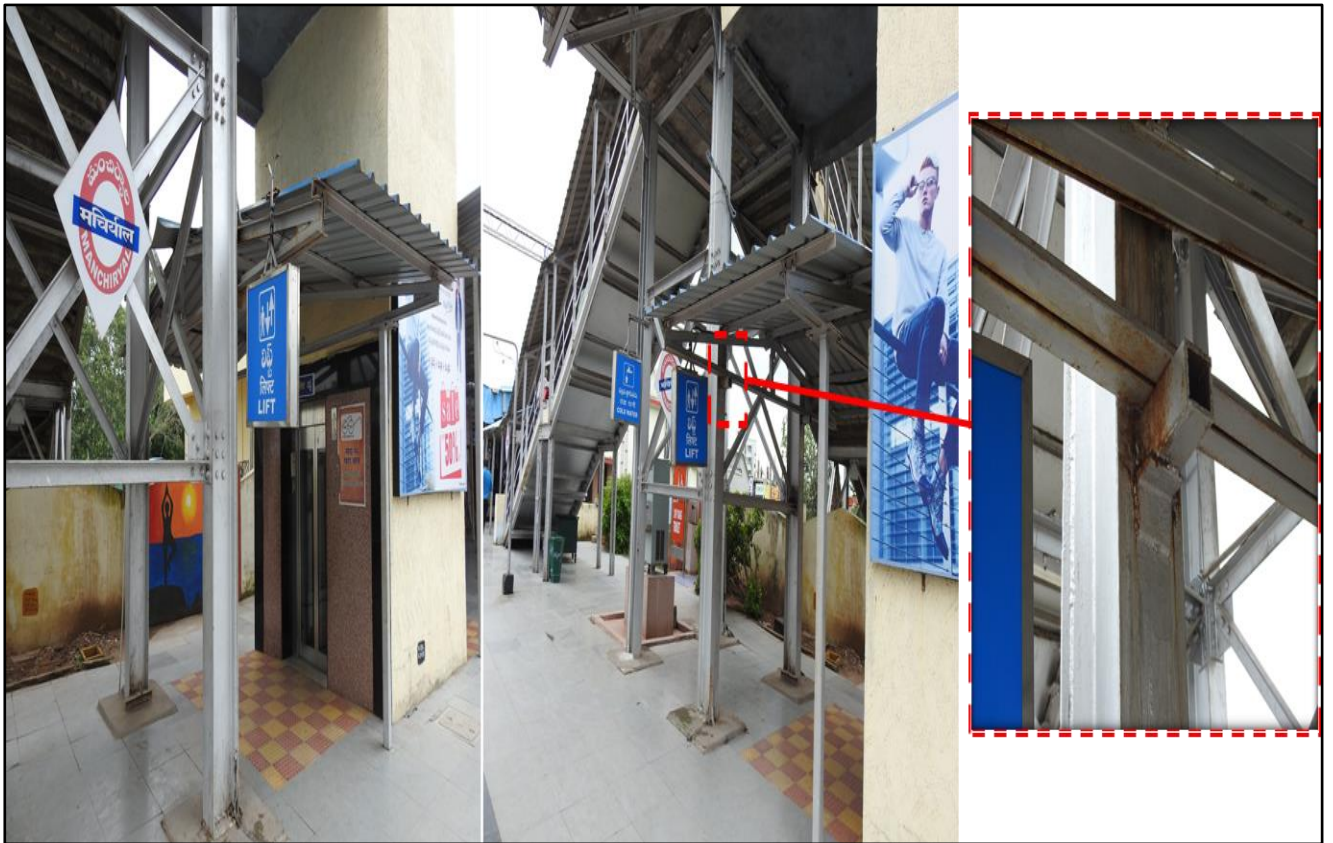
Fig 1.3: Elevator Roof truss supported on trestles on PF-1 and PF-2
