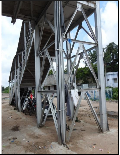
(f) 2 nd span Circulating area
