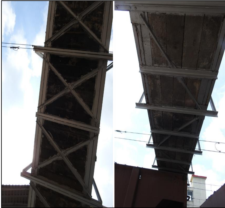
Fig 1.5: Bottom view of 1 st and 2 nd span of FOB
