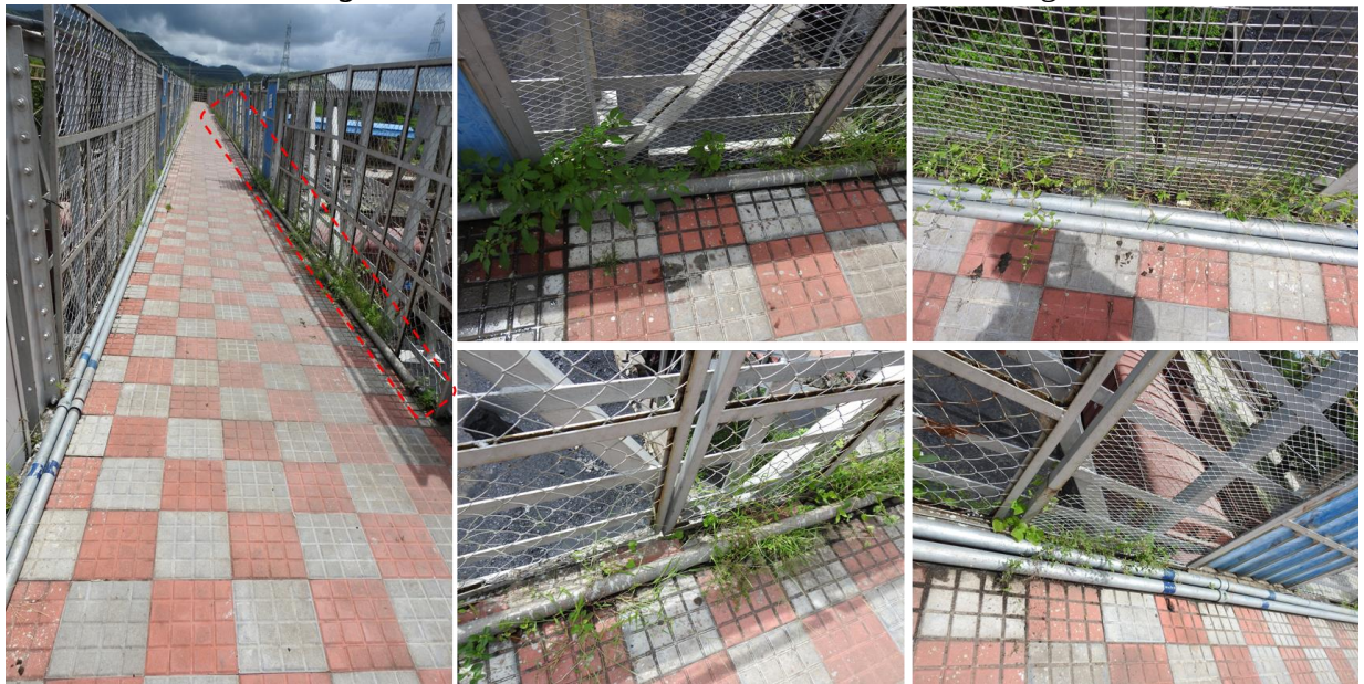
Fig 2.18: vegetation is observed on pathway of gangway
