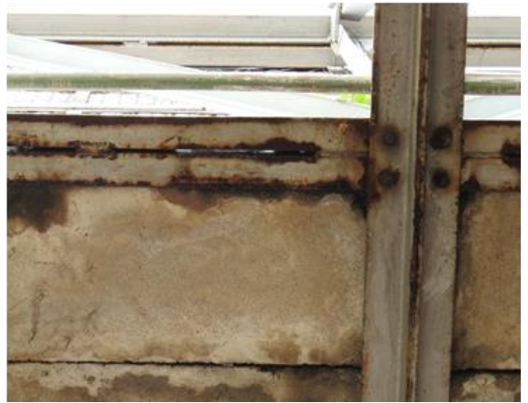
Fig 2.7: Some locations of Missing bolts and nuts in span 2
