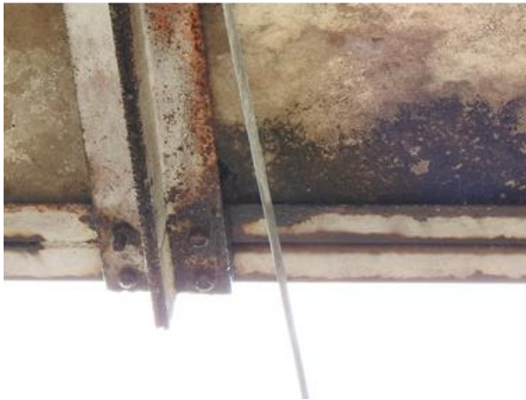
Fig 2.7: Some locations of Missing bolts and nuts in span 2
