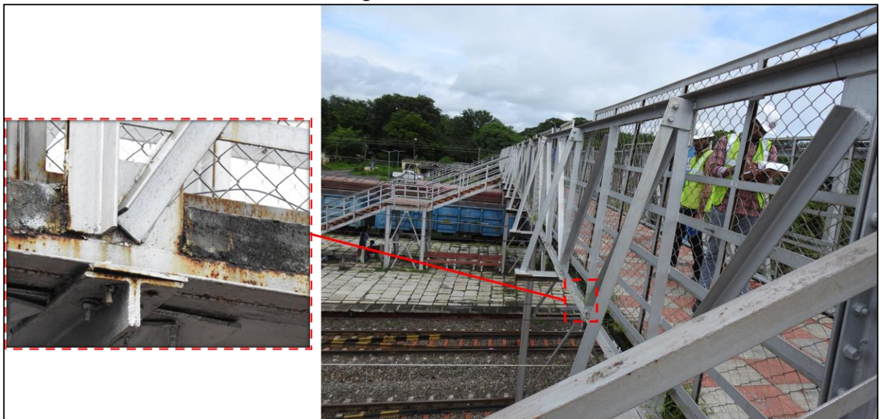
Fig 1.3: Main chord members, Floor beams, vertical and diagonal bracings
