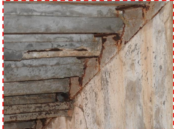
Fig 2.4: Spalling and cracking is observed in repaired panels of staircase 2
