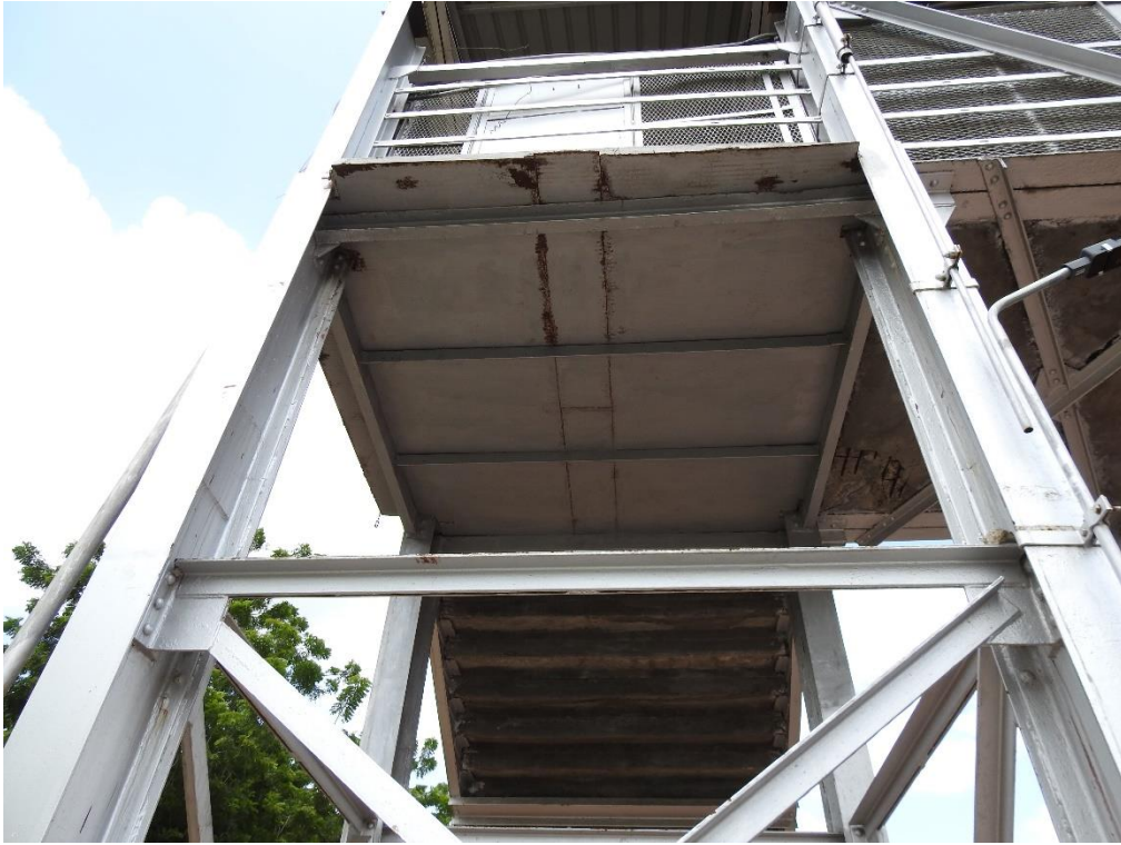
Fig1.9: Pathway on trestles on platform 2, under the staircase there is room, which is of debris.
