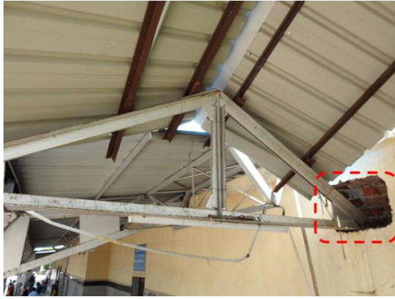
Fig 1.2: Staircase Roof truss on platform-1 one end is supported on Masonry wall
