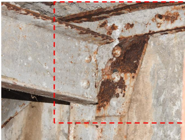
Fig 2.5: Locations of Deteriorations in staircase first flight from bottom
