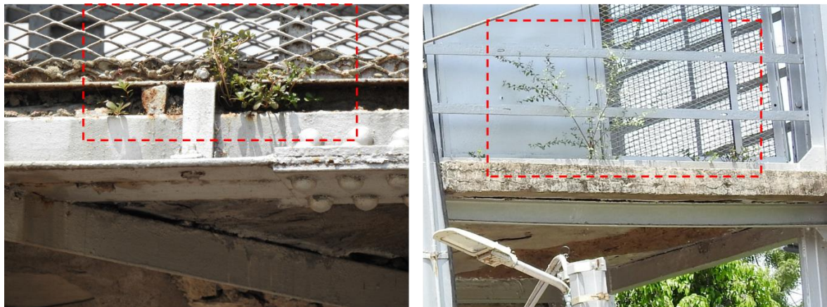
Fig 2.1: Locations of Vegetation growth and debris
