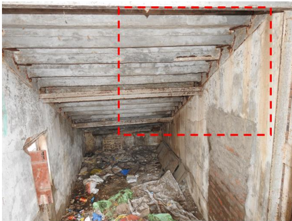
Fig 2.4: Spalling and cracking is observed in repaired panels of staircase 2
