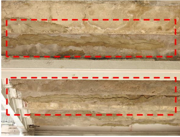
Fig 2.4: Spalling and cracking is observed in repaired panels of staircase 2
