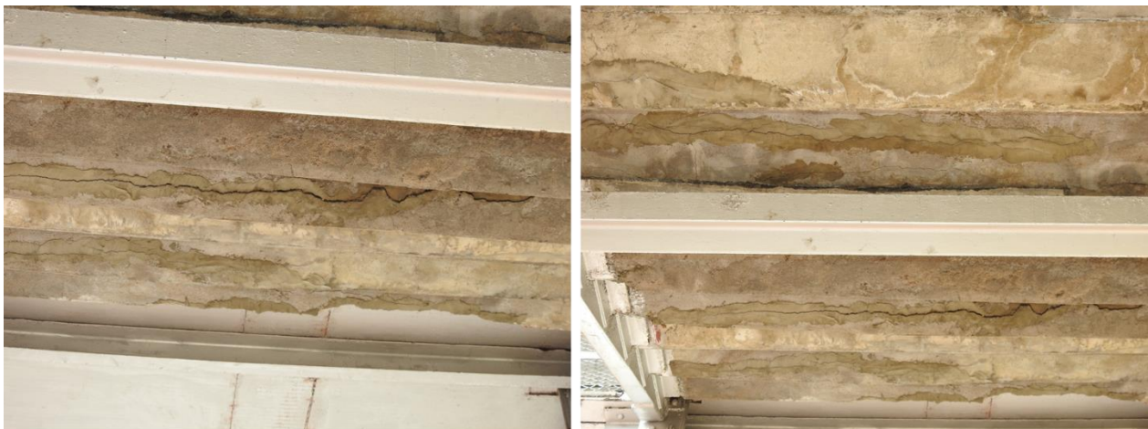
Fig 1.7: Spalling is observed in Floor slab from bottom
