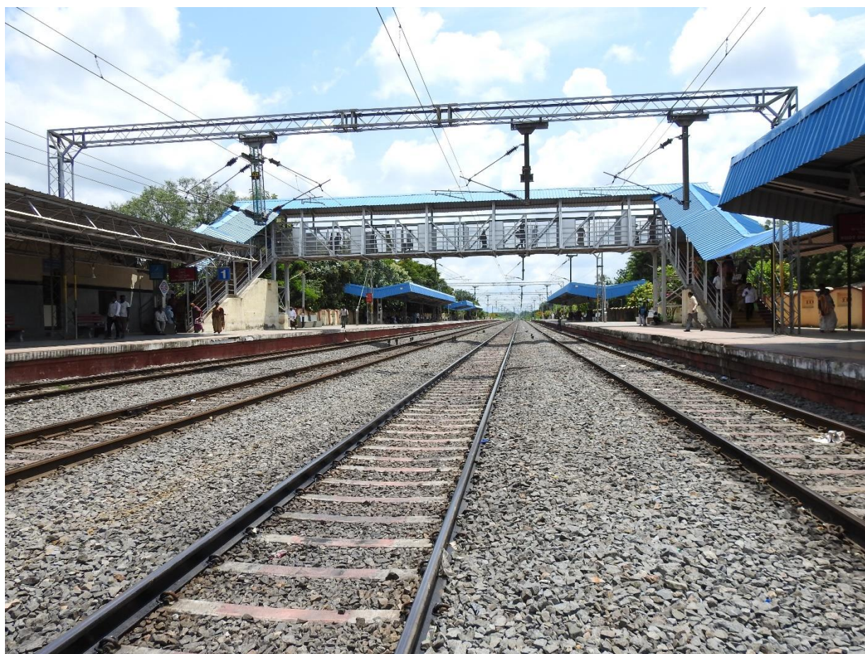
Fig 1.1: Front view of FOB towards Vijayawada Junction
