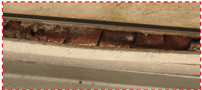
Fig 1.6: Bricks are used to fill the gap above floor beam
