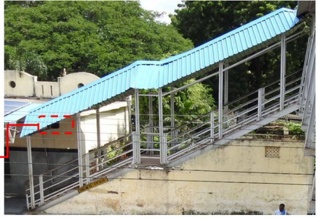
Fig 1.2: Staircase Roof truss on platform-1 one end is supported on Masonry wall
