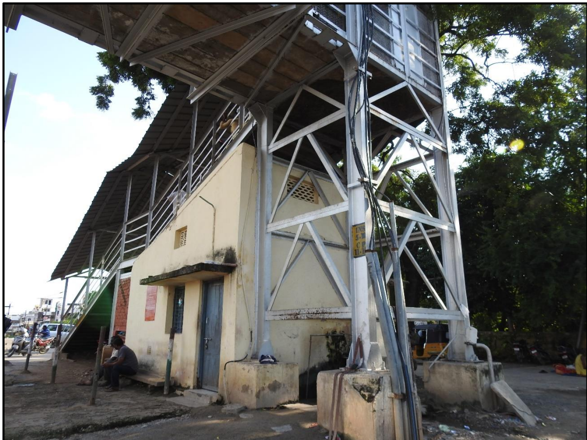
Fig 1.10: Trestles supporting staircase
