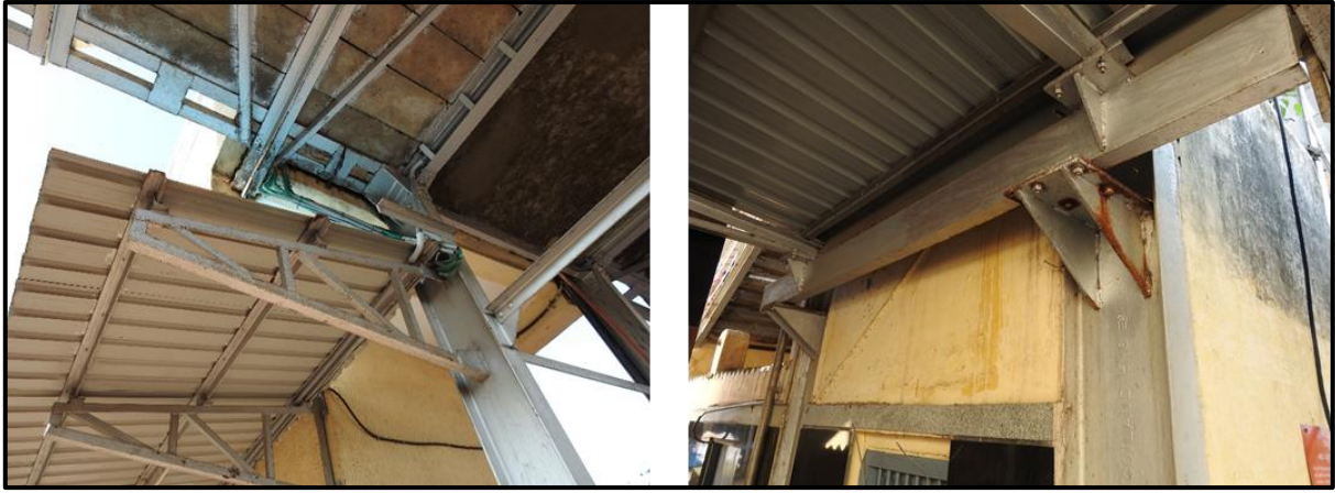
Fig 1.8: shed above lift is supported to Trestles
