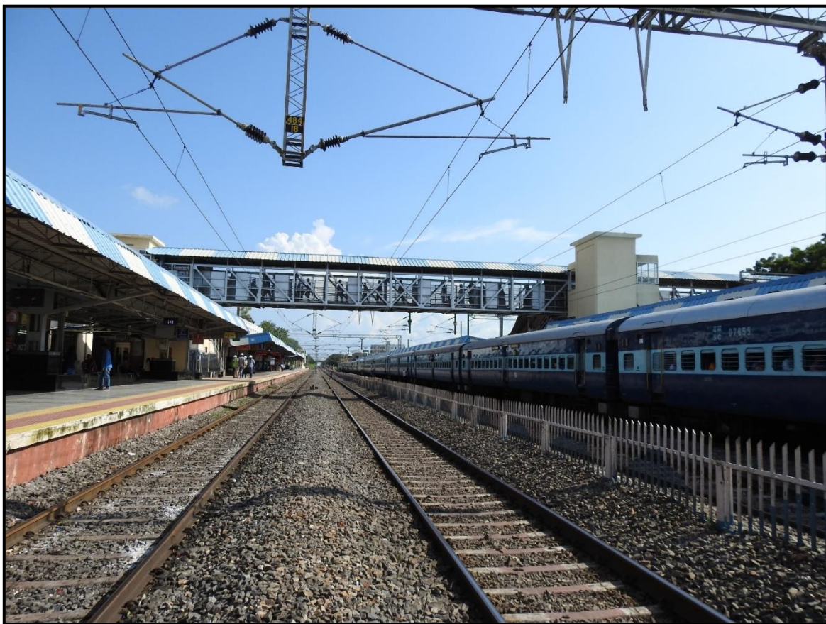
Fig 1.1: Front view of FOB span 1 towards Madira
