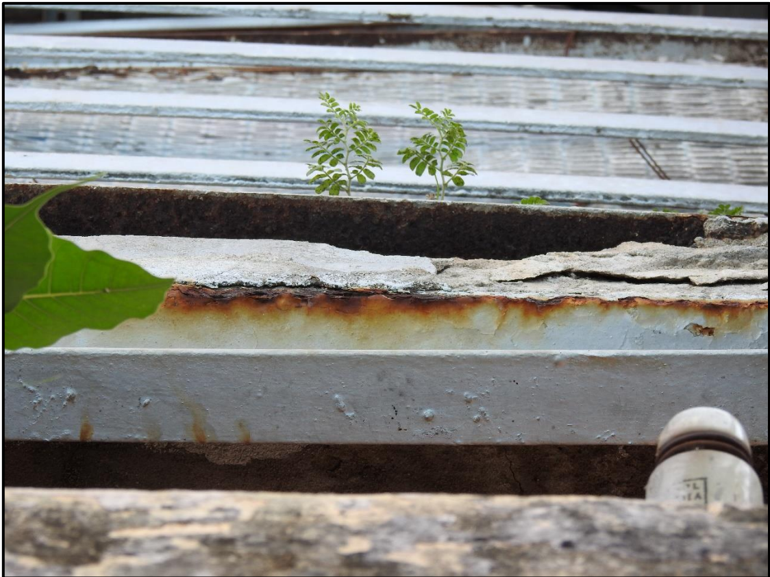
Fig 1.7: Vegetation is observed along the length of FOB
