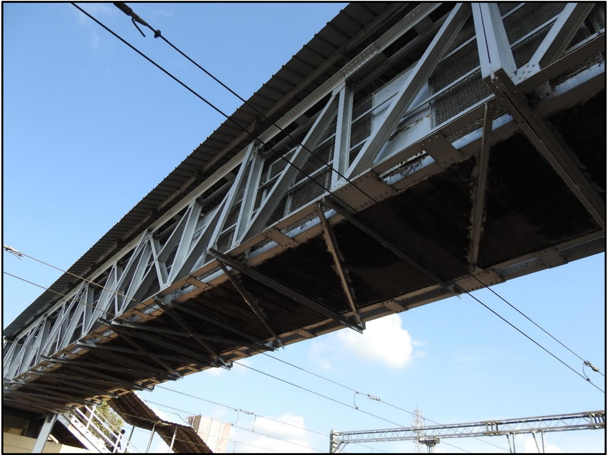
Fig 1.11: Span 1 bottom view
