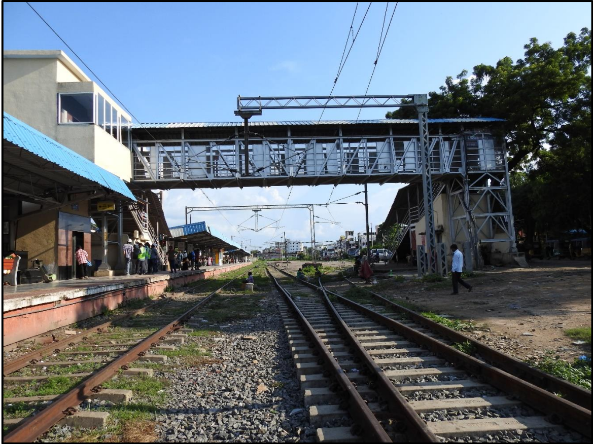
Fig 1.2: Front view of FOB span 2 towards Madira
