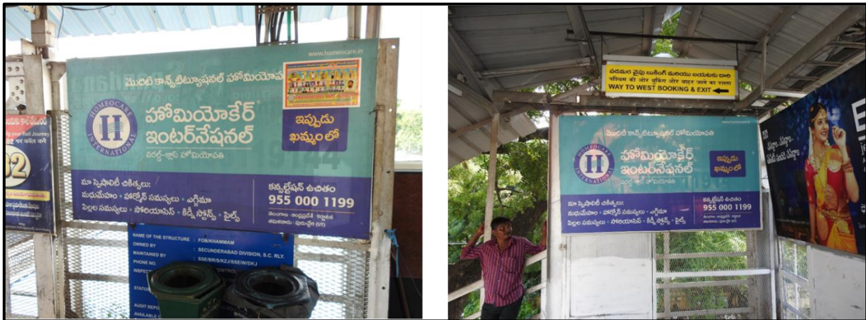
Fig 1.9: Advertisement boards are supported to passenger protection
