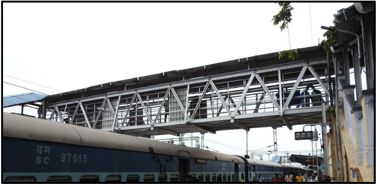
Fig 1.1: Front view of FOB towards Secunderabad Junction
