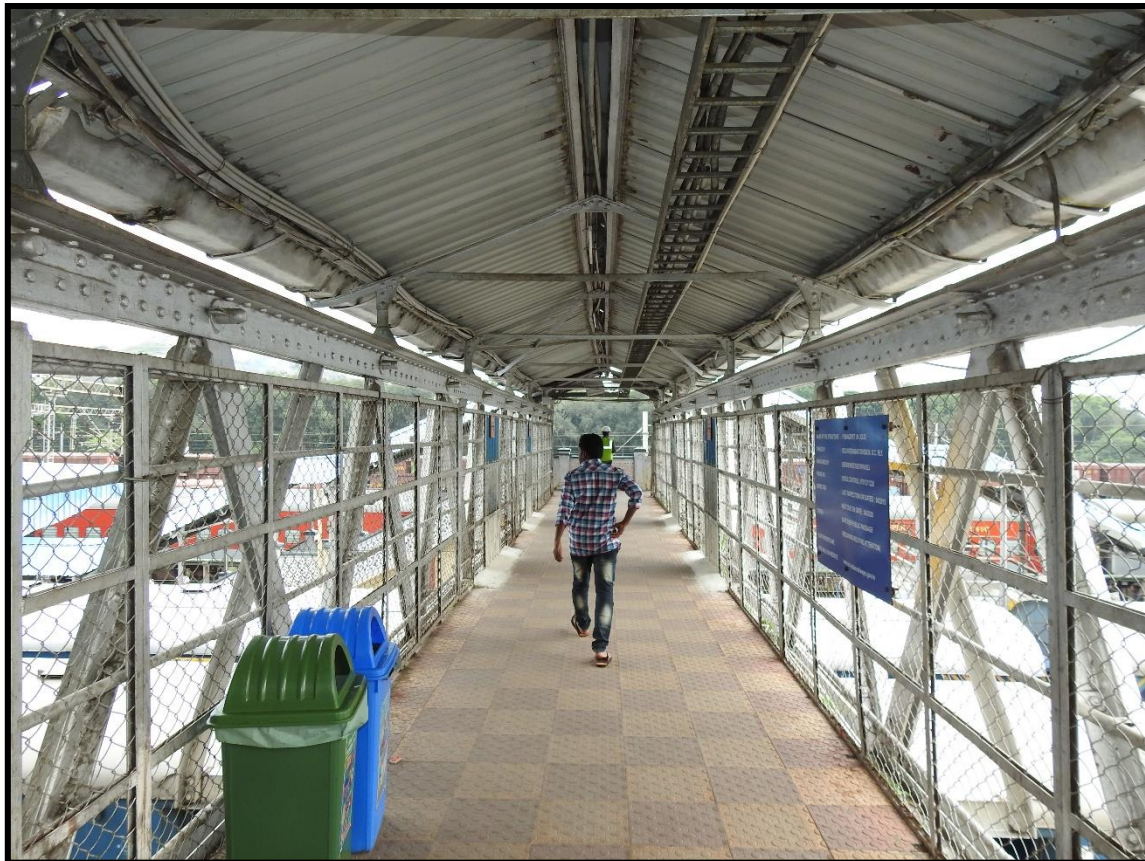
Fig 1.2: Set of cables running along the length of FOB
