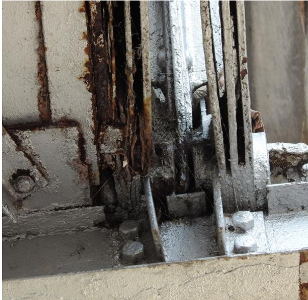
Fig 2.5: Locations of Severe corrosion on deck from bottom
