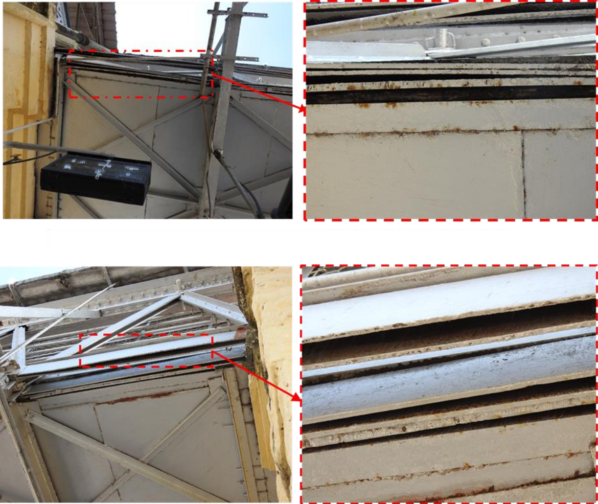
Fig 1.7: Bending of bottom main plates
