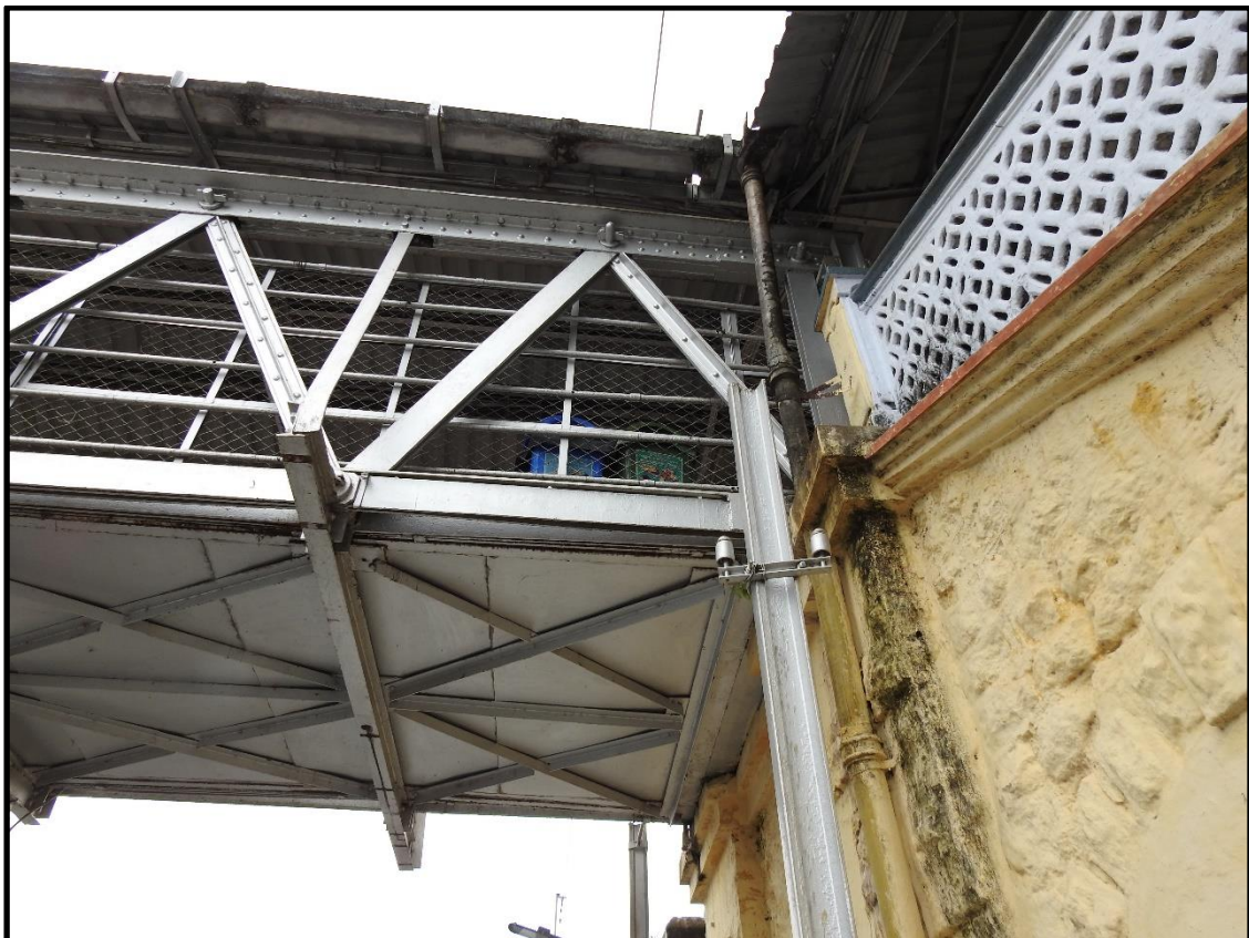
Fig 1.10: Bottom view of FOB near platform 1
