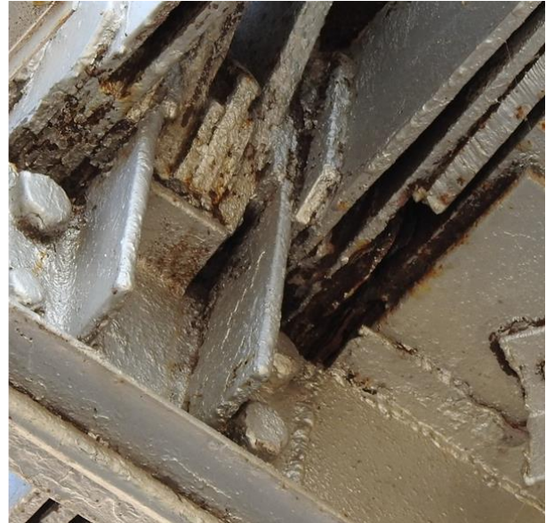
Fig 2.5: Locations of Severe corrosion on deck from bottom
