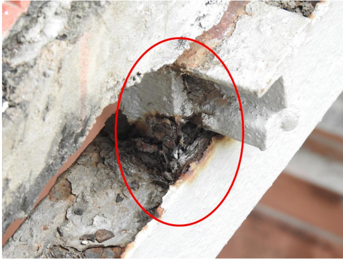
Fig 2.7: Corrosion at joints
