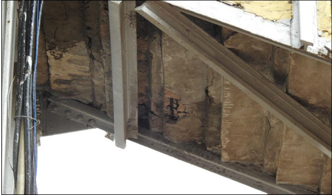
Fig 1.8: Patch work is observed at PF-2 stair case flight slab panels
