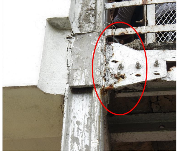
Fig 2.7: Corrosion at joints
