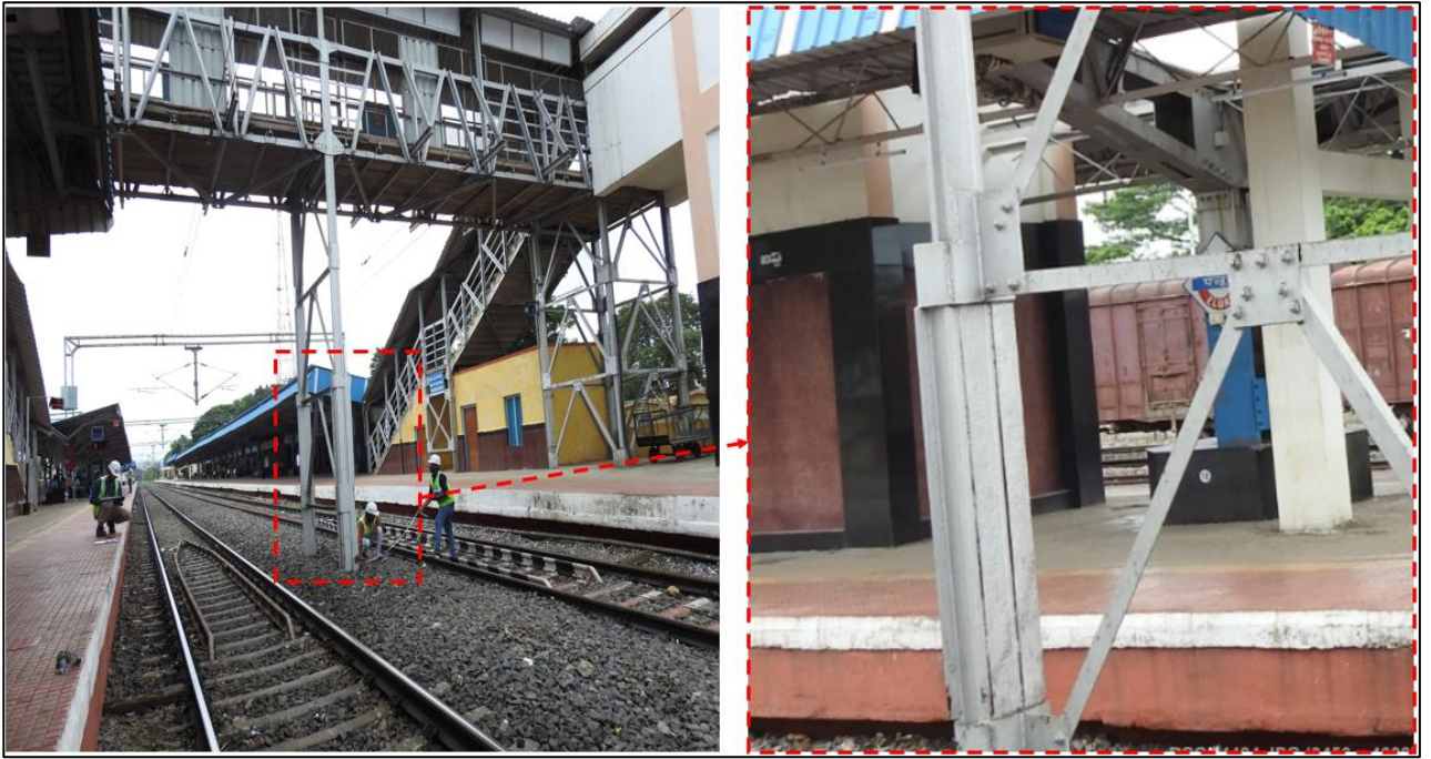
Fig 1.4: Stanchion Rail sections details
