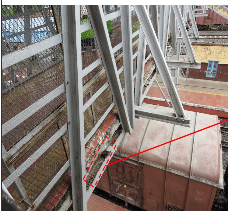
(c) Corrosion at Bottom chord
