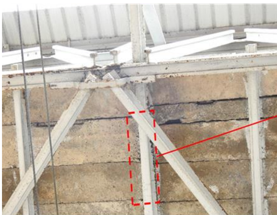
Fig 2.4: Corrosion of floor beams
