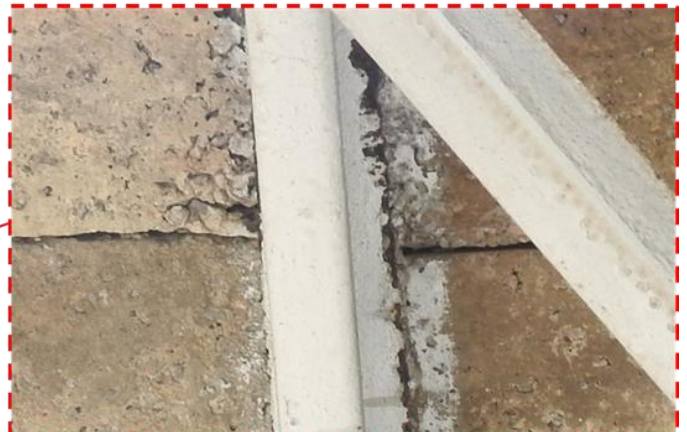
Fig 2.4: Corrosion of floor beams
