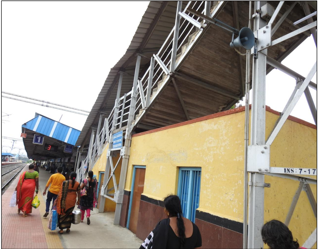
Fig 1.6: Under staircase not inspected due to existing room
