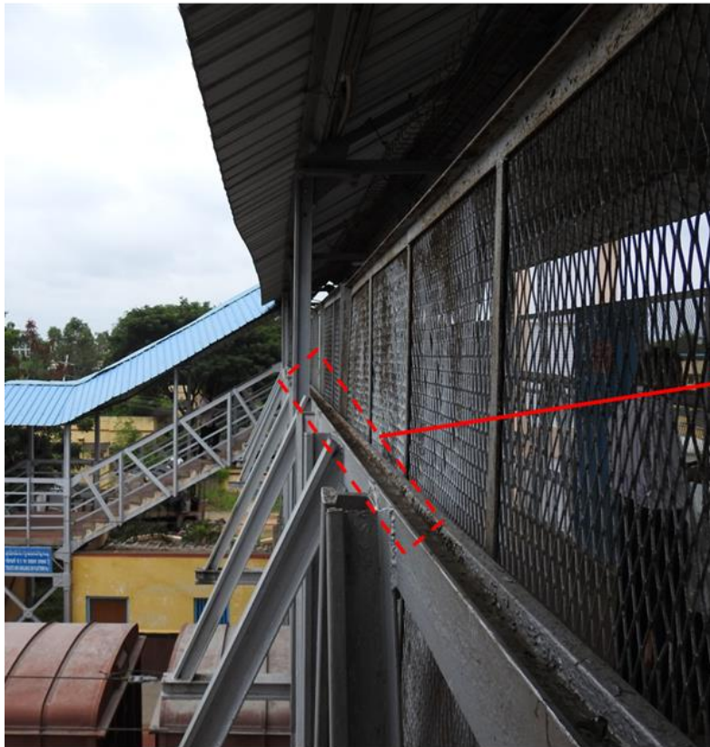
Fig 2.3: Corrosion of top chord member
