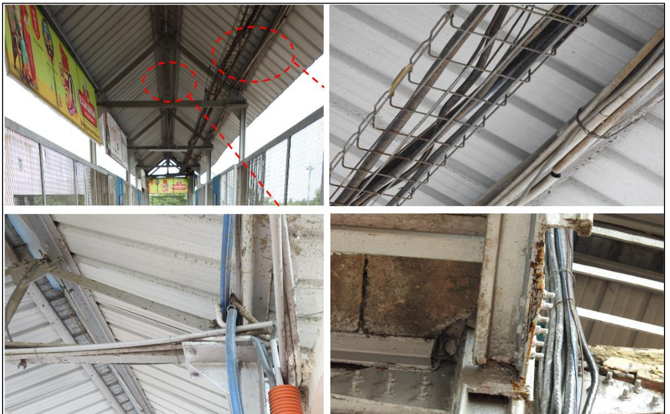
Fig 1.3: Additional loads of HDPE, PVC pipes
