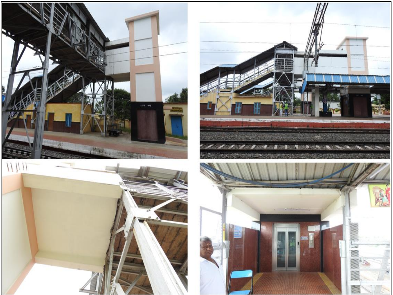
Fig 1.5: Lift is connected to staircase landing in both platforms
