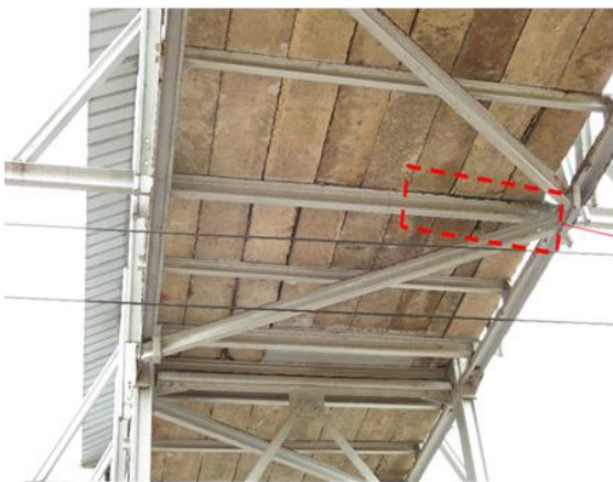
Fig 2.3: Corrosion of top chord member
