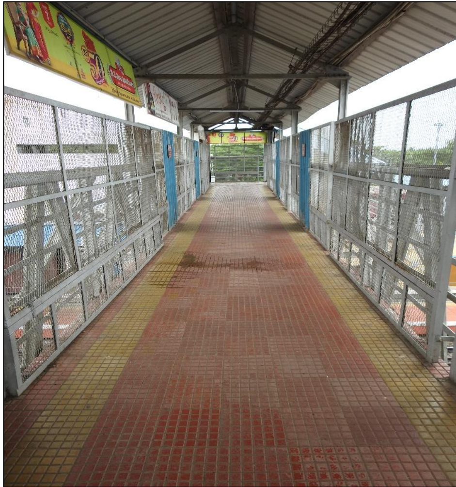
Fig 1.2: FOB span 1 & 2 pathway, Roof Truss, Chequered tiles, protective screen and Hoardings
