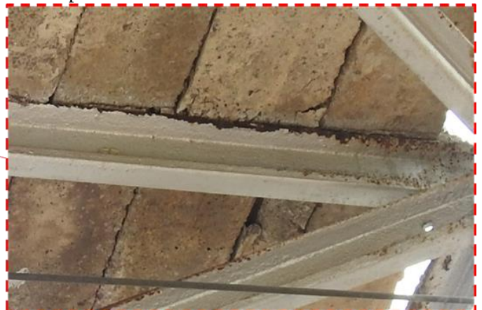
Fig 2.3: Corrosion of top chord member
