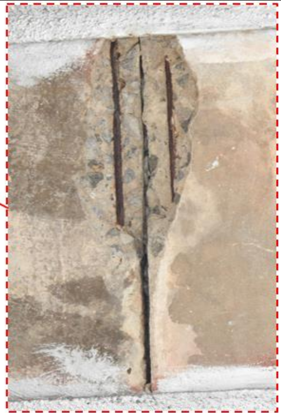
c) Reinforcement exposed on bottom of slab panels (Staircase 3 - Main landing)
