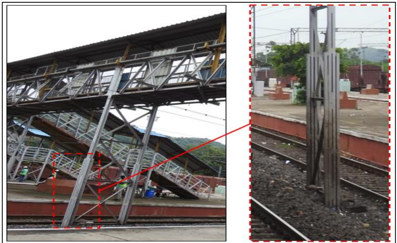
Fig 1.4: Stanchion column Rail sections details
