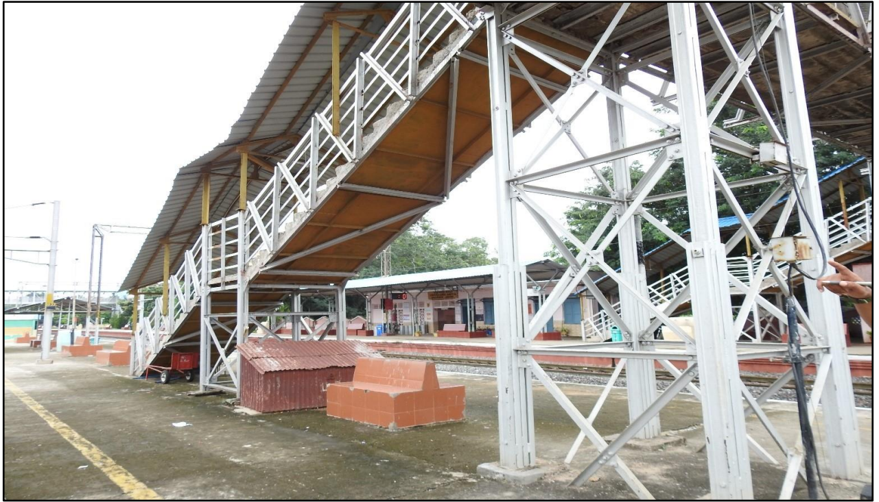
Fig 1.5: Staircase bottom view
