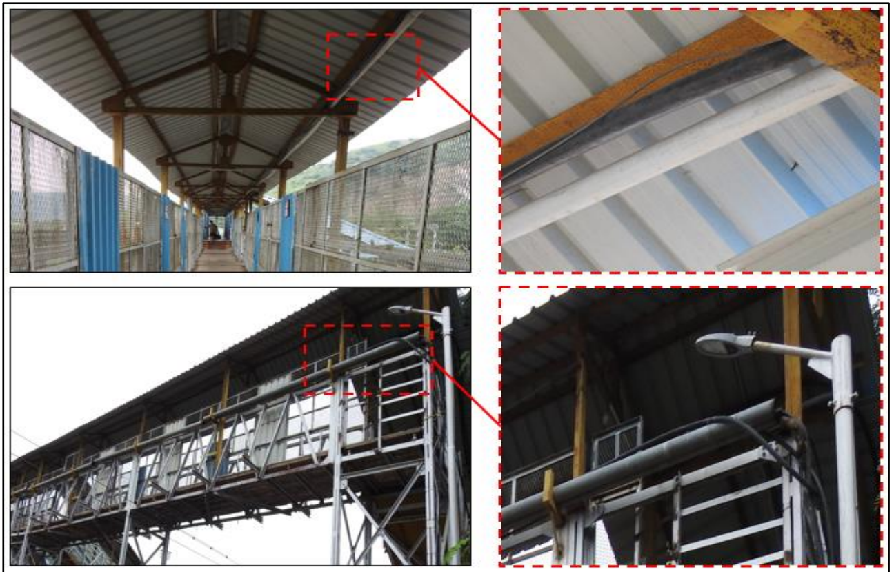
Fig 1.3: Additional loads of GI, HDPE, PVC pipes
