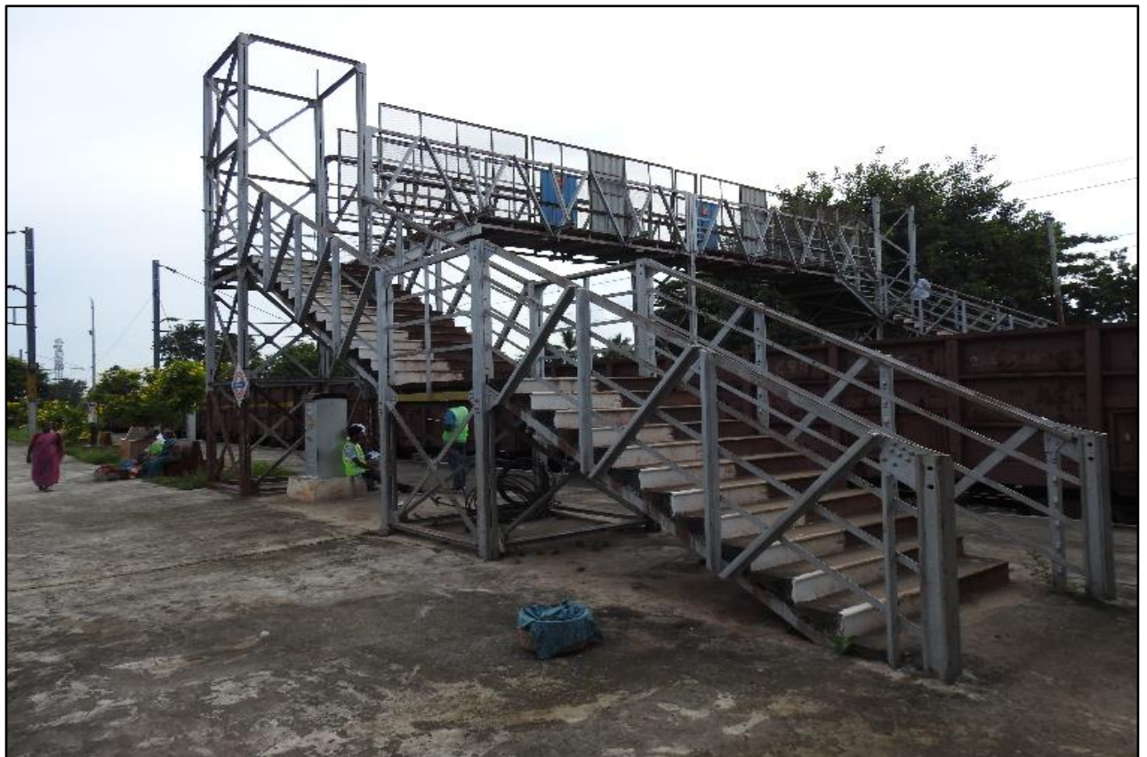
Fig: 1.8 Railing, Trestle of FOB
