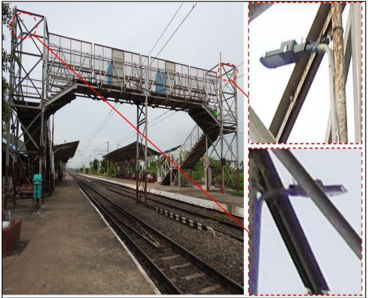
Fig 1.1: Light Post attached at Trestles 1 & 2
