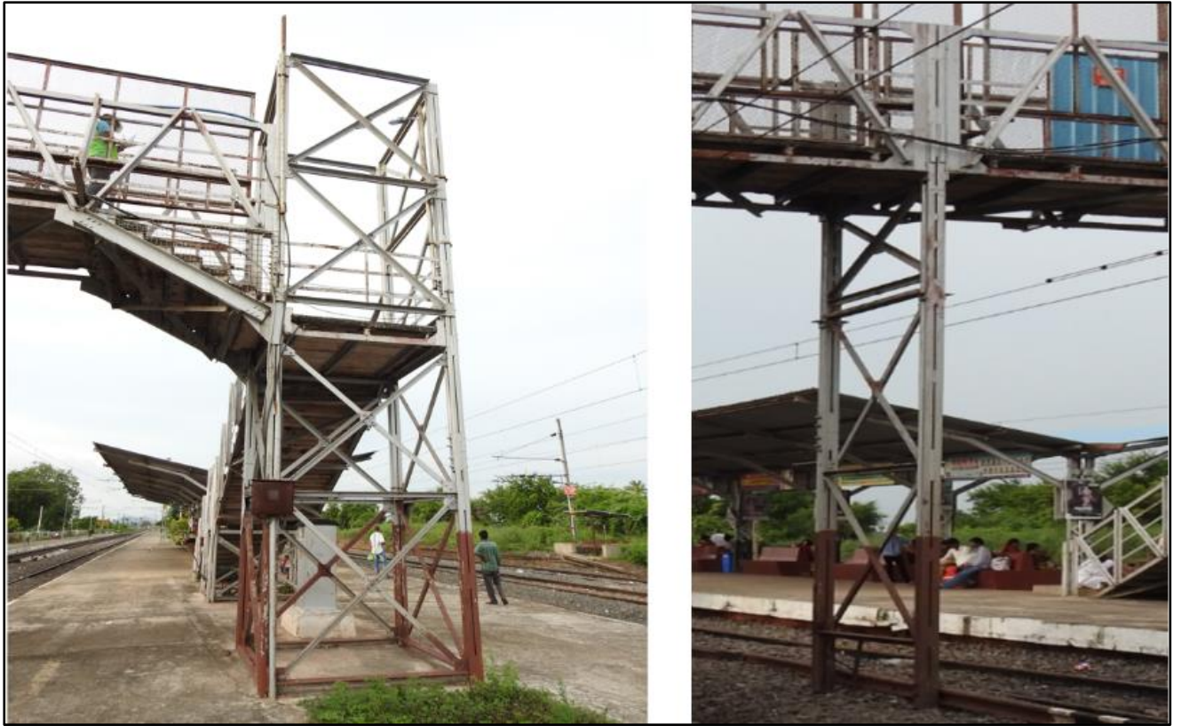
Fig 1.9: Trestle and Stanchion of FOB
