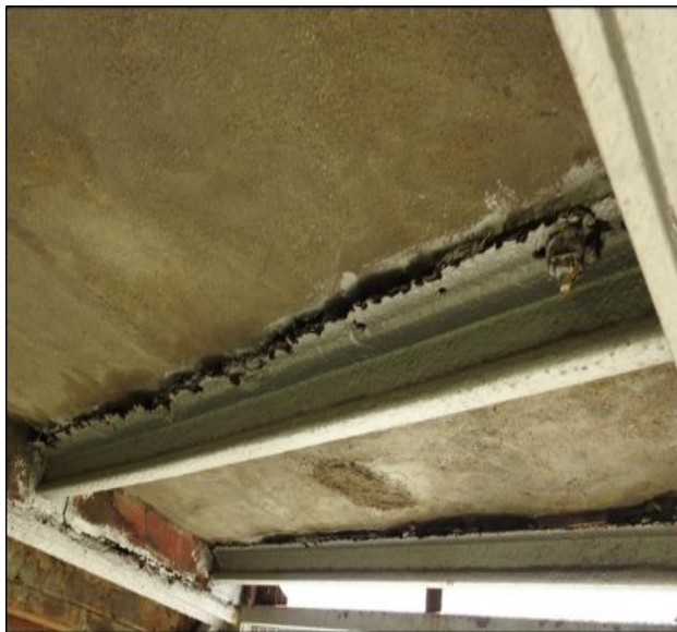
d) Corrosion of floor beam and Patch work observed at landing
