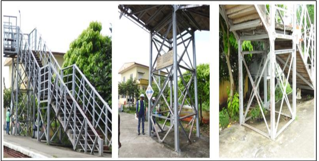
Fig 1.3: Staircase-1 Trestles details
