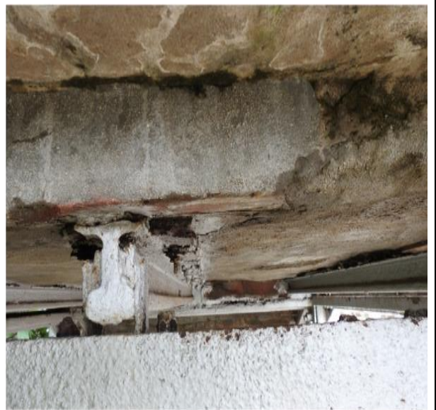
d) Corrosion of floor beam and Patch work observed at landing
