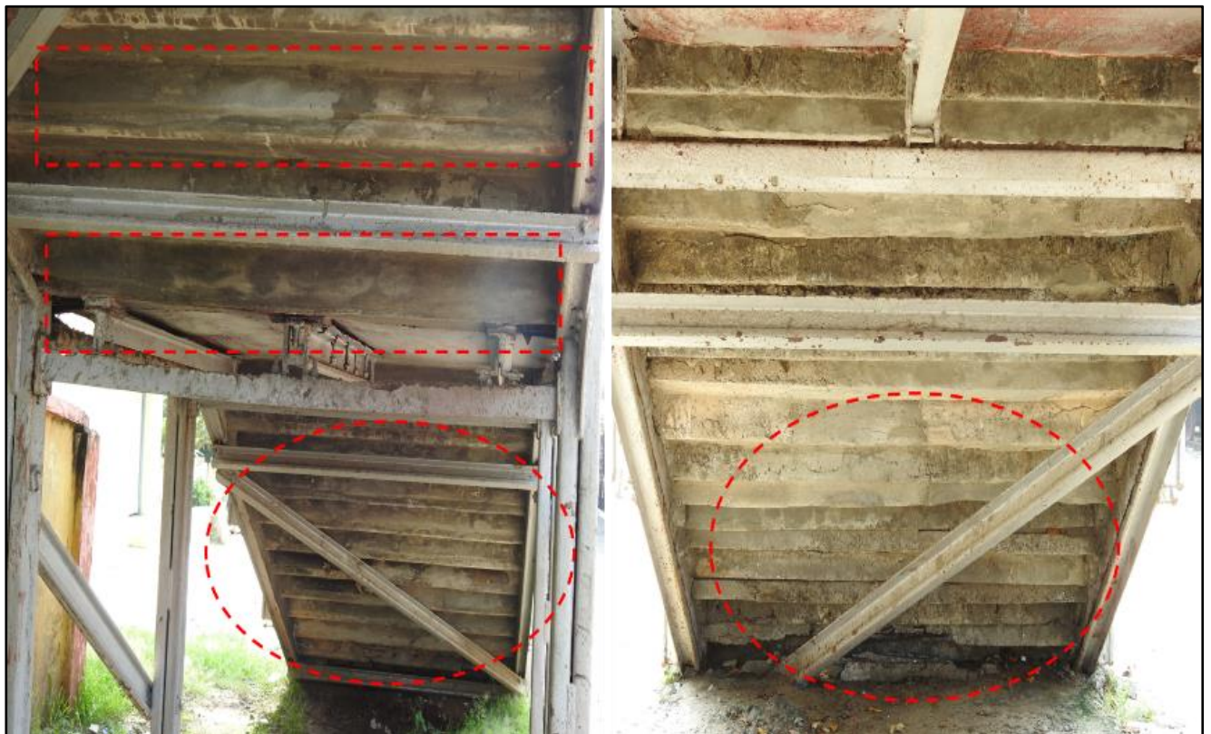
Fig 1.5: Patch work is observed at PF- 2 stair case flight slab panels
