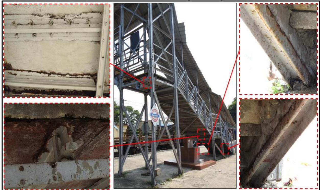
III. Corrosion observed at floor beams in landing and Stringer beams in Staircase 1
