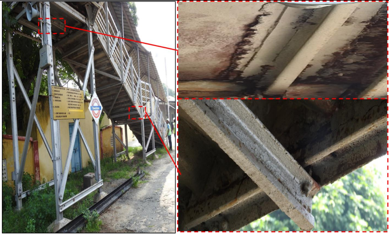
III. Corrosion observed at floor beams in landing and Stringer beams in Staircase 1
