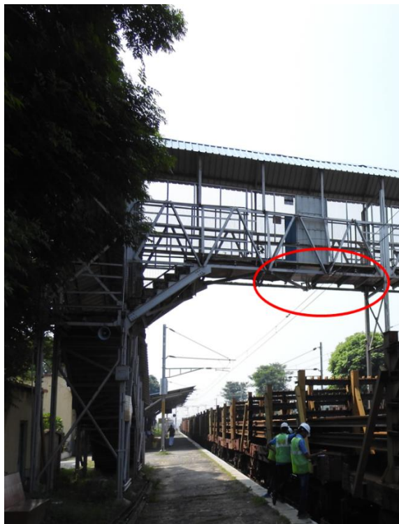
Fig 2.2: Corrosion of floor beams of span-1
