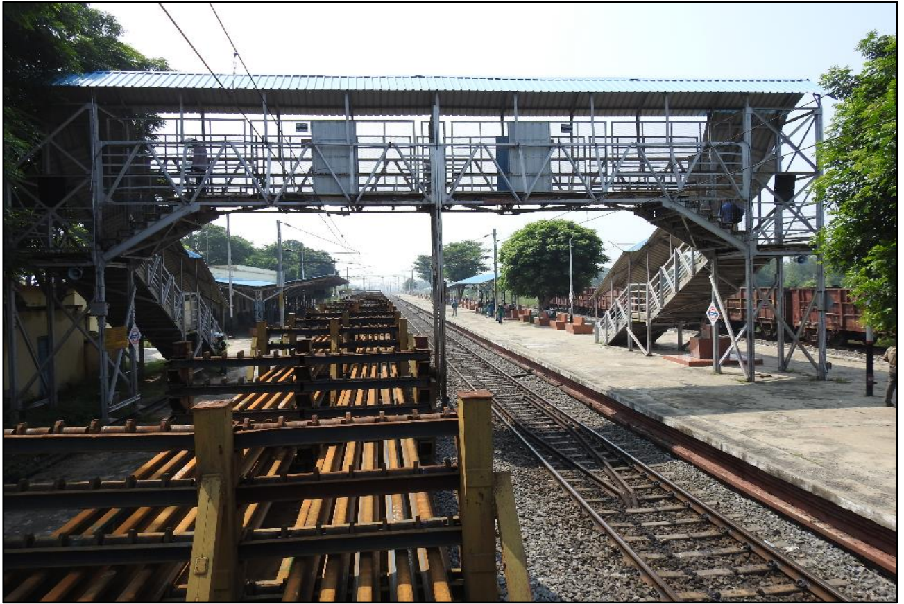
Fig 1.1(a): Front view of FOB span 1 &2
