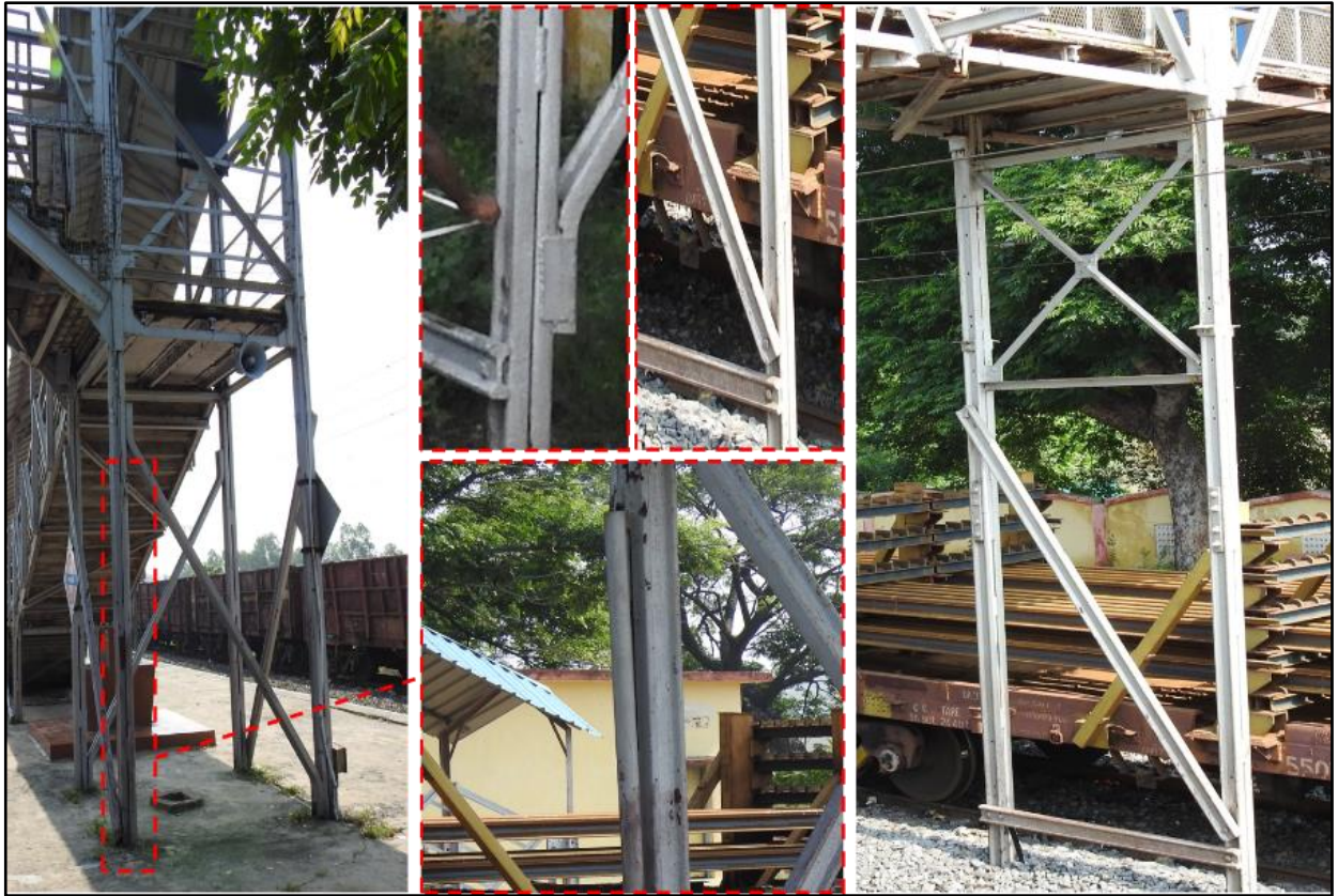
Fig 1.4: Trestles, Stanchion column Rail sections details and Additional GI pipe supported
