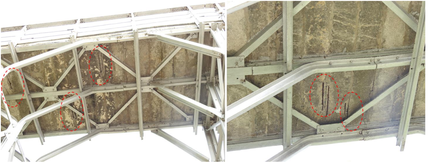
Fig 2.20: Exposed reinforced Pre-cast slab panels
