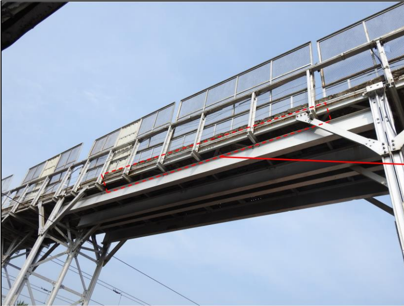
f) Corrosion observed in bottom chord
