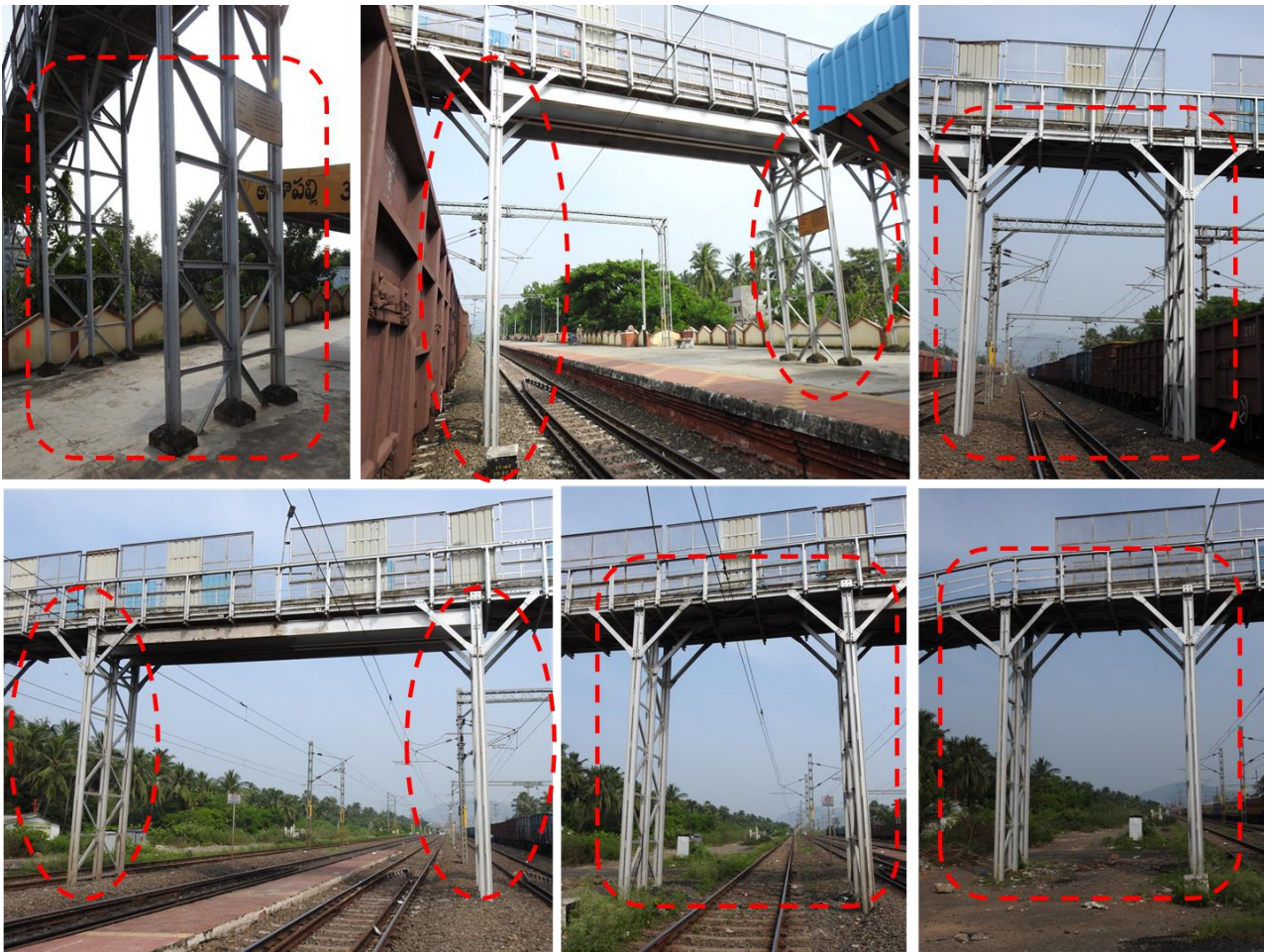
Fig 1.3: Stanchion column sections details
