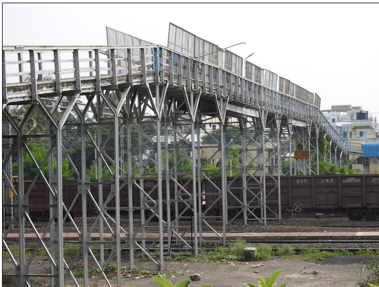
Fig 1.1: View of FOB and Ramps on both sides
