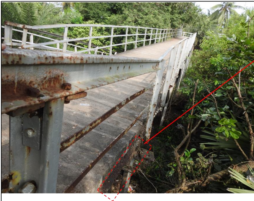
g) Corrosion of ramp landing beam
