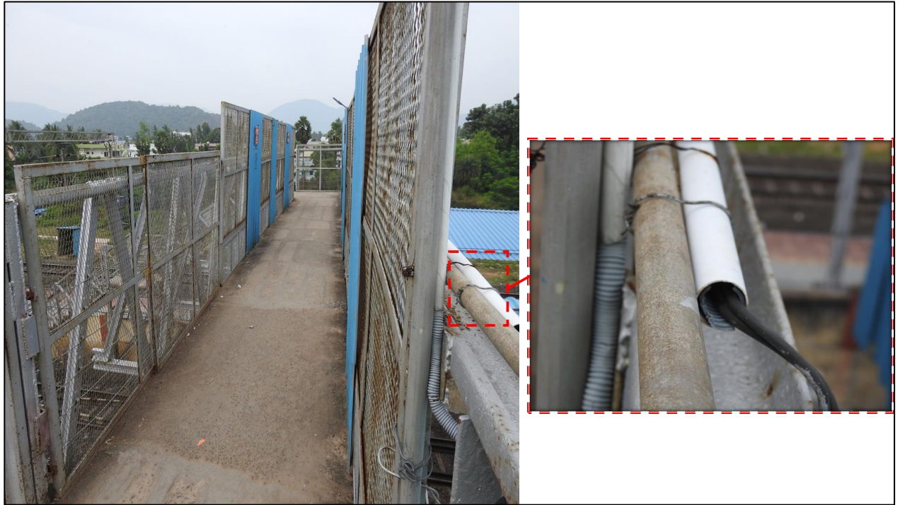
Fig 1.2: FOB pathway, protective screen and Additional loads of PVC pipes
