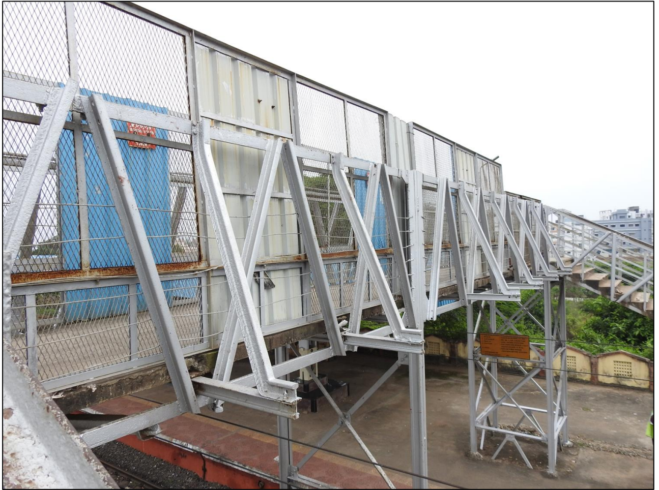
Fig 1.4: Arrangement of truss
