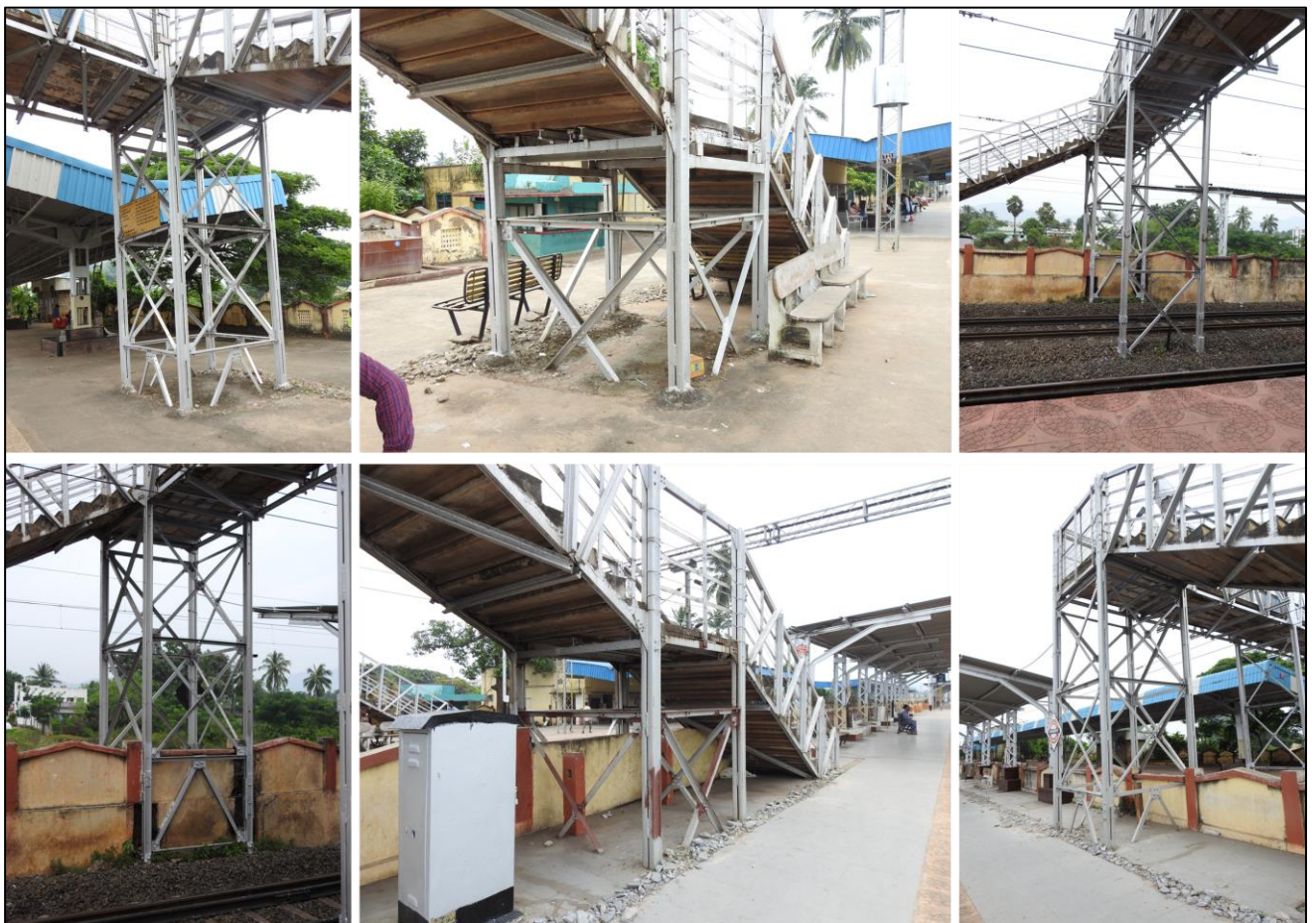
Fig 1.3: Trestles and Stanchion column sections details
