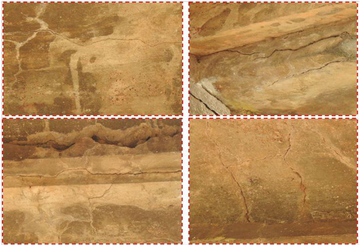
h) Cracks observed at Flight-1 of Staircase-2
