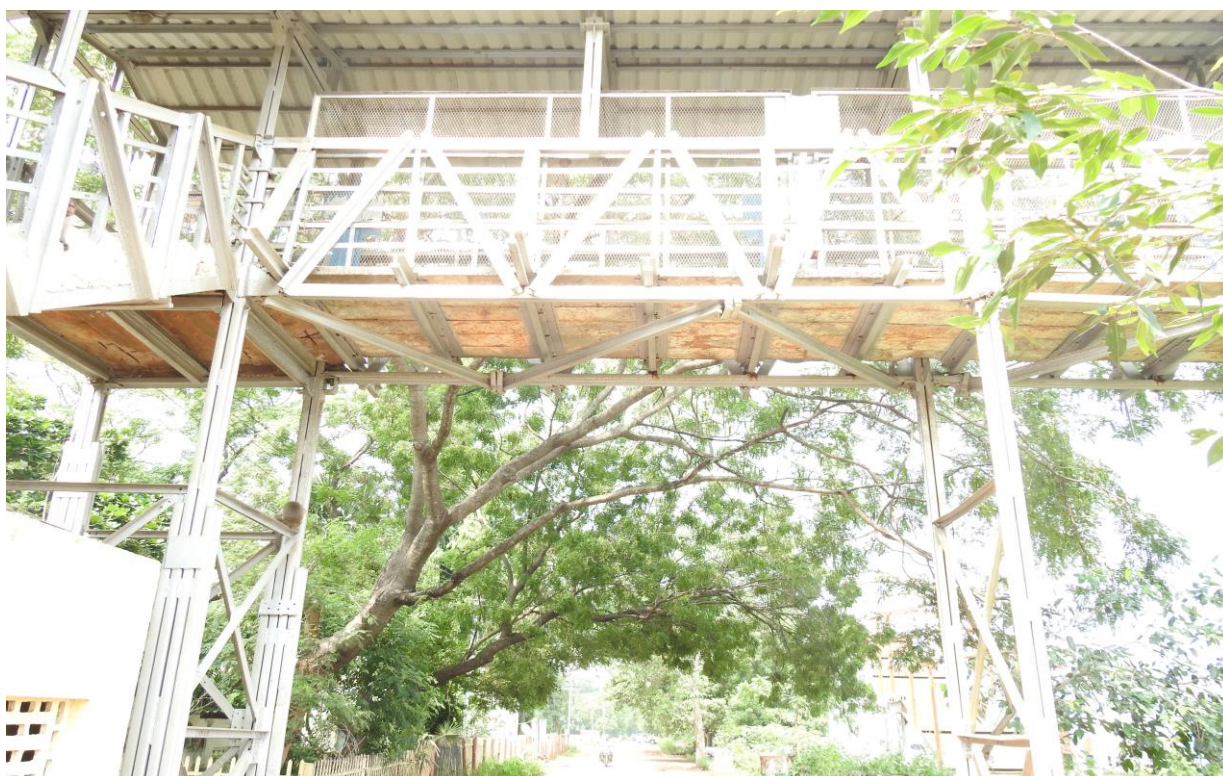
Fig 1.1: Front & Bottom view of span-1
