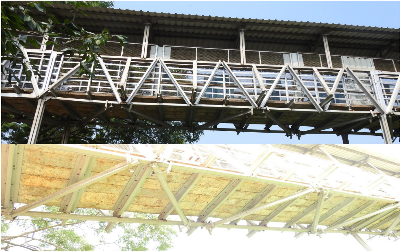
Fig 1.2: Front & Bottom view of span-2
