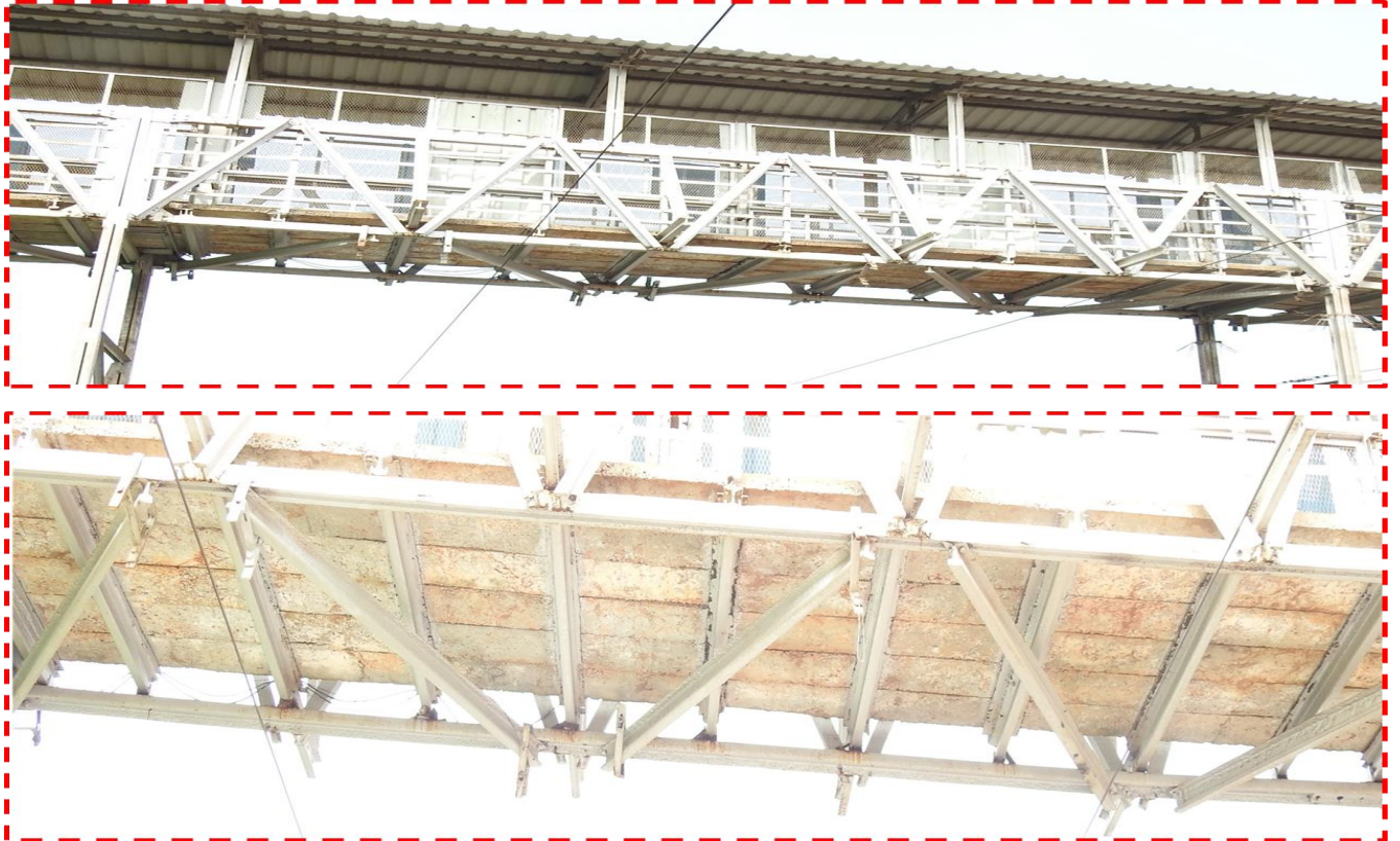
Fig 1.4: Front & Bottom view of FOB span-4
