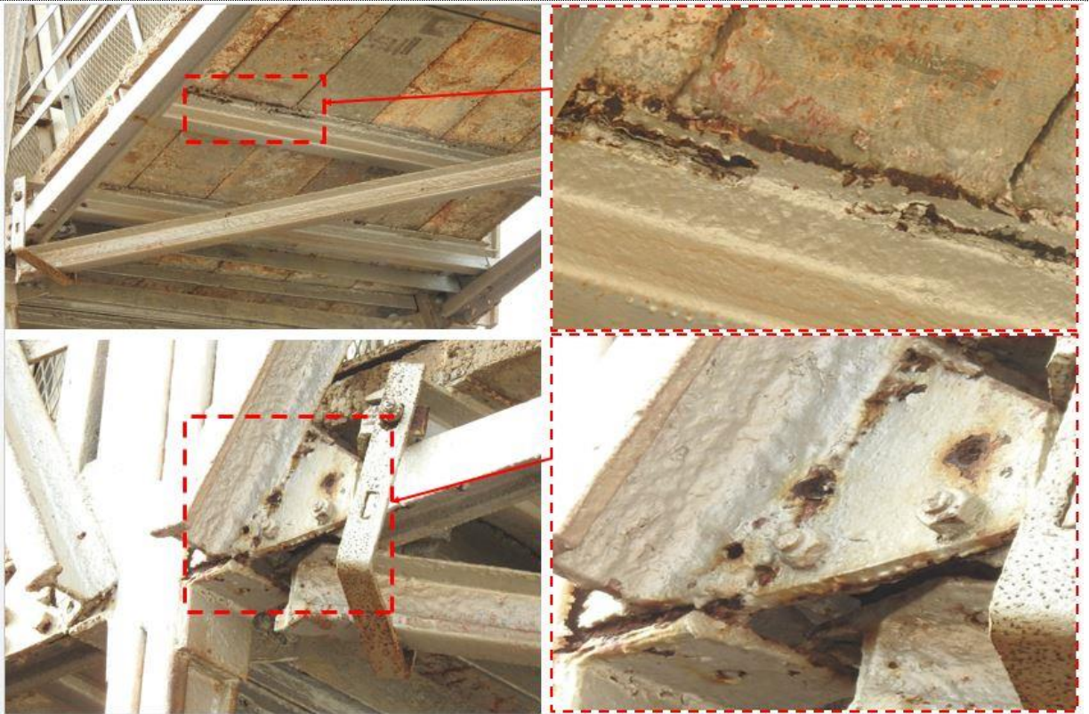
f) Corrosion observed at Floor beam & cleat angles of Span-6
