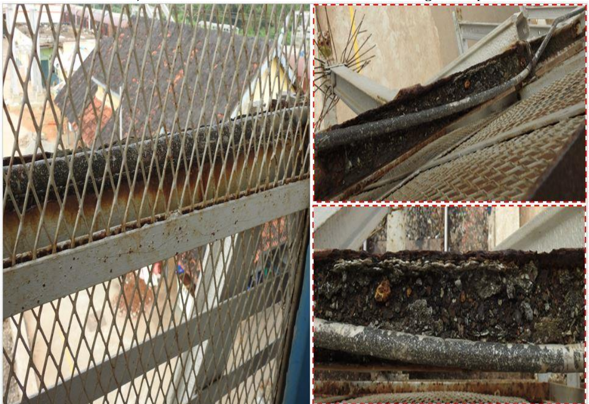
f) Corrosion observed at Floor beam & cleat angles of Span-6
