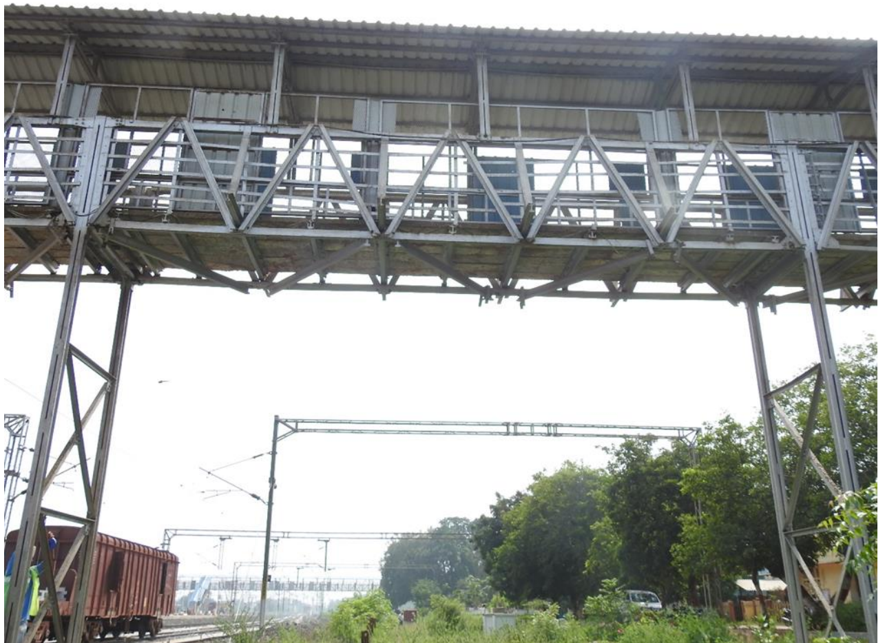
Fig 1.3: Front & Bottom view of span-3
