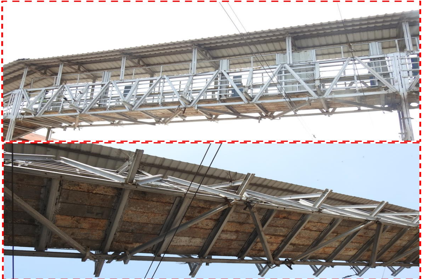
Fig 1.6: Front & Bottom view of FOB span-6
