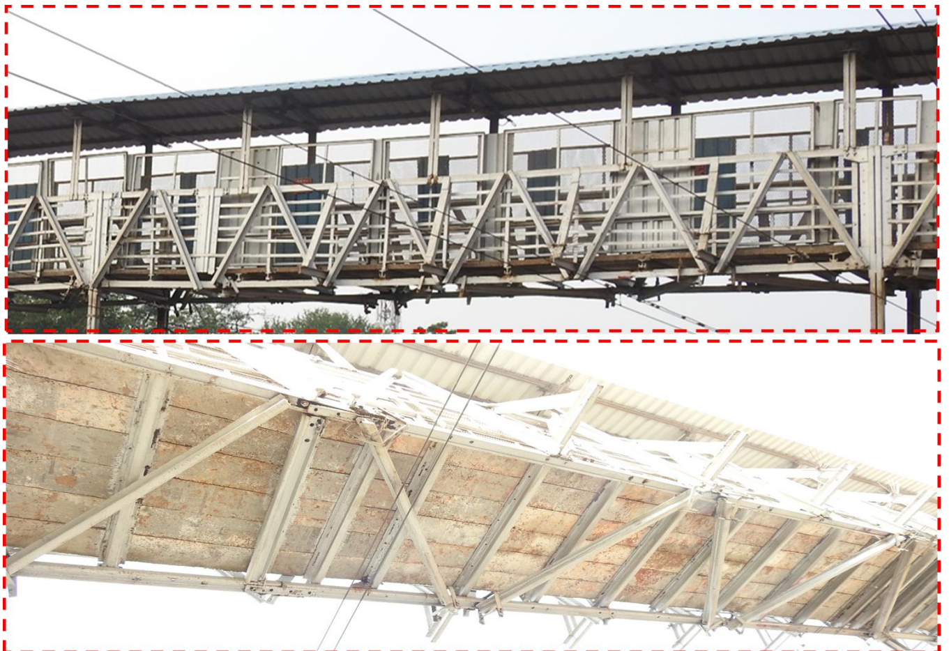
Fig 1.5: Front & Bottom view of FOB span-5
