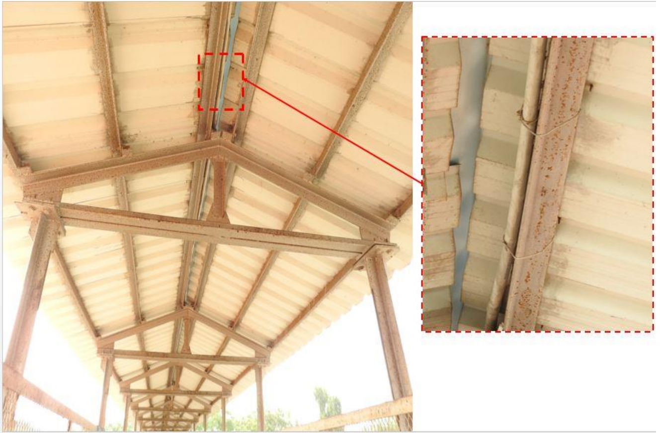
Fig 1.8: Additional loads of PVC pipes
