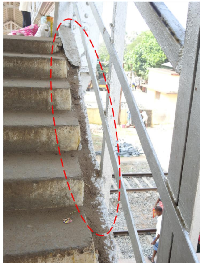
Fig: 2.4 Corrosion of Stringer beams
