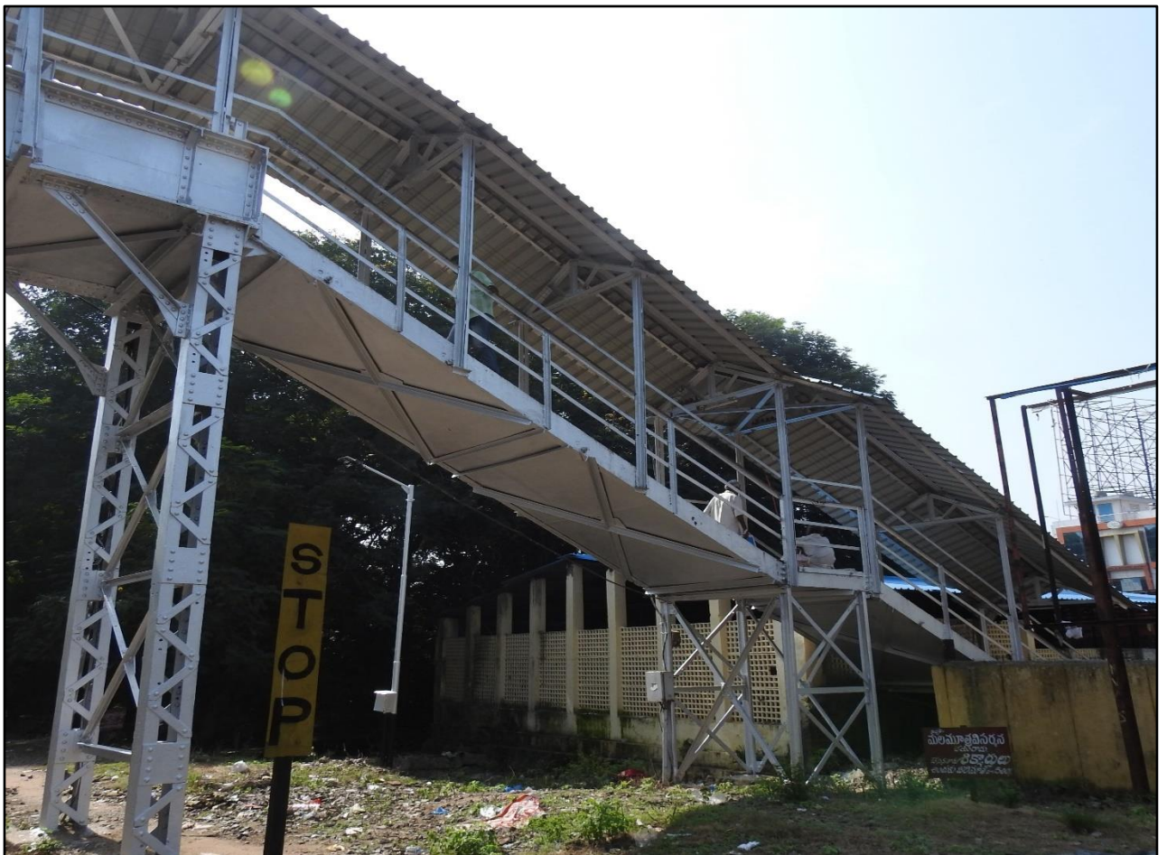
Fig1.8: Staircase Bottom view
