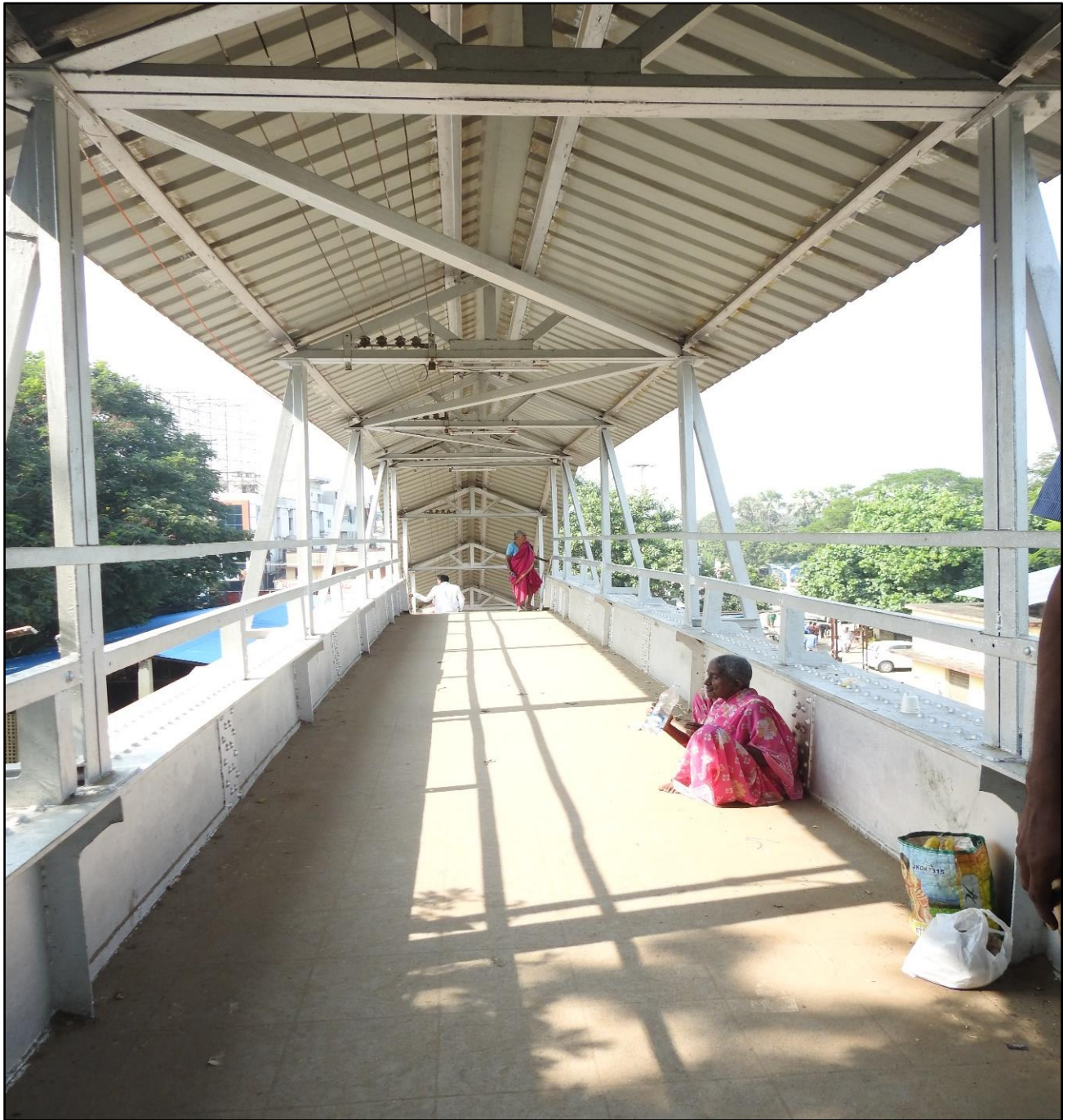
Fig 1.2: Pathway, Steel Railing of FOB
