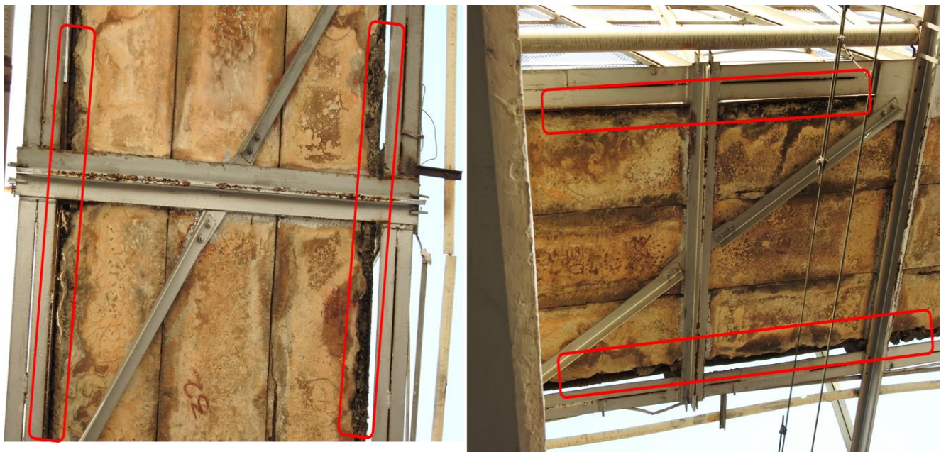
Fig 3.9: Exposed reinforcement in slab panels at span-3
