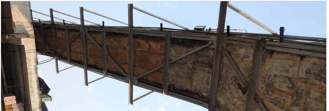
Fig 1.3: Front view and bottom view of span 1
