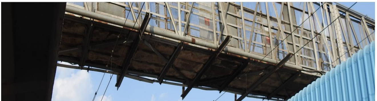
Fig 1.5: Front view and bottom view of span 3
