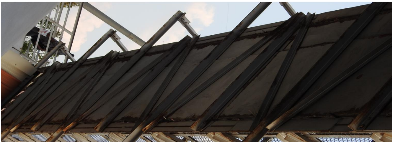
Fig 1.7: Front view and bottom view of span 5
