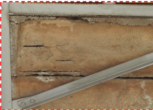
Spalling and reinforcement exposure in span 1
