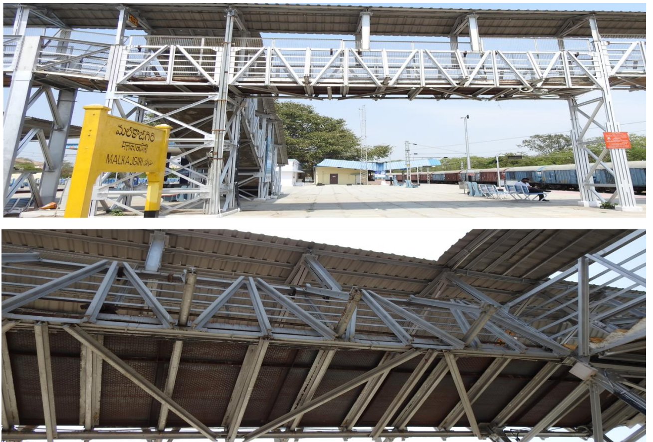
Fig 1.4: Front view and bottom view of span 2
