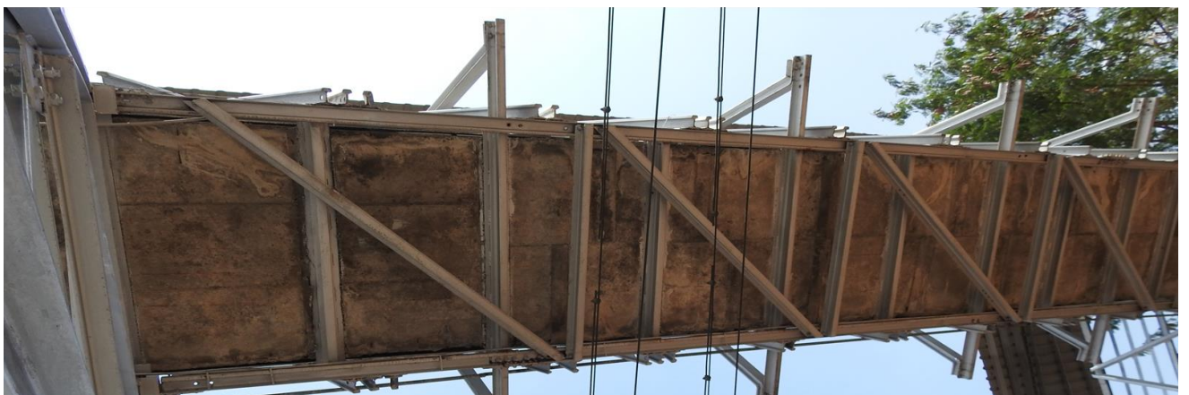
Fig 1.6: Front view and bottom view of span 4
