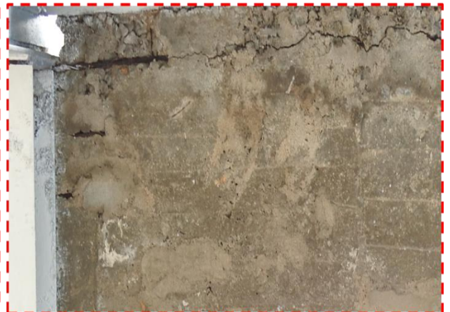
Spalling and reinforcement exposure in span 1
