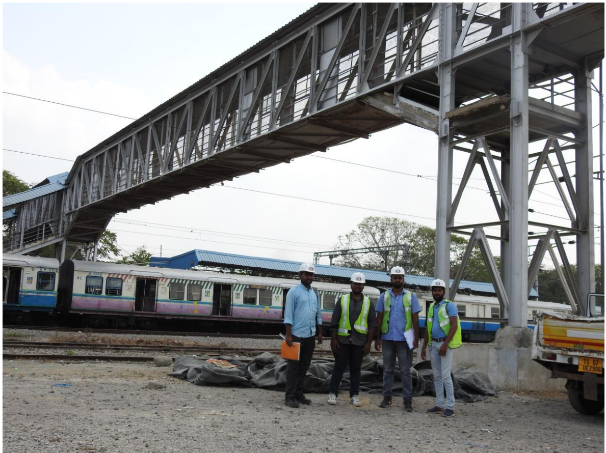
Fig 1.7: Inspection team at Falaknuma FOB
