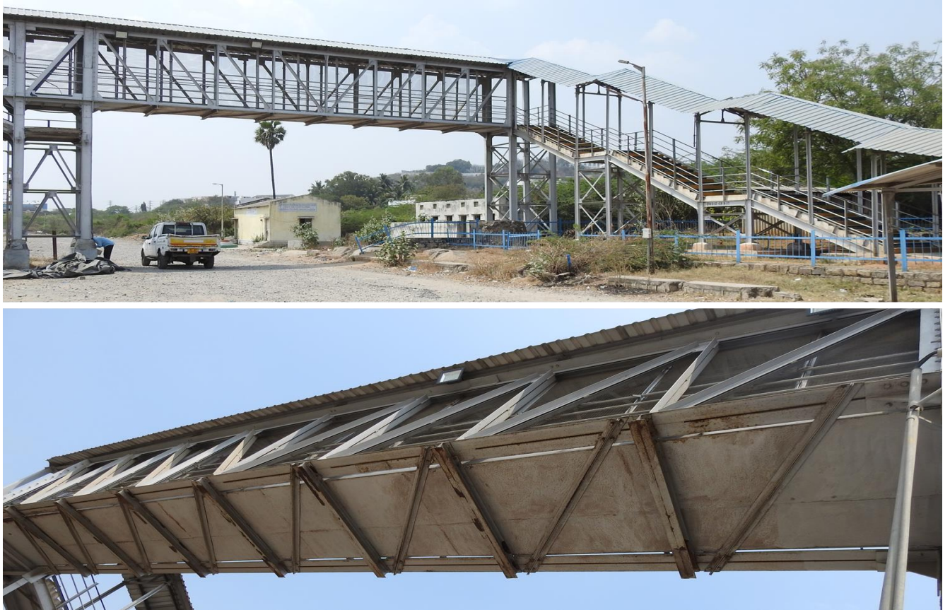
Fig 1.5: Front view and bottom view of span 3
