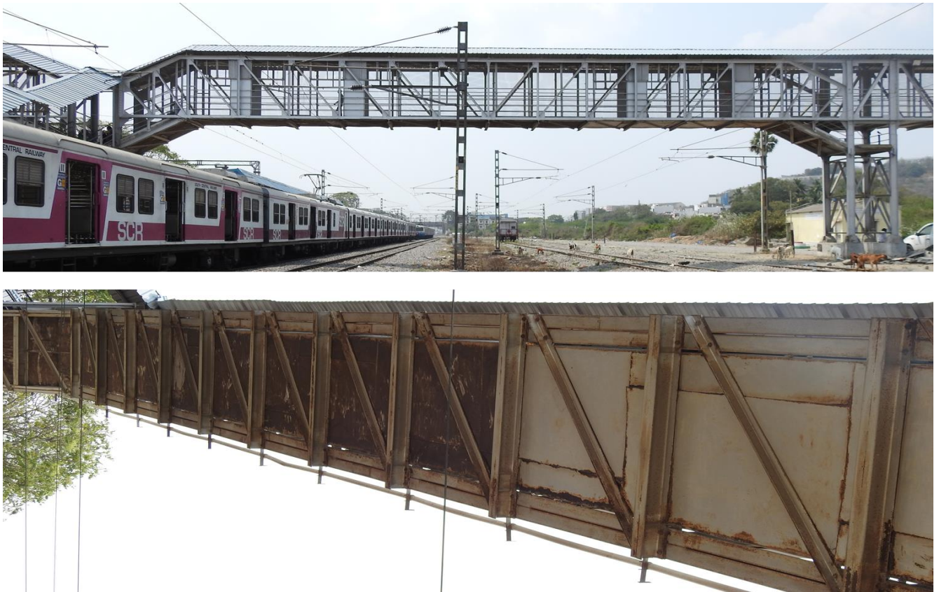
Fig 1.4: Front view and bottom view of span 2
