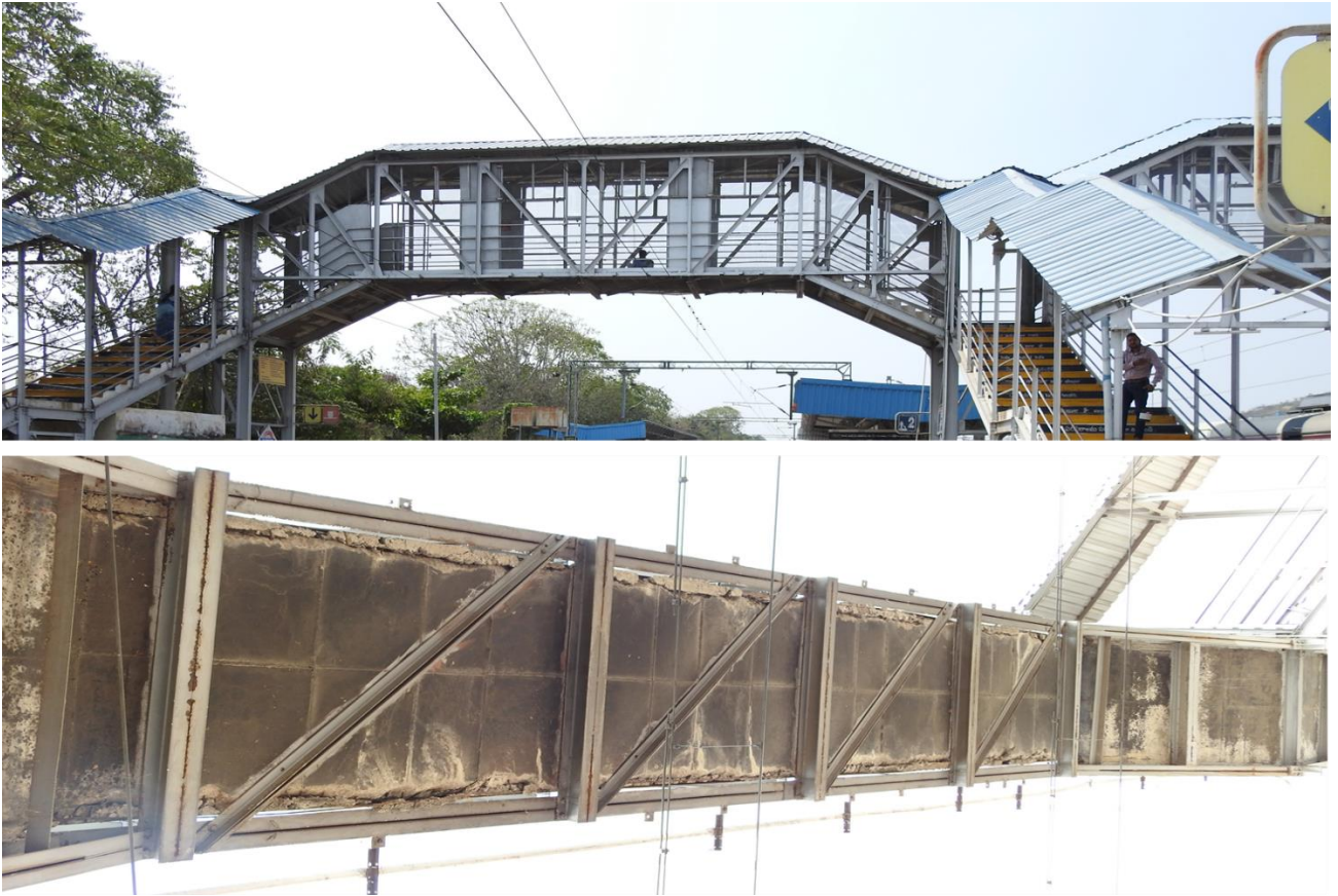
Fig 1.3: Front view and bottom view of span 1
