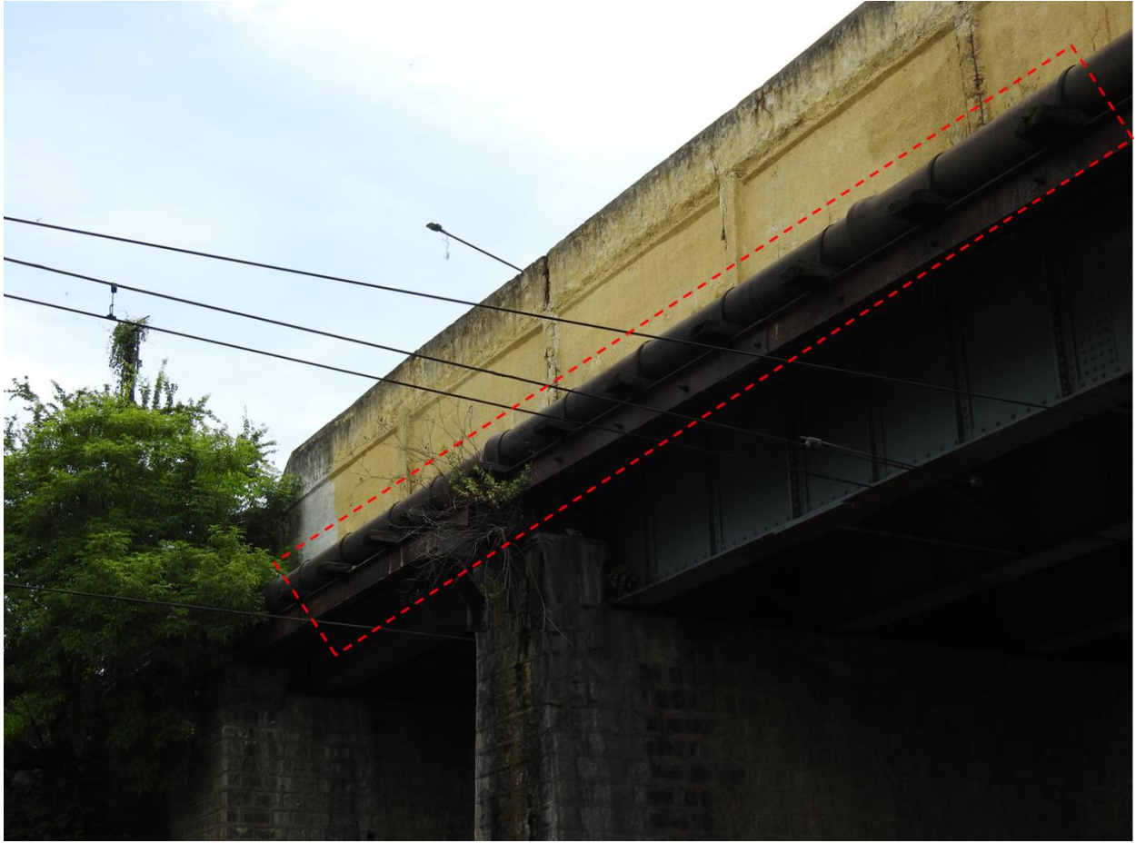
Fig: 1.9 Additional load of utility is observed
