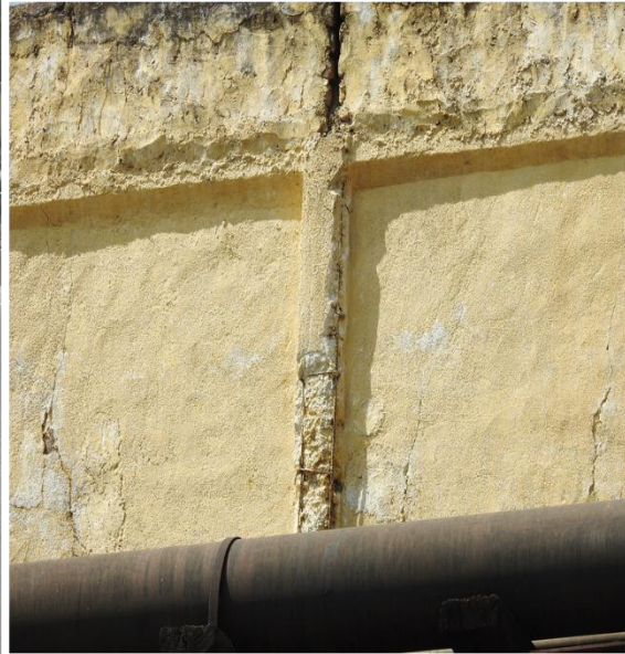
Fig: 1.13 Cracks on parapet wall
