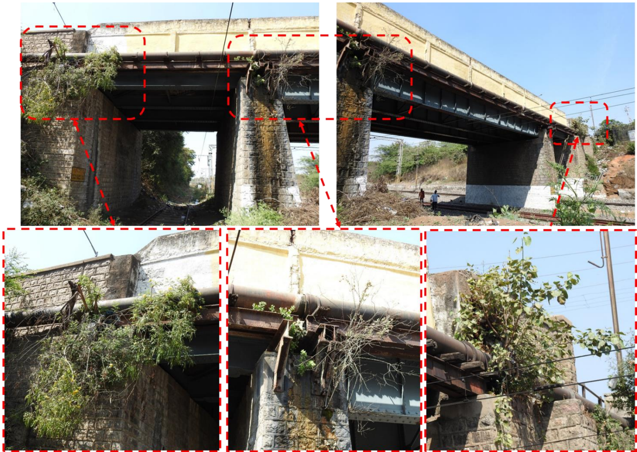
Fig 3.8 : Vegetation observed on the top of the pier (abutment wall)
