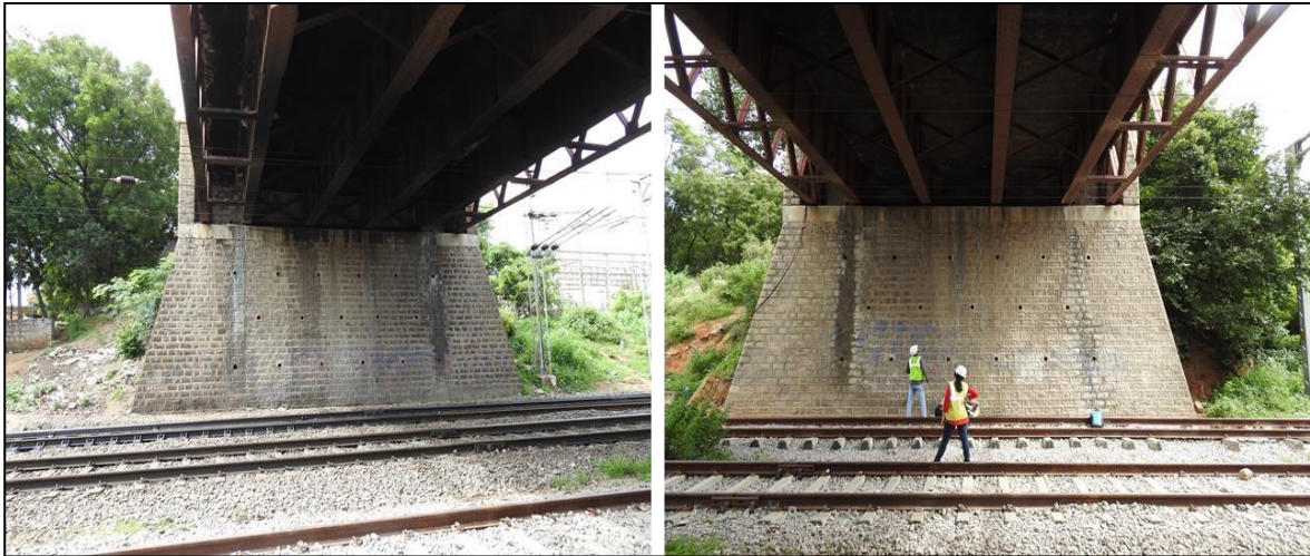
Fig 1.1: Stone masonry abutments
