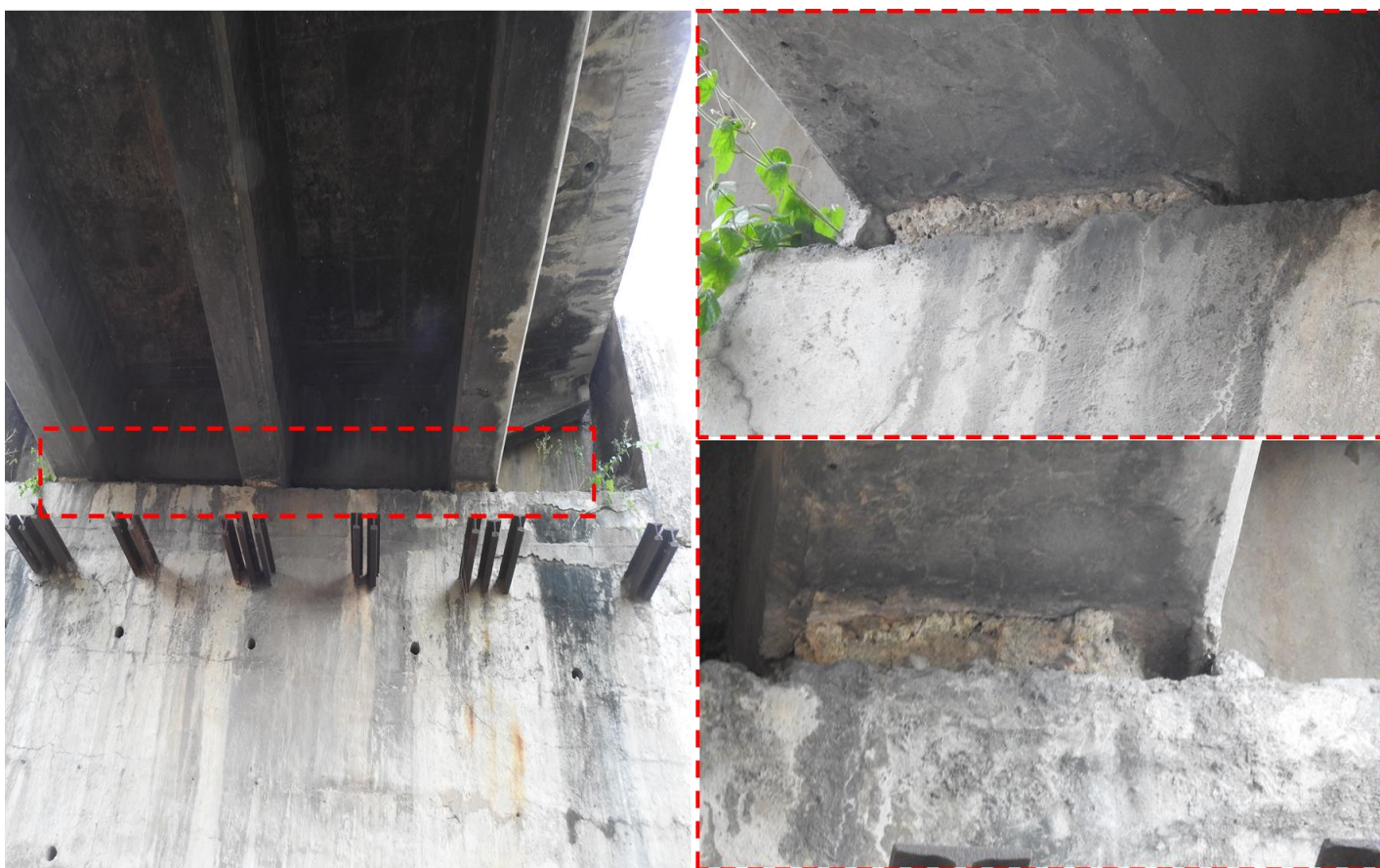
Fig 4: Bearings at Abutment 1
