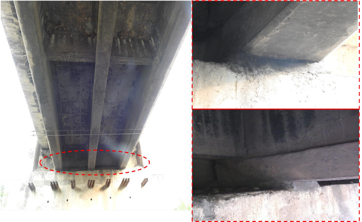
Fig 5: Bearings at Abutment 2
