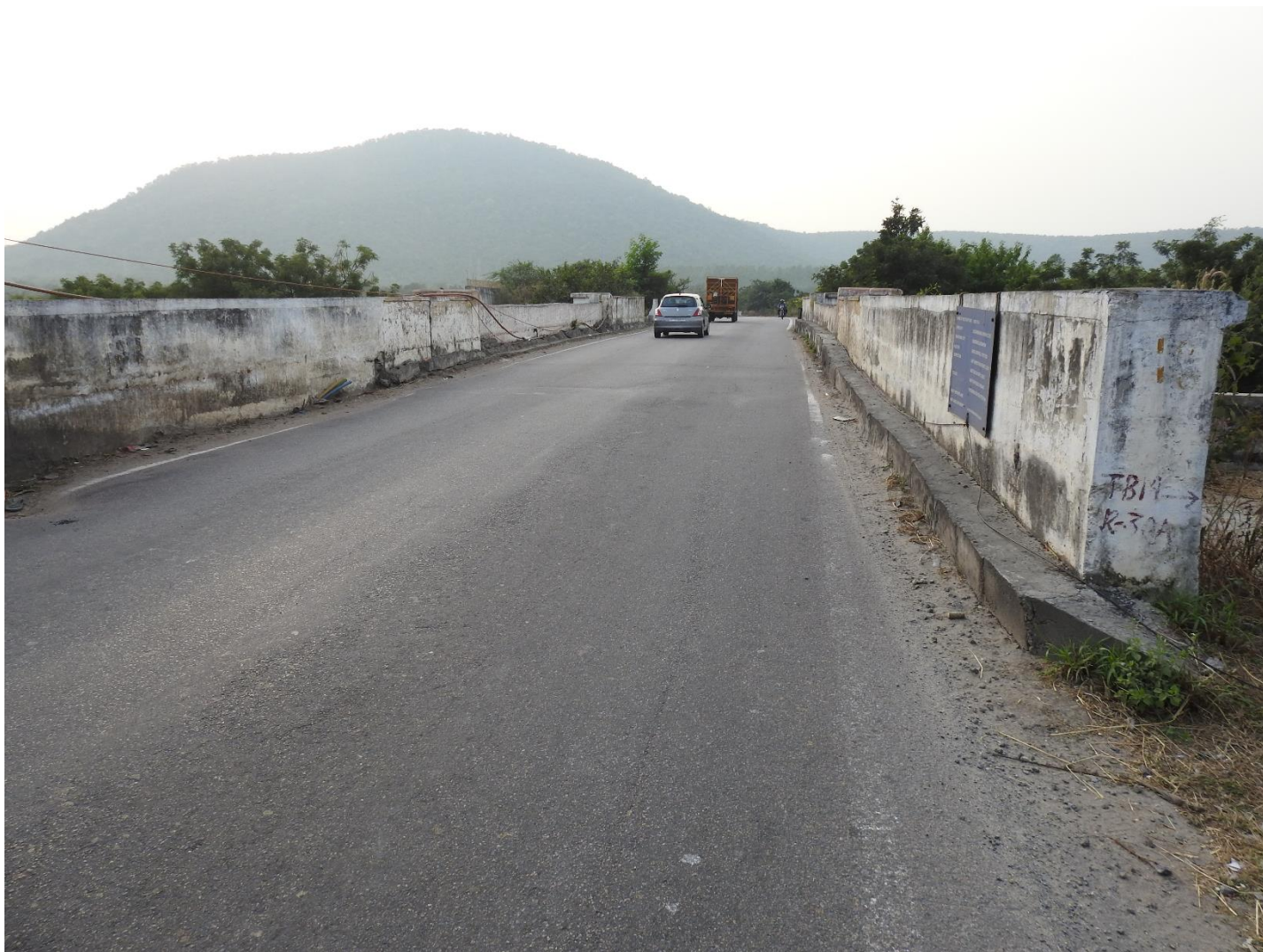
Fig 13: Wearing coat & Parapet wall
