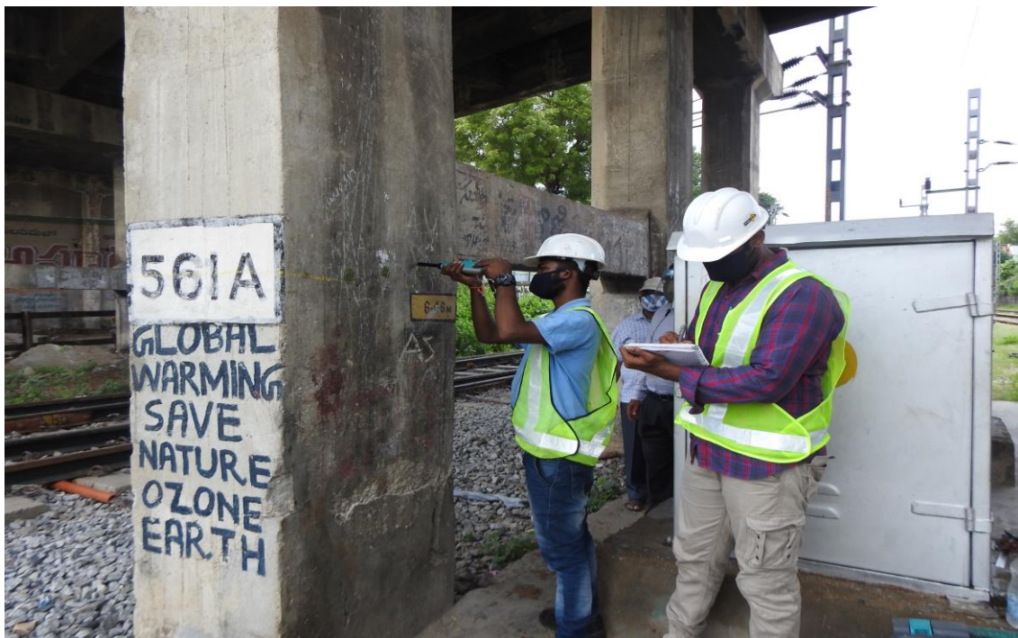
Fig 16: Rebound hammer test at site
