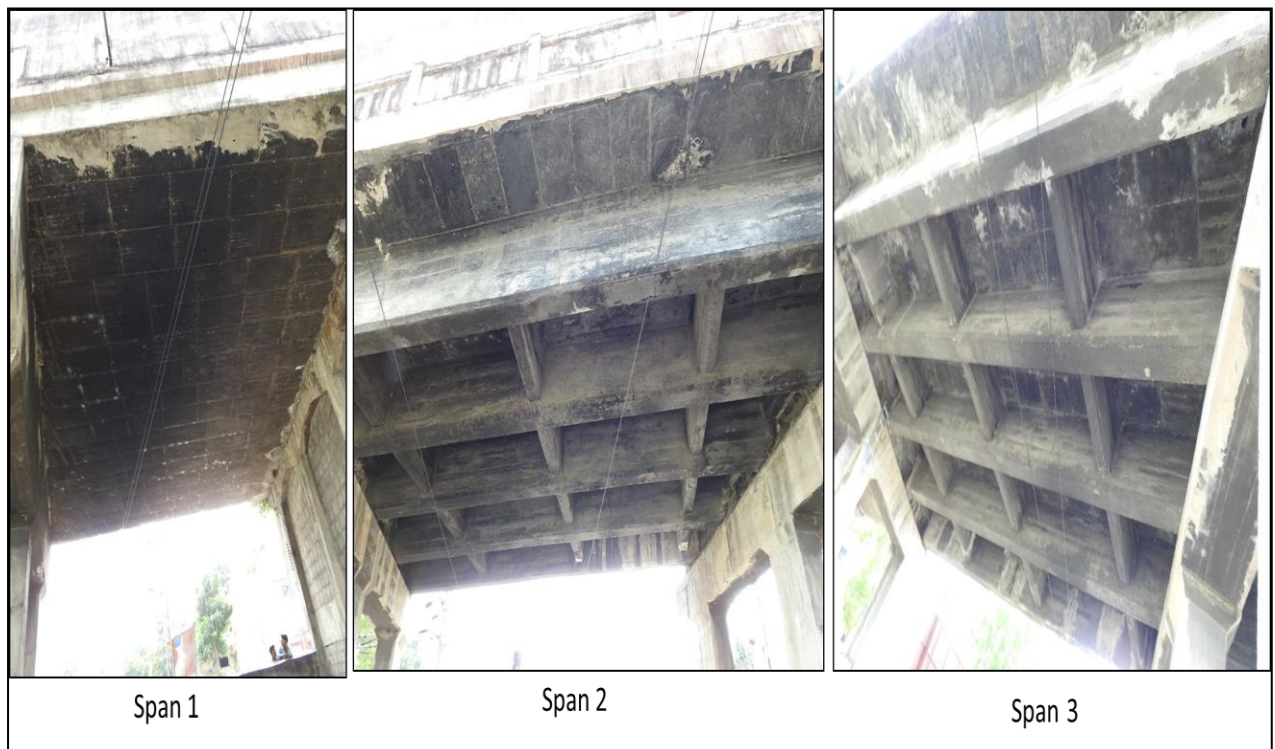
Fig 2: Bottom view of the Bridge
