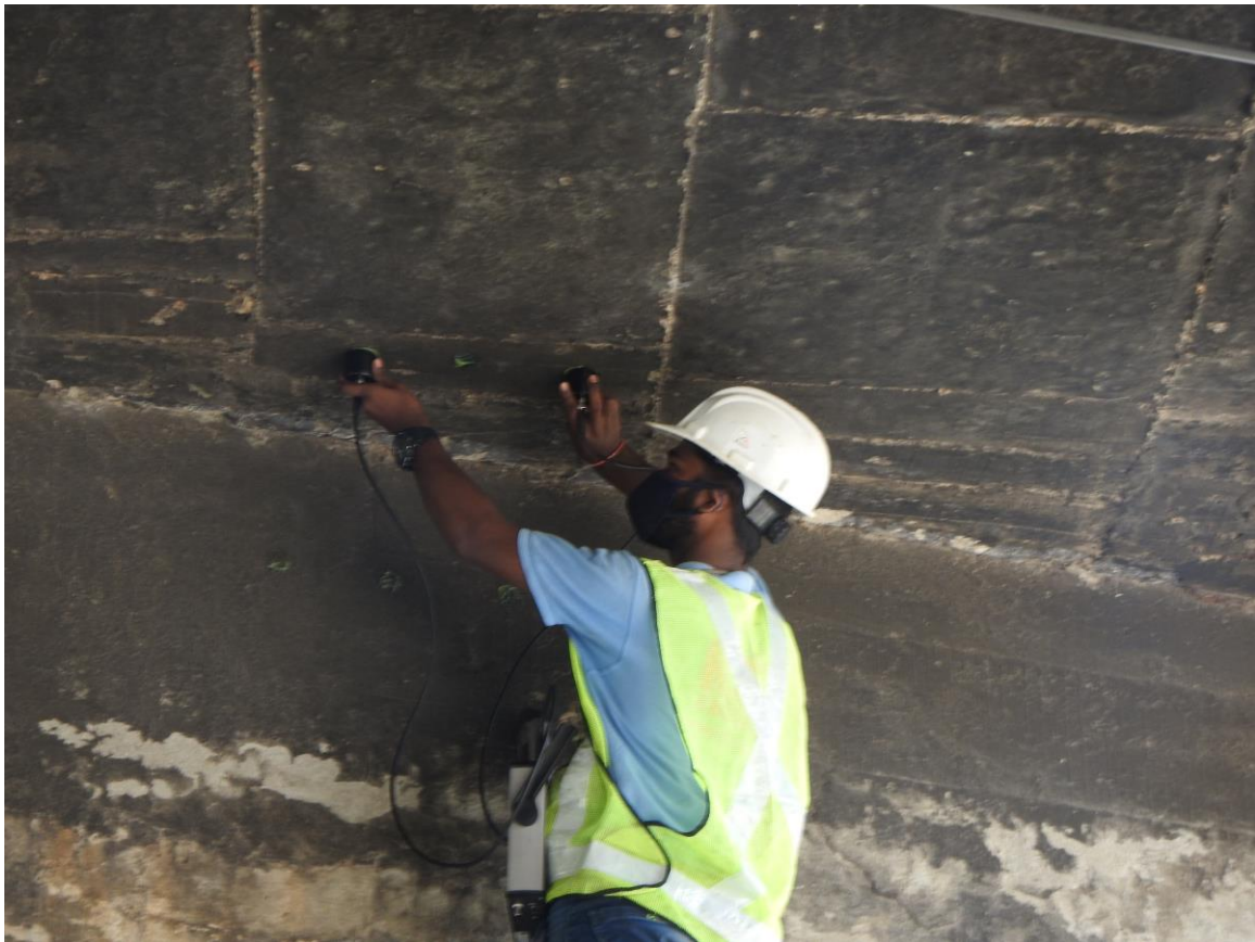
Fig 15: UPV test at site
