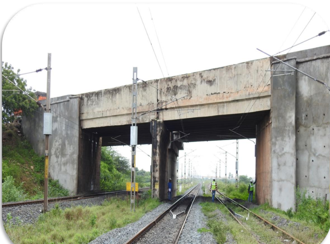
INSPECTION OF ROB NO.295A NEAR KOMMALAPUDI RAILWAY STATION
