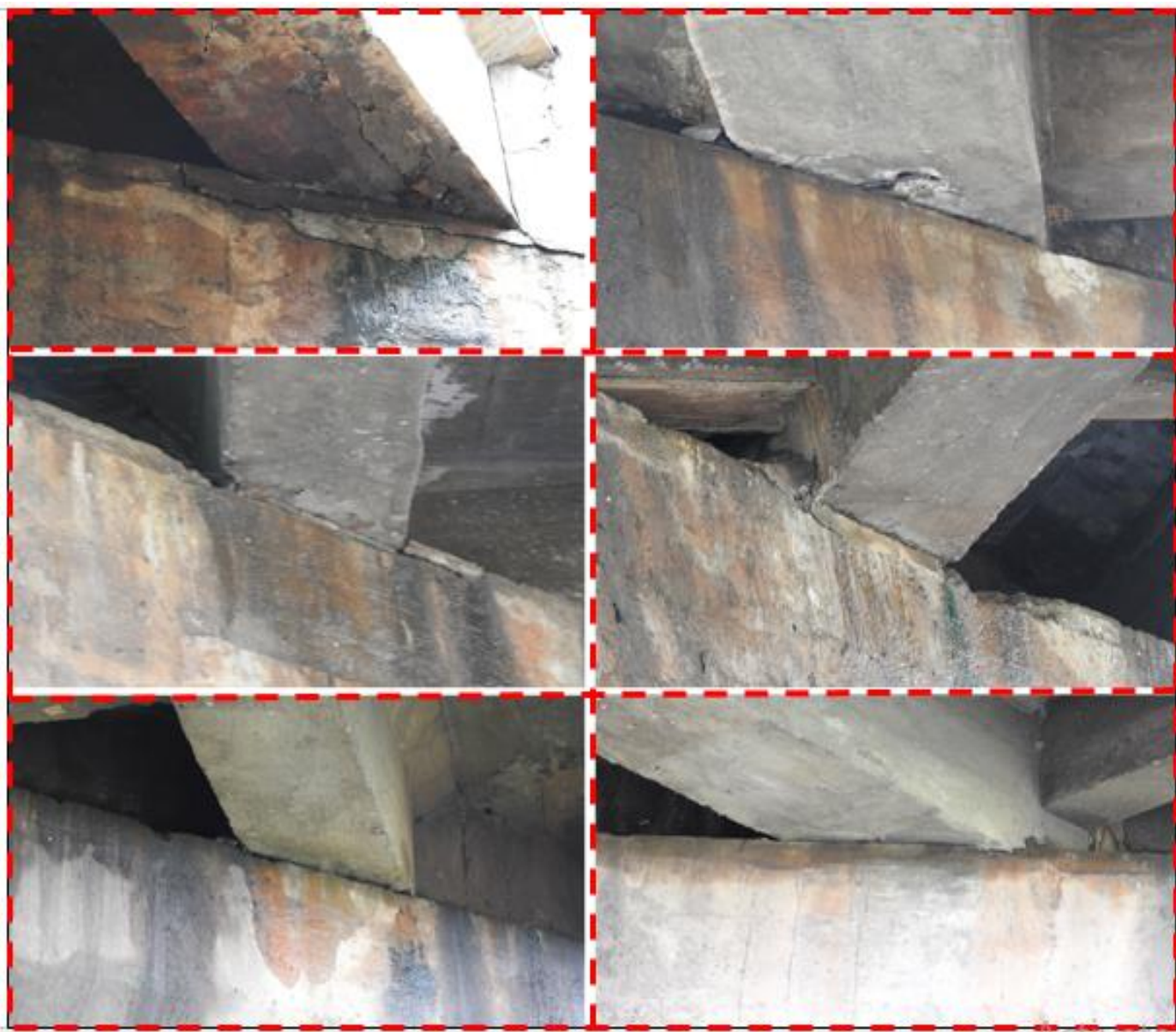
Fig 15: Bearings settled.
