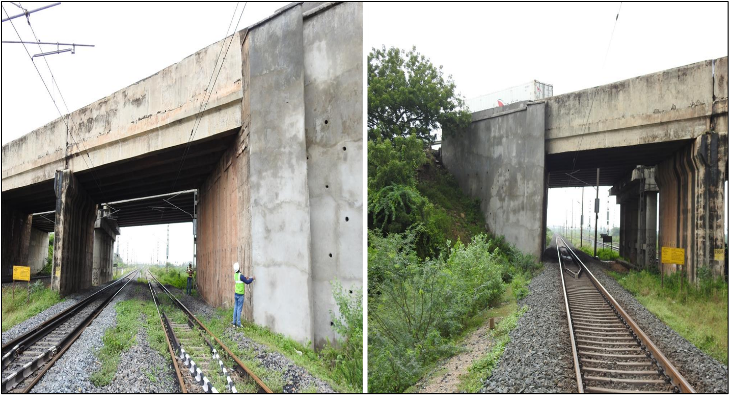
Fig: 2 View of Abutments (A1 and A2)
