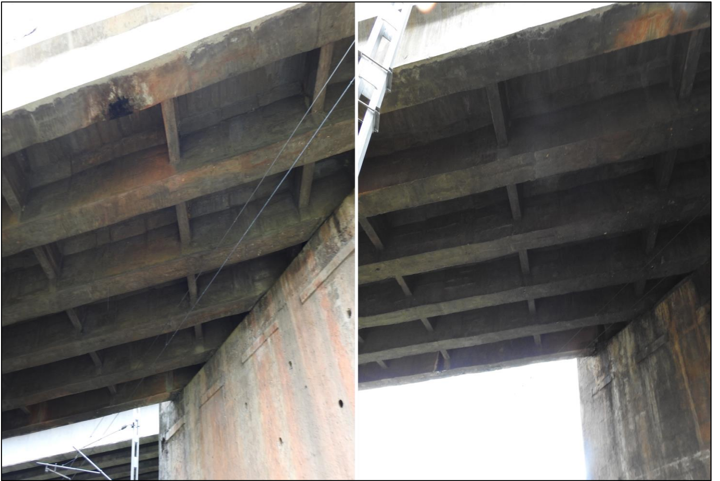
Fig: 3 Bottom view of Bridge
