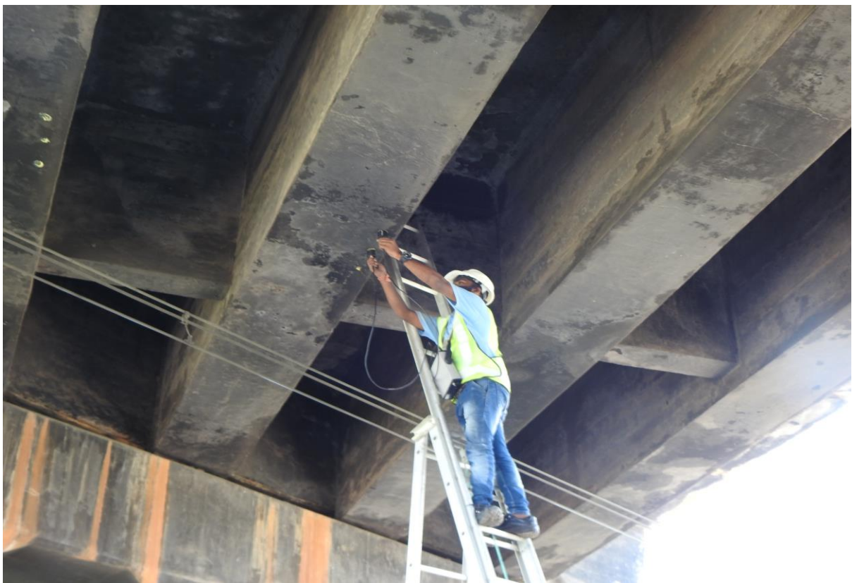
Fig 18 UPV test at site
