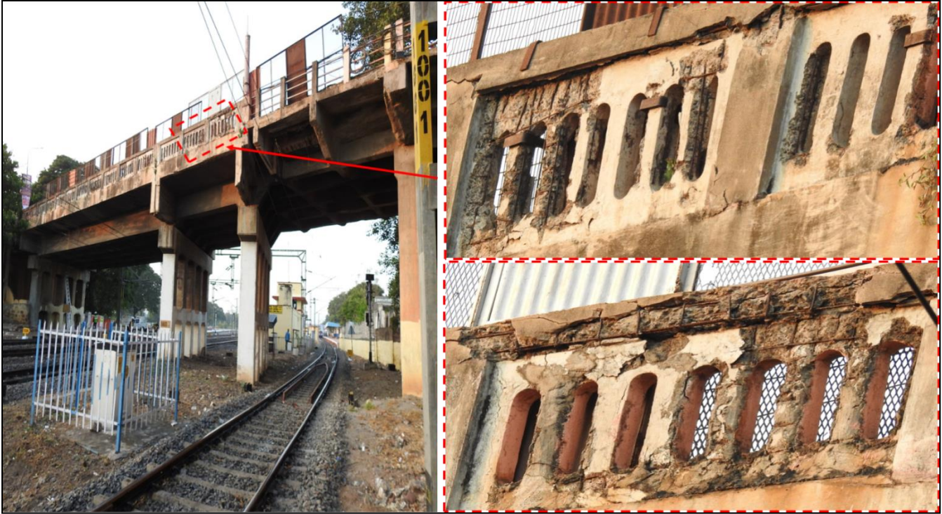
Fig: 4 Condition of parapet wall / Railing
