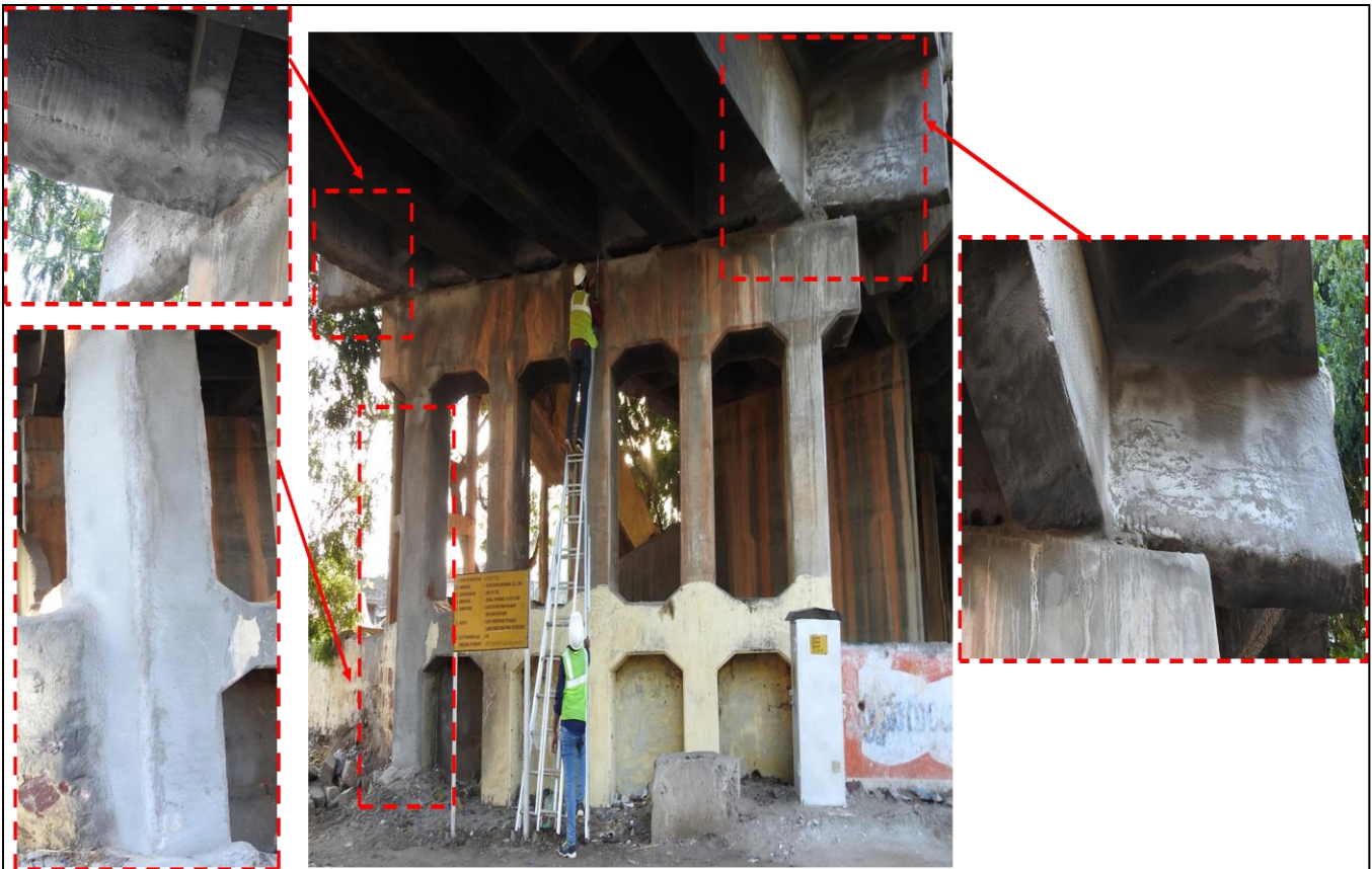
Fig 5: Shotcreting observed in pier-1 columns & Girders
