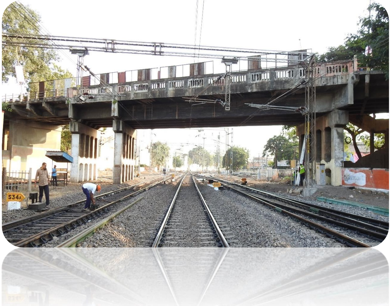
INSPECTION OF ROB NO. 660A NEAR TENALI RAILWAY STATION
