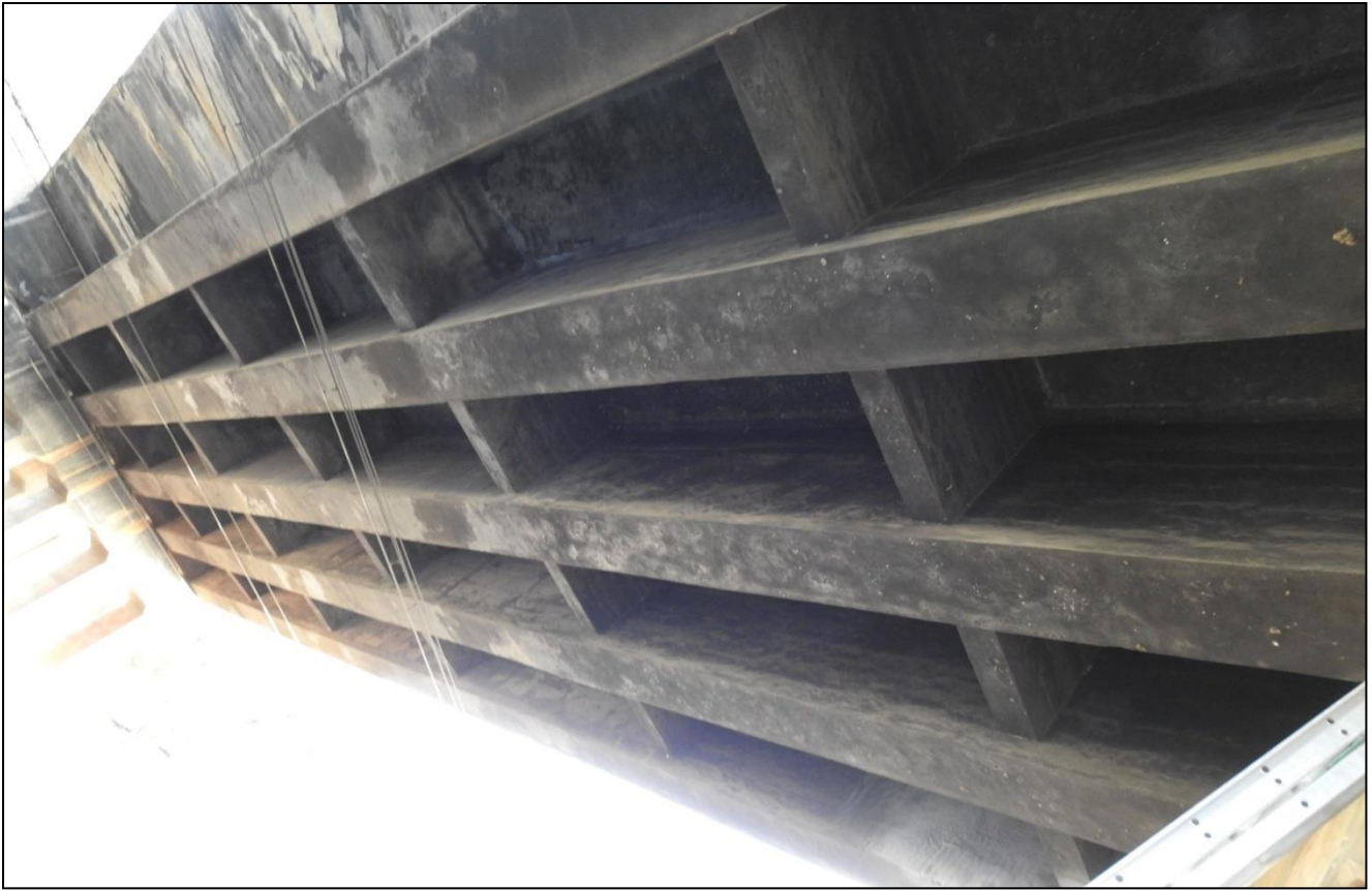
Fig: 2 Bottom view of Bridge
