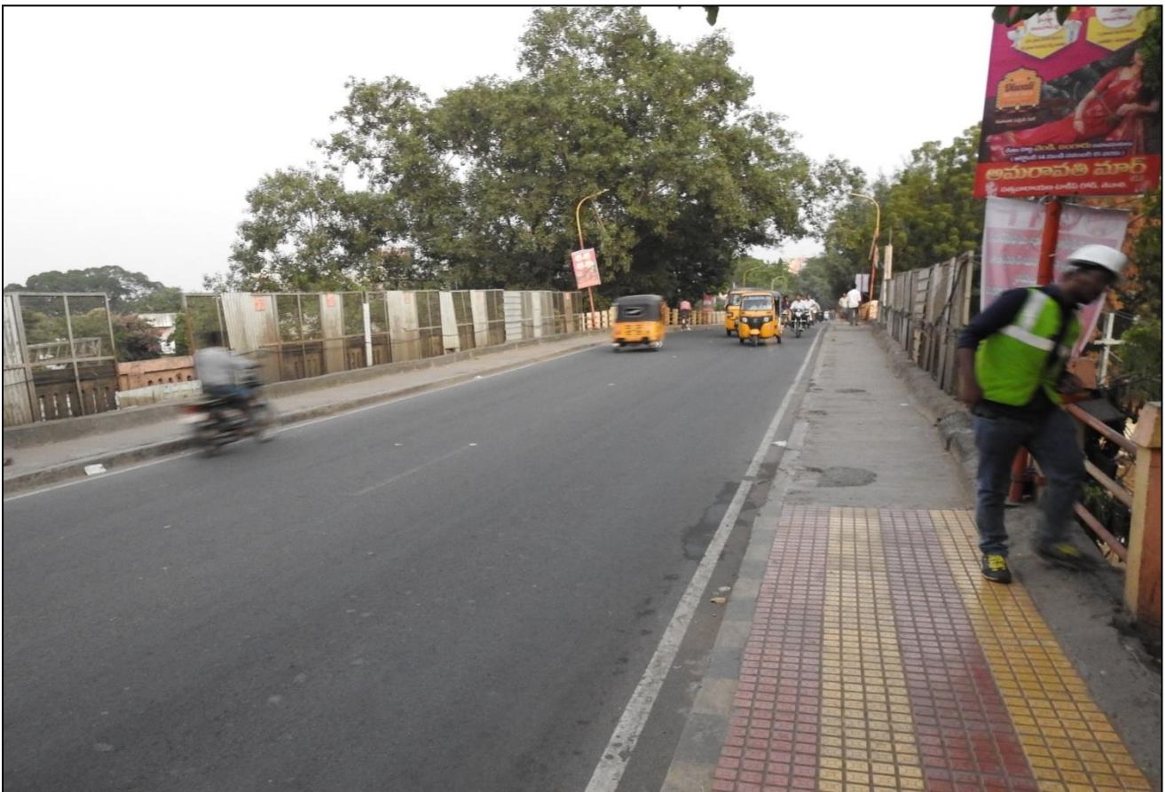
Fig: 3 Top view of the Bridge / Condition of Wearing coat
