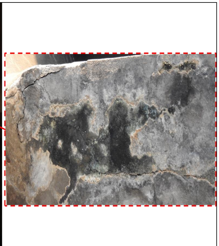
Fig 8&9: Severe cracks & Vegetation observed in end of the cross girders
