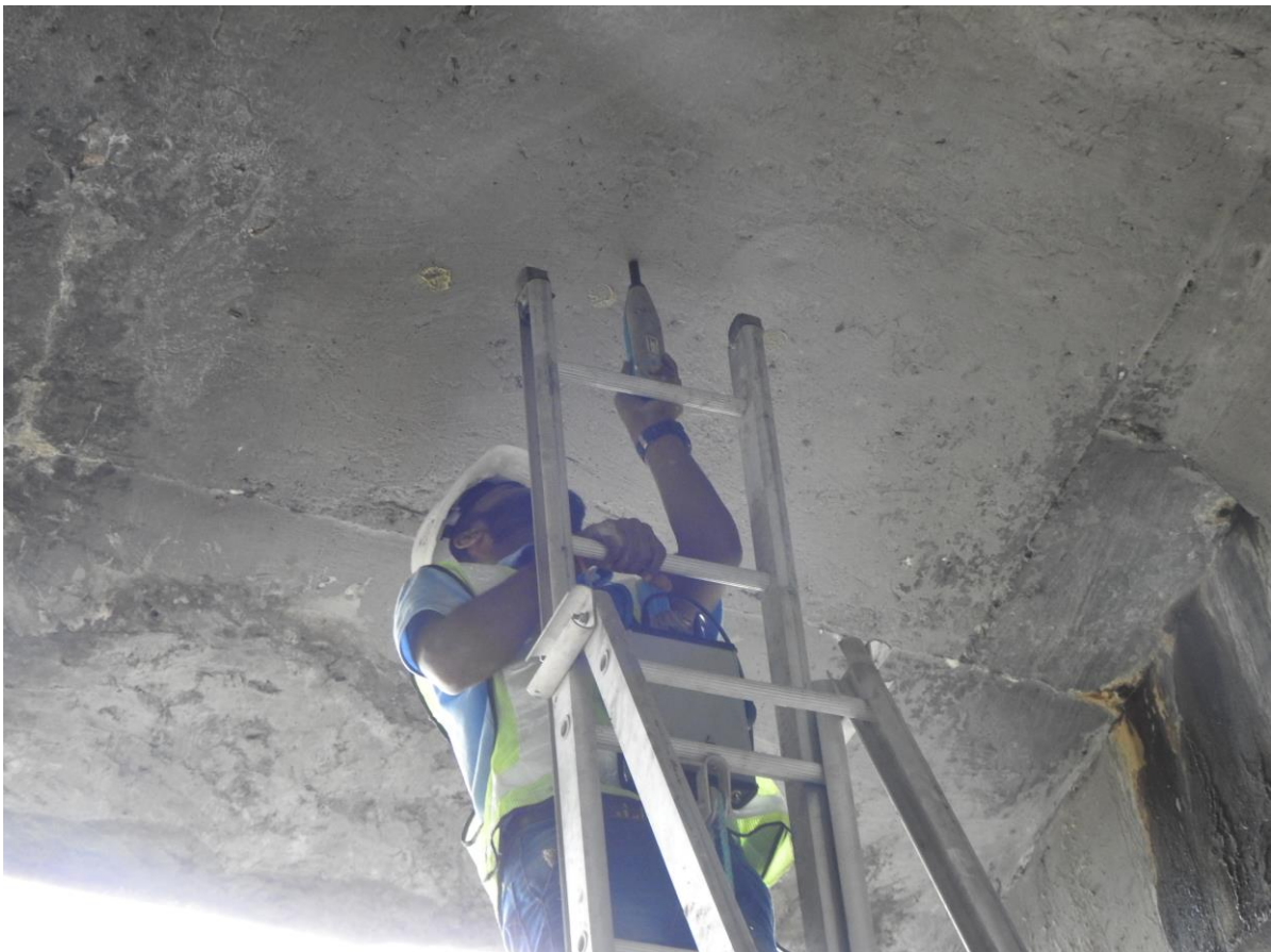
Fig 18: Rebound hammer test at site
