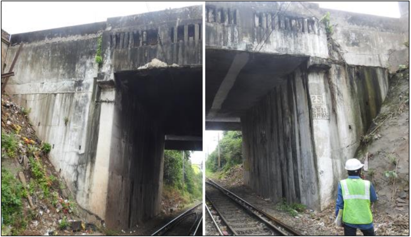
Fig: 2 Abutments (A1 and A2)
