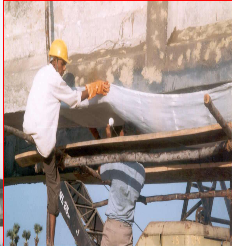
Application of Nitowrap System to soffit of Girders
