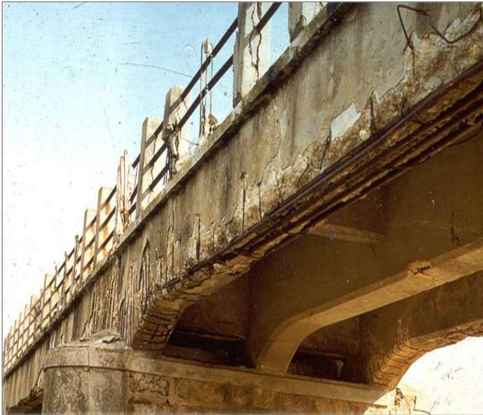
Combined Carbonation and Chloride Attack
