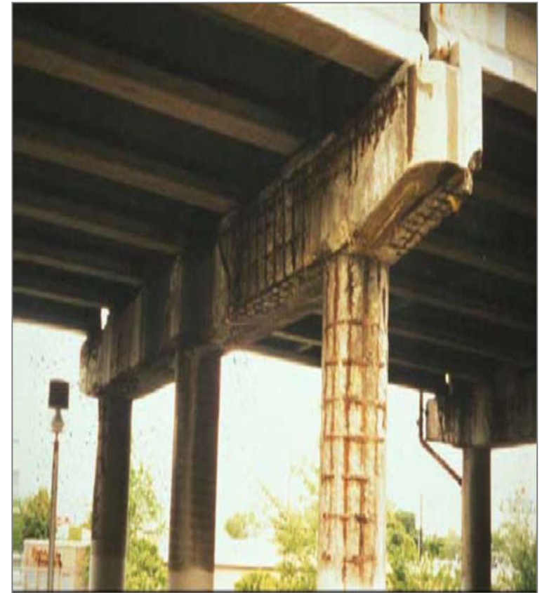
Combined Carbonation and Chloride Attack
