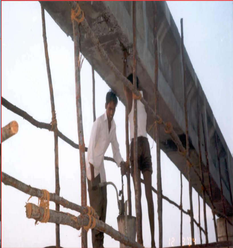
Pressure grouting in progress
