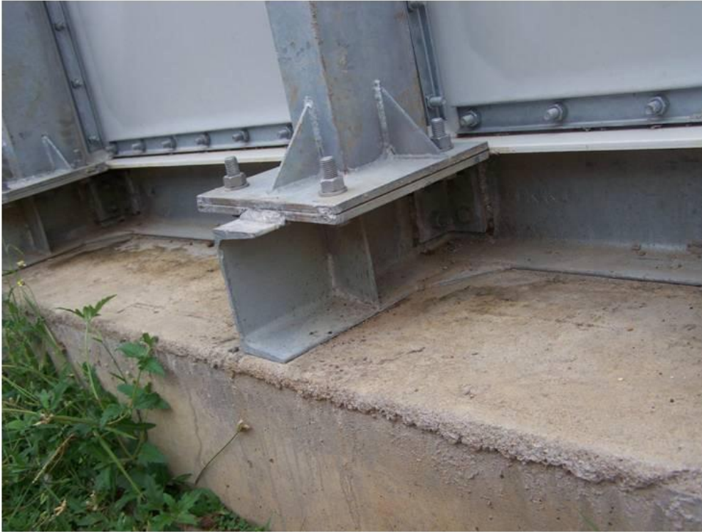
External Supports - Welded
