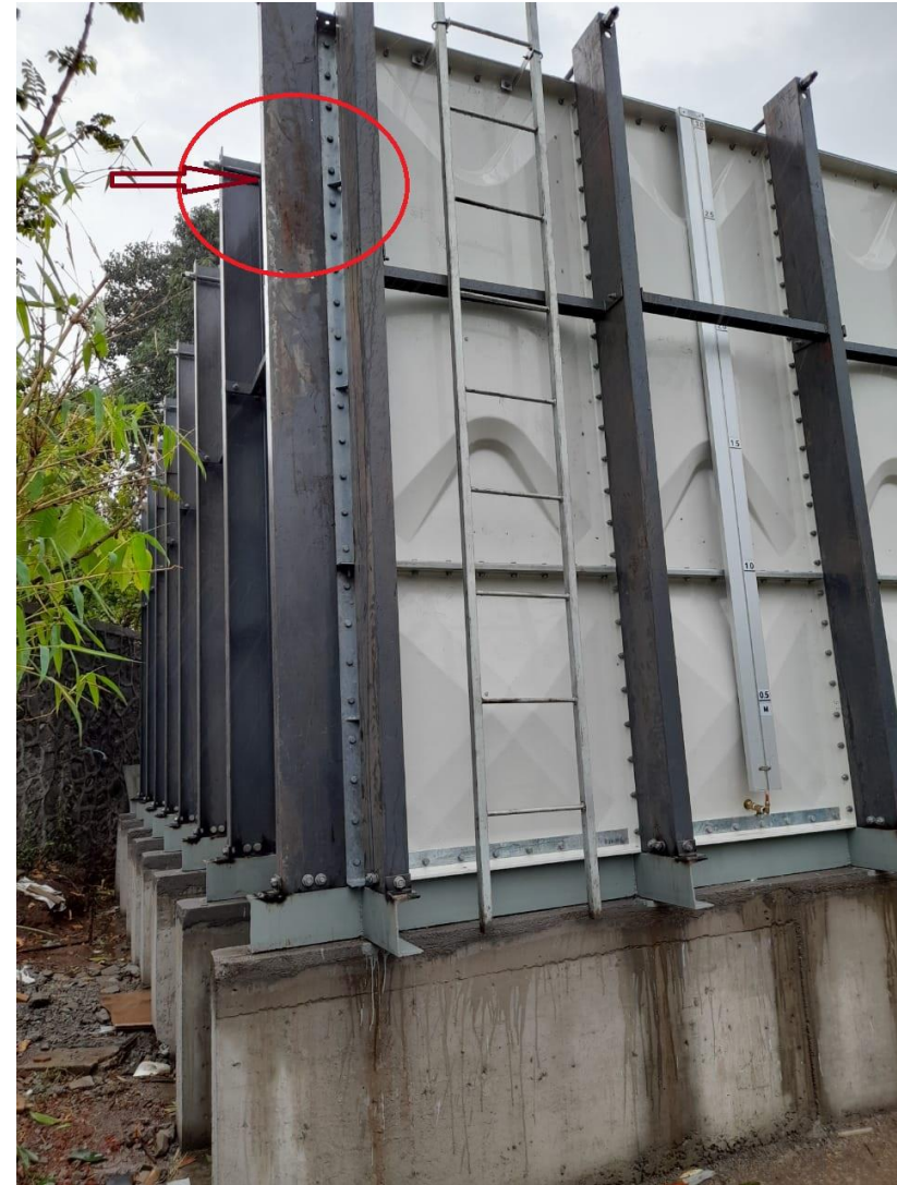
External Supports - Painted
