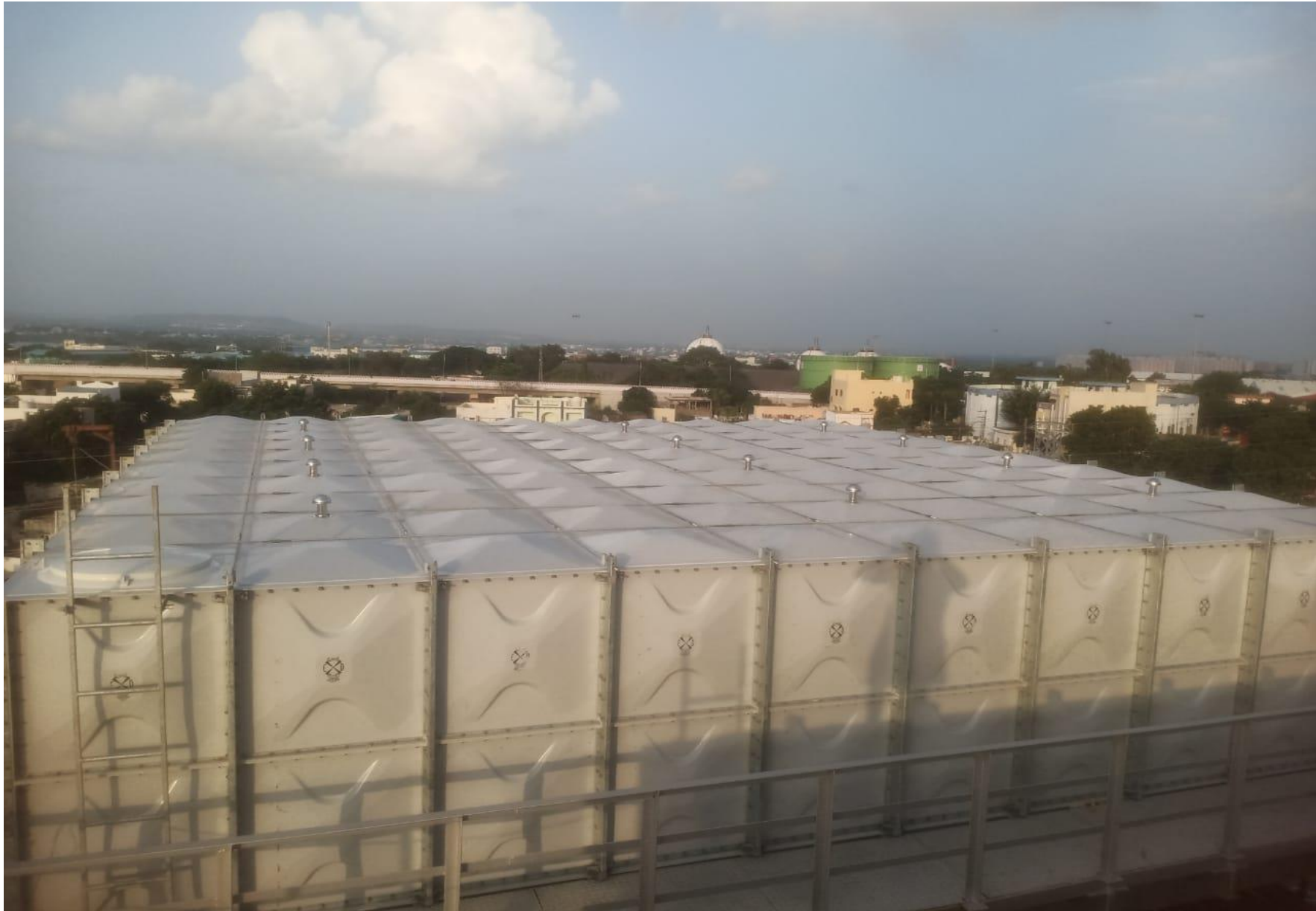
Top Tie rod Arrangement
