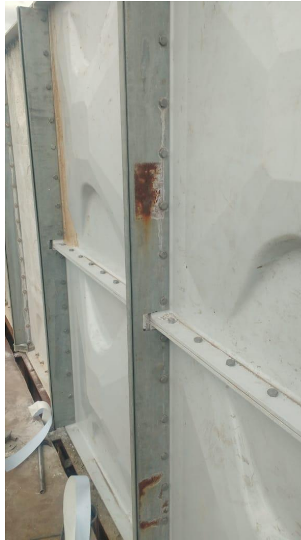
Tank After Repair
