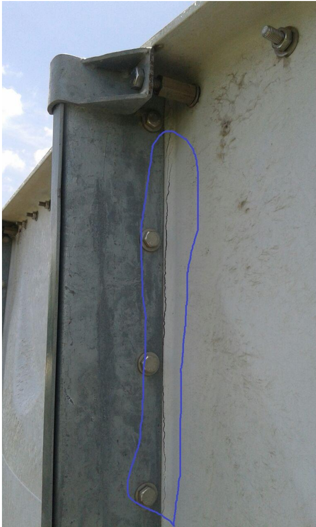
Tank Before Repair
