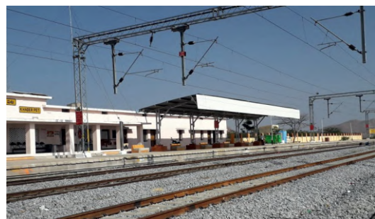
Electrification of Guntakal - Kalluru section
