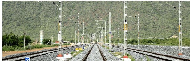
Obulavaripalli - Venkatachalam new Railway line
