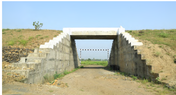
Elimination of level crossing gates by constructing limited height subways in the state of Andhra Pradesh
