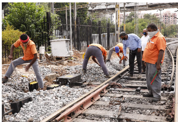
Track Maintenance in progress
