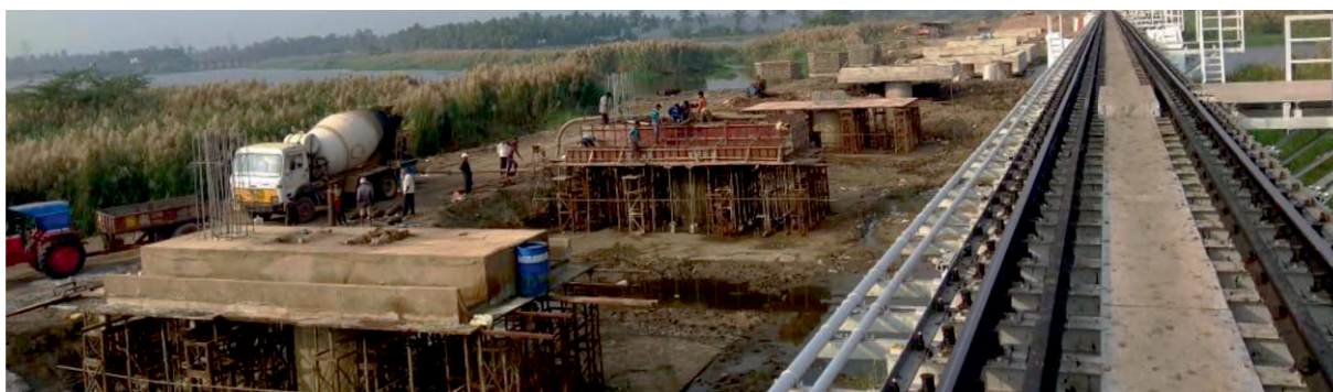
Double line works between Moturu - Akividu in Gudivada - Bhimavaram section
