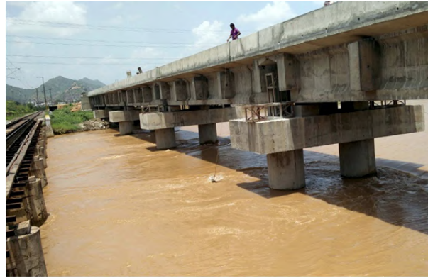
Major bridge in Vijayawada- Kondapalli section
