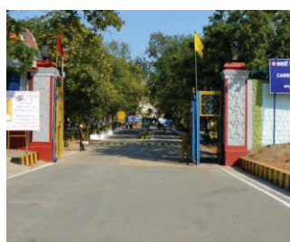
Carriage Repair Shop, Tirupati - "Gold rating"
