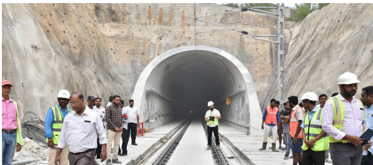
6.6 km Tunnel Constructed between Rapur and Cherlopalli - Longest Electrified Tunnel on Indian Railways
