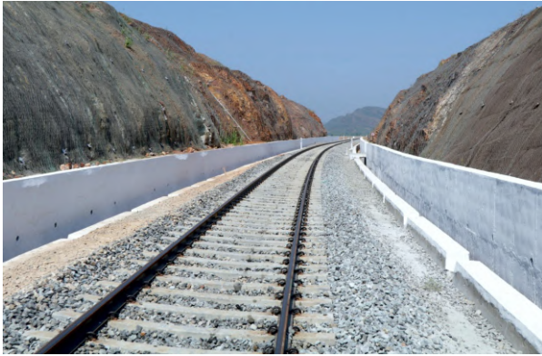
New Railway line between New Piduguralla - Savalyapuram
