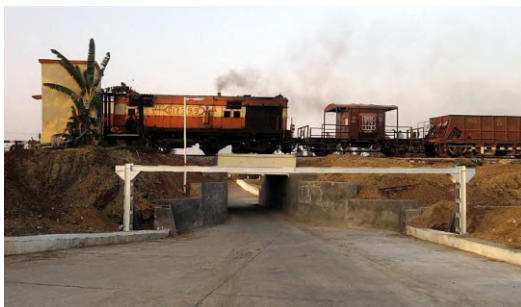
Road under bridge near Guntur
