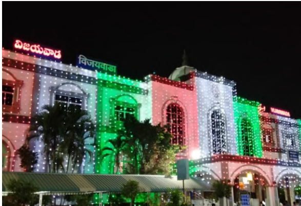
LED-Lit Vijayawada Railway station
