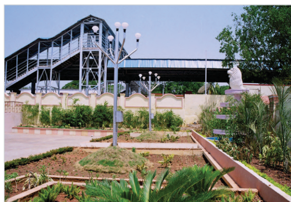
Foot over bridge at Nellore station
