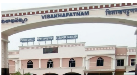
Visakhapatnam Railway station - "Platinum rating"
