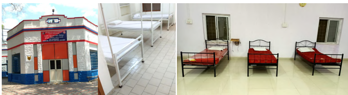
Isolation ward at RPF barracks, Guntur
