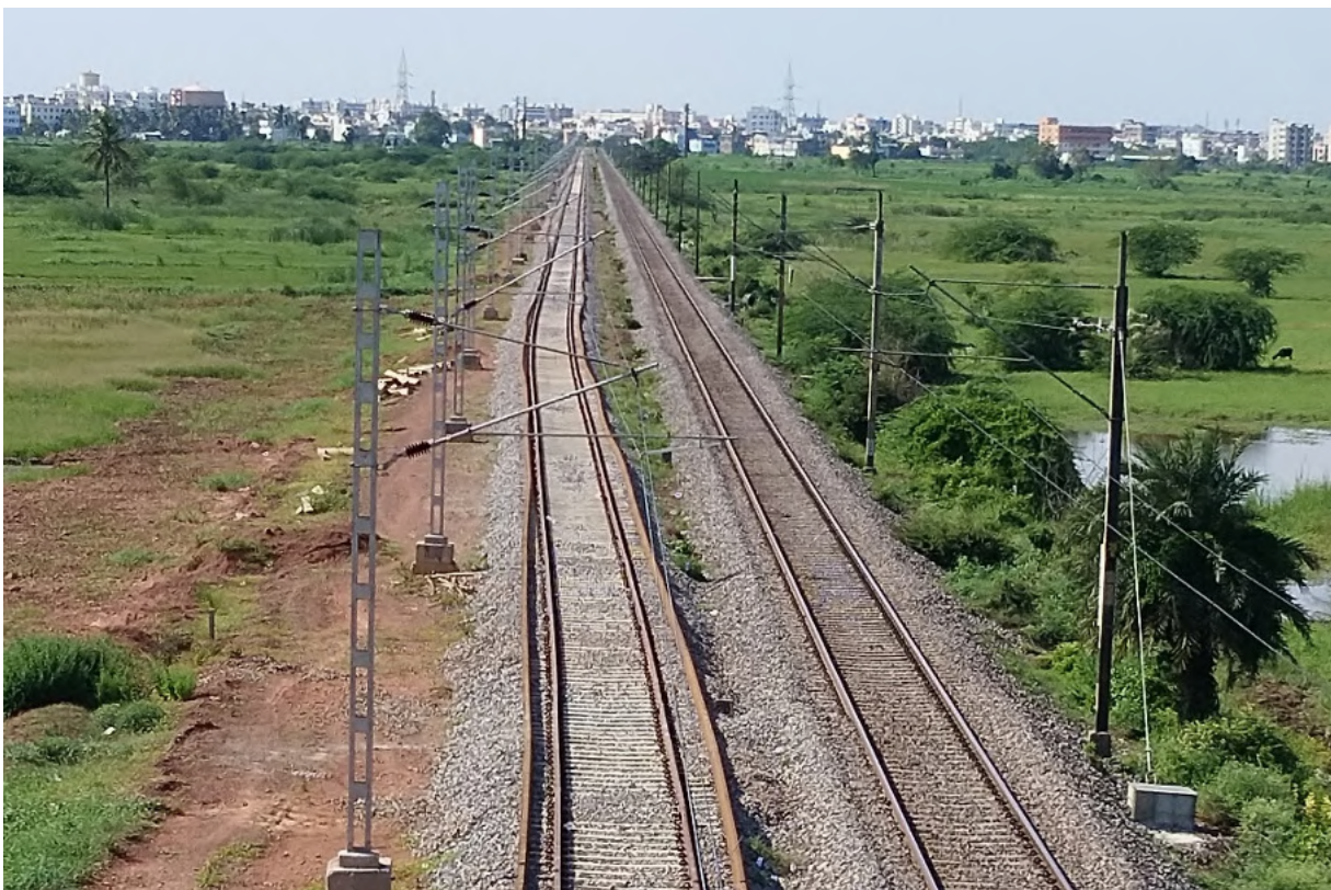
Guntur - Tenali Doubling & Electrification
