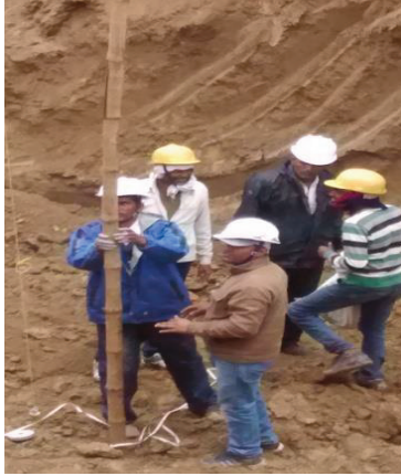
Approximate depth check by bamboo
