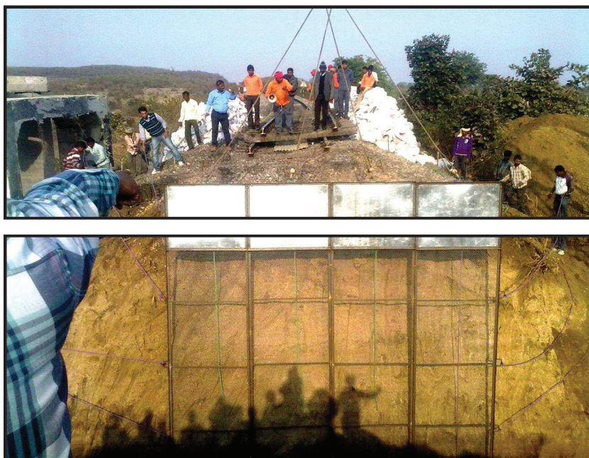
Protection screen being inserted during construction of LHS
