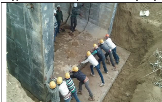
Alignment being adjusted prior to final placement
