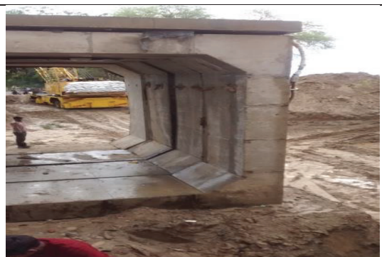
Pre cast slabs and RCC box segments
