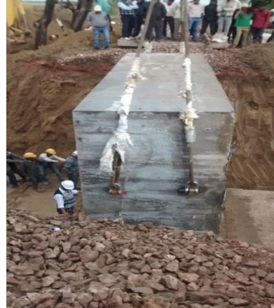
First RCC box segment being placed (to be placed with one edge at centre of track)
