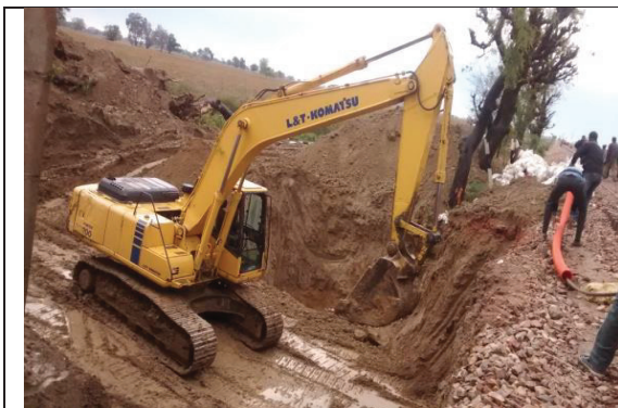
Cutting of slope prior to block
