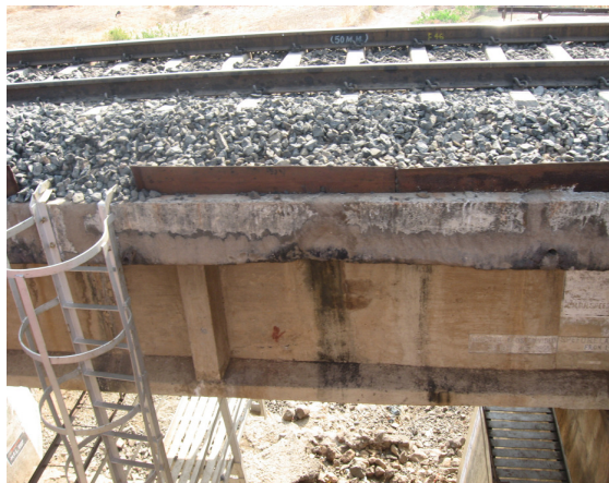
Figure 9: Arrangement for descending onto the inspection cradle from track
