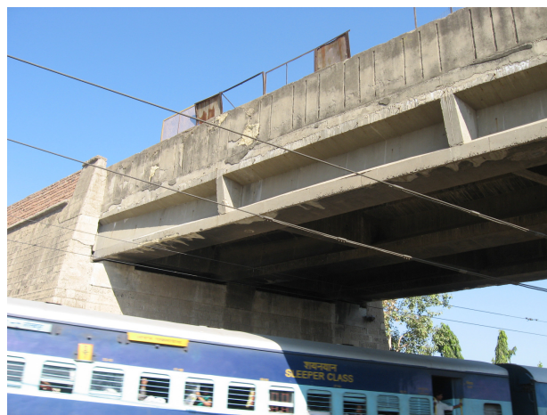
Figure 14: A typical Road Over Bridge in electrified territory
