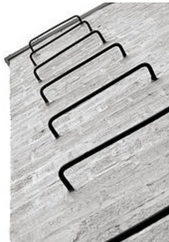
Figure 15: Steel rungs provided in sub structure
