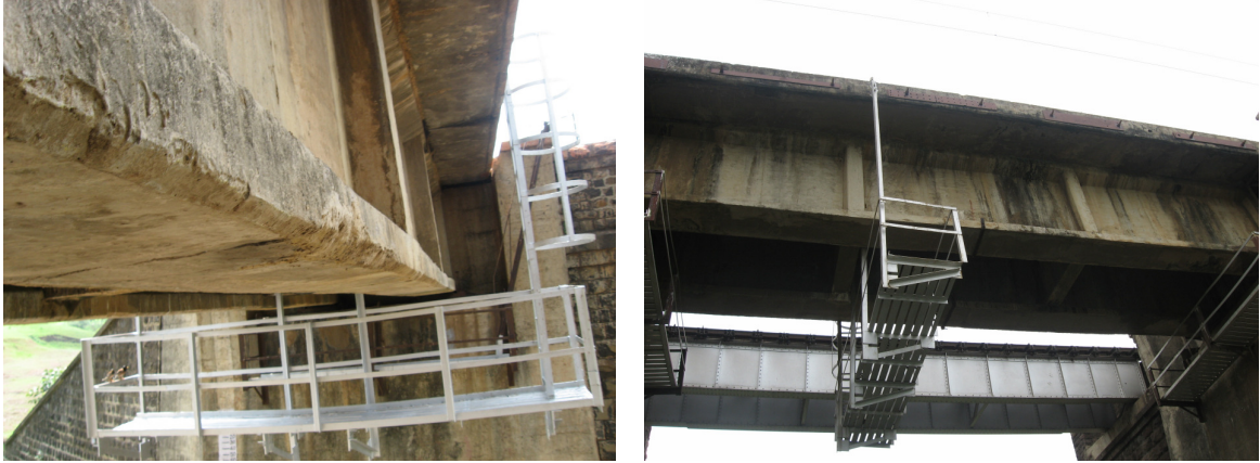
Figure 8: Front and side views of Inspection cradle at intermediate point of a PSC I-girder
