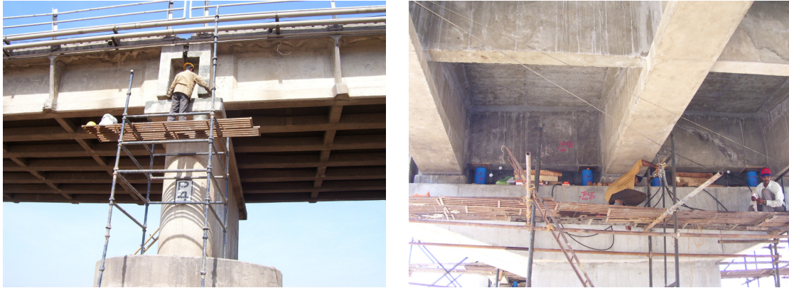
Figure 18: Scaffolding erected from ground/sub structure
