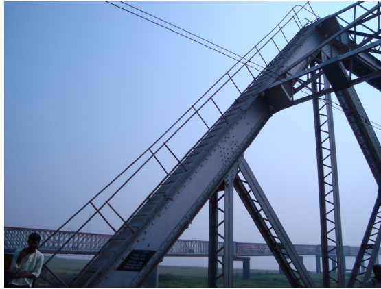
Figure 6: Ladder with railing on end raker of through type girder
