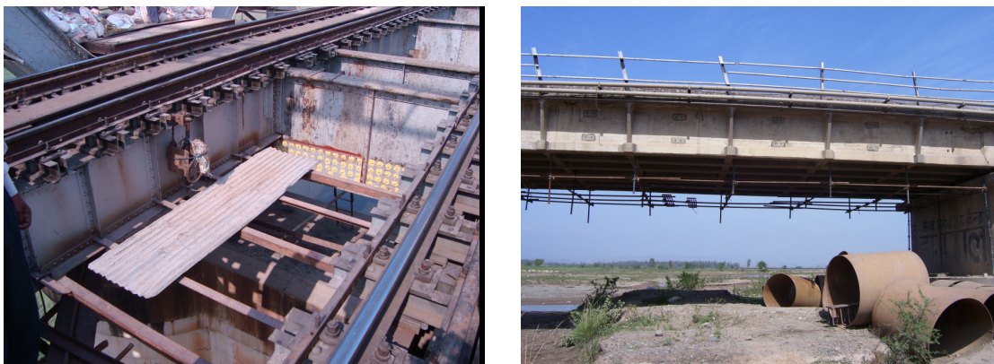
Figure 17: Steel/ bamboo scaffolding hung from the girder
