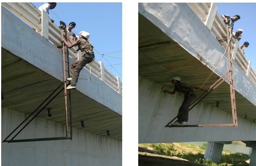
Figure 20: Temporary cradle erected from the hand railing. The hand railing shall be properly designed if such arrangement is to be used.
