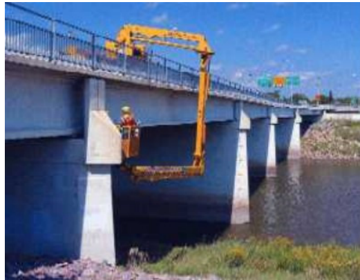
Figure 2: A track mounted vehicle used for inspection of underside of girder.
