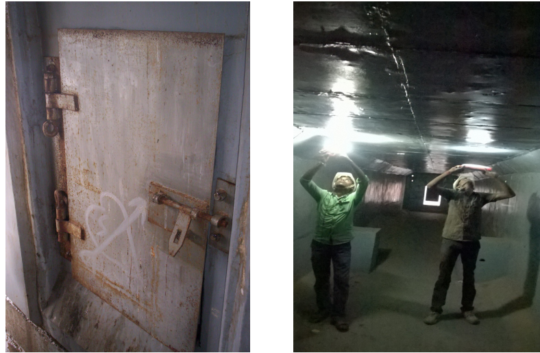
Figure 13: Door in a PSC Box Girder, and inspection in progress inside the girder
