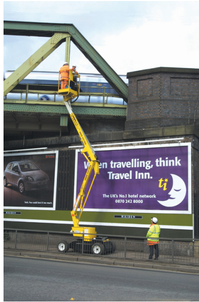
Figure 3: A road mobile vehicle being used for inspections.
