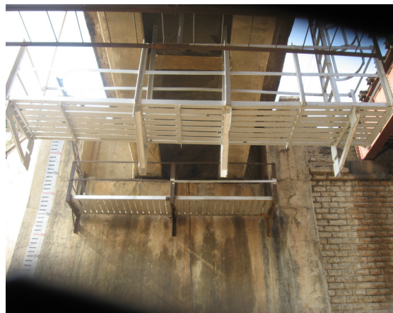
Figure 10: Cradles at intermediate point and abutment in a PSC I girder seen from underside
