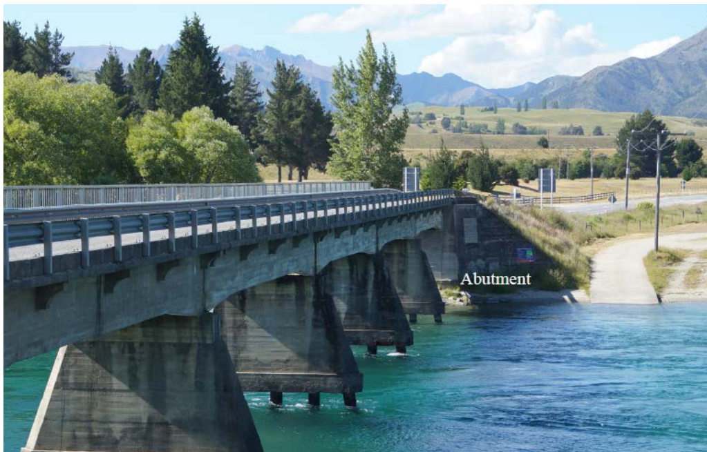
Fig. 1.6 Photograph of a wing wall abutment
