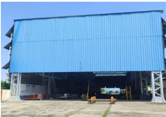
COACH LIFTING BAY WITH 30/5Ton & 5Ton cranes
