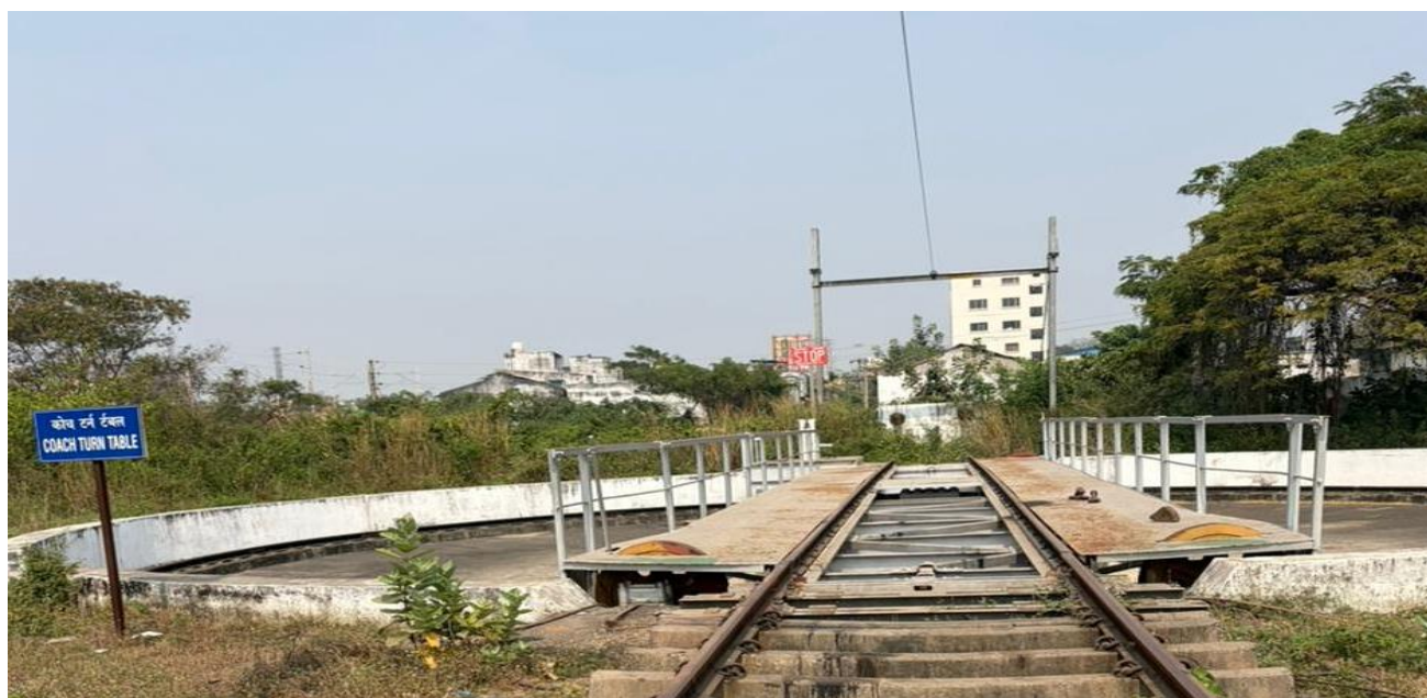
TURN TABLE: For changing of coach orientation
