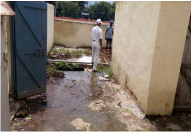
STAFF OF PURNA STATION PARTICIPATING IN CLEANLINESS STATION
