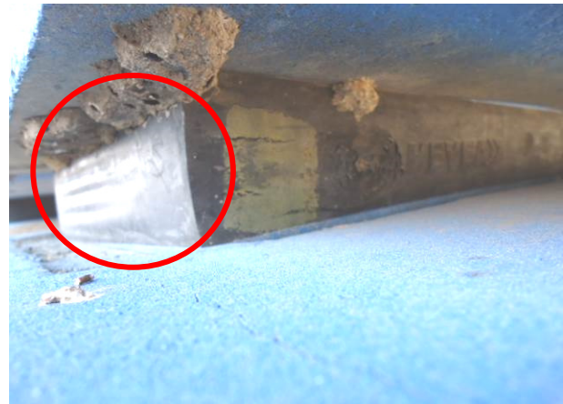
Bearing with separation of rubber from steel
