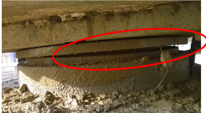
Gap in One side of POT PTFE Bearing
