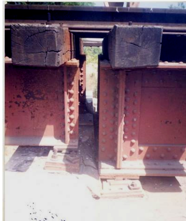
Bed plate missing holding down bolt; Cracked bed block with stool sunk
