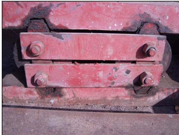
Close up of rollers (2 Nos per bearing)
