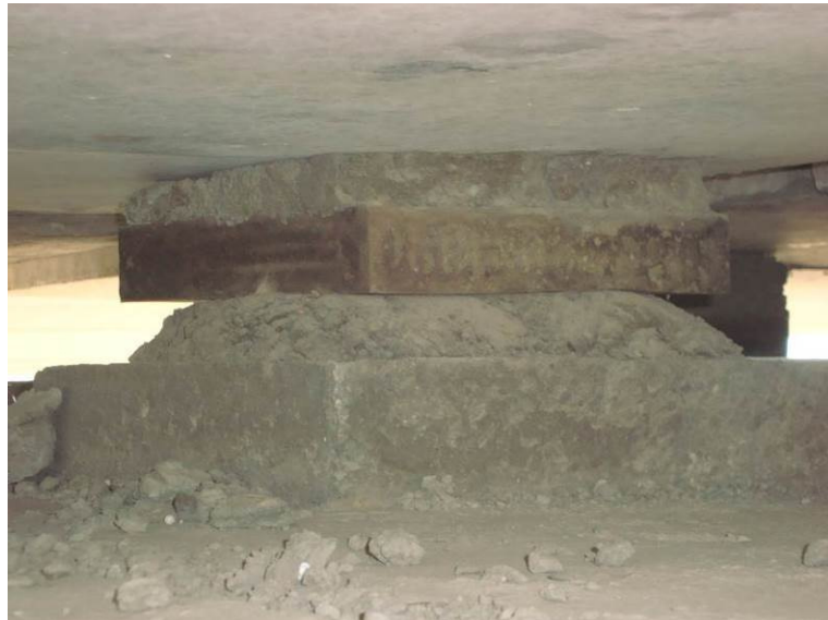
Defective epoxy concrete under a bearing
