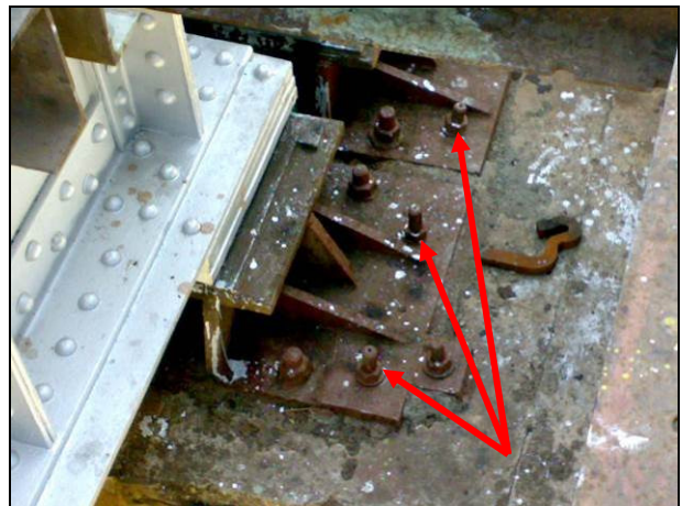
Extra Holding down bolts in extension of bed plate
