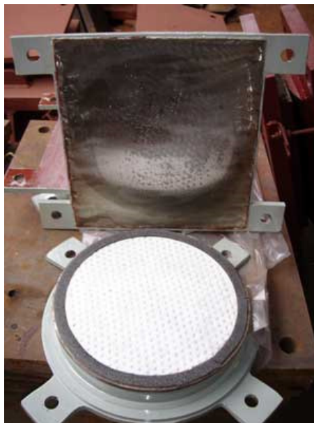
Sliding arrangement of a 'free' bearing- stainless steel as well as PTFE surfaces are seen
