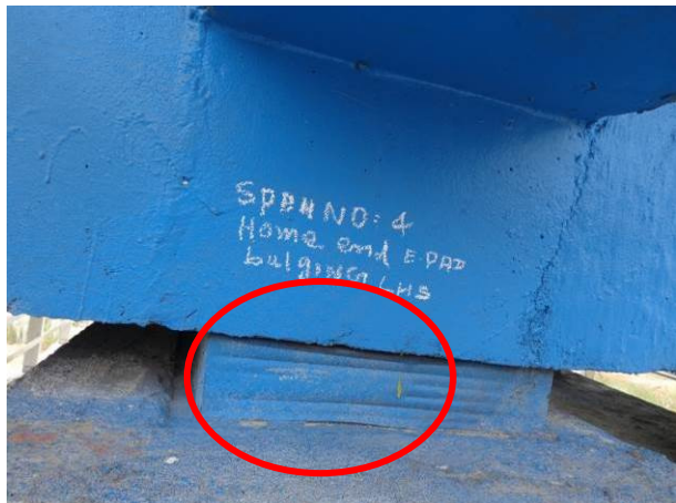
Separation of cover is seen in middle portion
