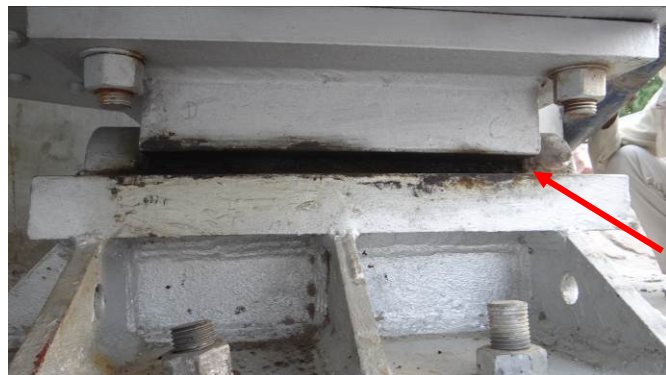
Improperly seated rocker
