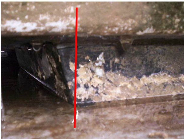
A tilted bearing (The tilt from vertical shall be quantified);
