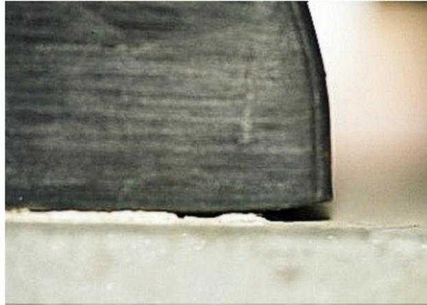
Bearing with edge off-loaded
