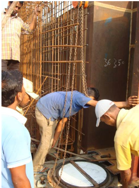
Wrong practice - Bearing opened during installation
