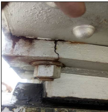
Cracked saddle of roller-rocker bearing;
