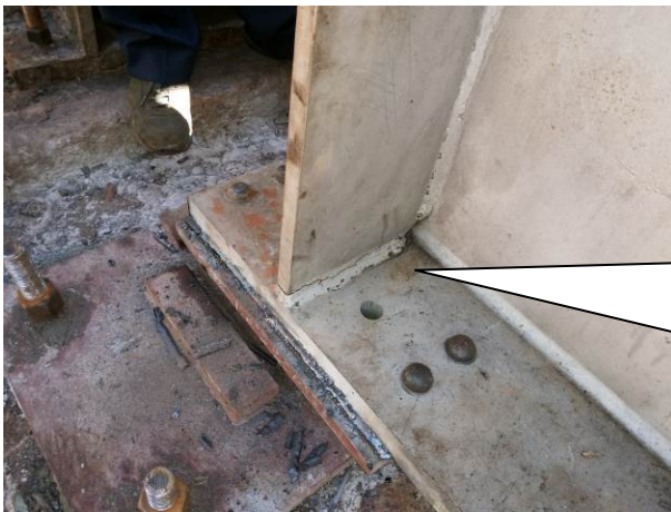
Crack in weld connecting bearing stiffener to bottom flange
