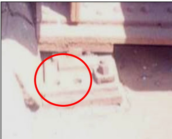
Missing holding down bolt;
