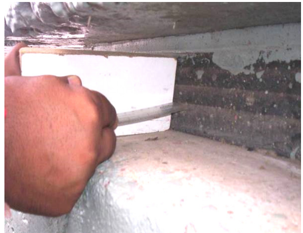
Bulging being measured with wooden straight edge & scale
