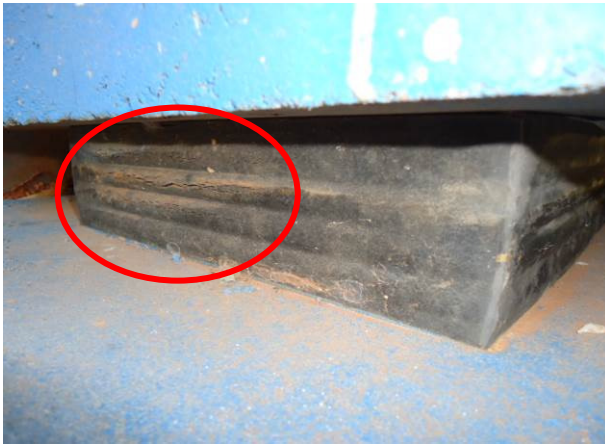
Tilted Bearing with rubber cracked in one layer;
