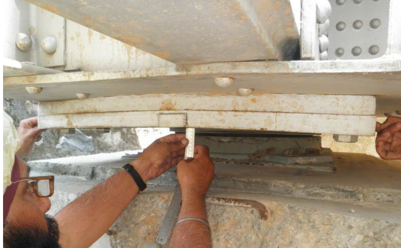
Top Plate of bearing developed upward convexity due to bending
