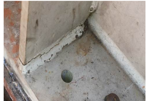
Corroded and bulged sliding bearing and bearing stiffener – cracks may also be there
