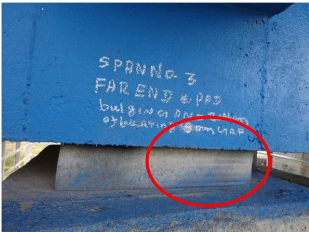
The far edge of bearing is having more load (as seen by deformation of rubber layers)
