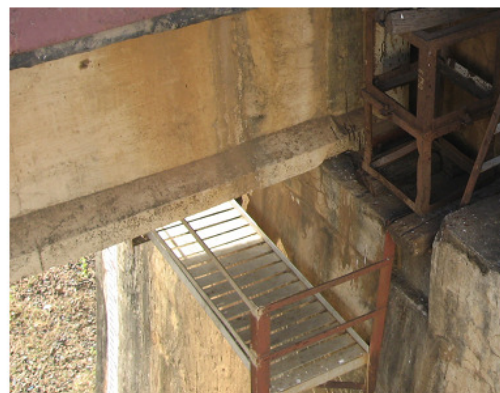
One type of arrangement for inspection of bearings (Schematic and actual)
