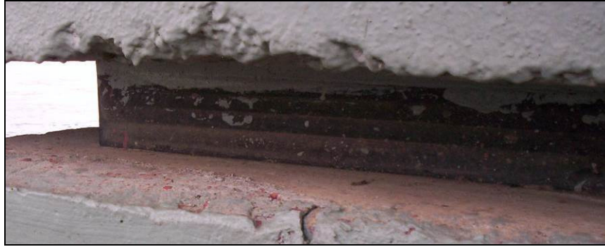
Elastomeric bearing under PSC girder
