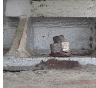
Packing under nut to make holding down bolt effective
