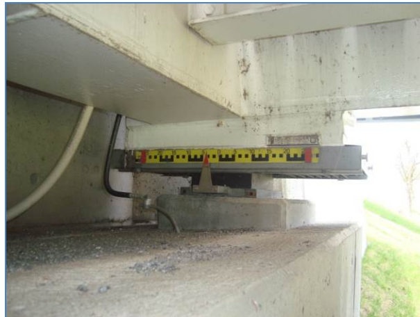
Pointer provided in an elastomeric bearing to indicate movement of superstructure
