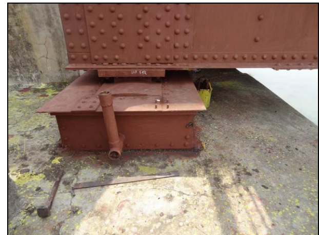
Rollers enclosed in oil bath
