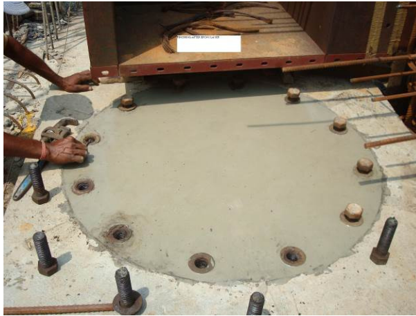
Holes in sleeves being cleaned for installation of bearing
