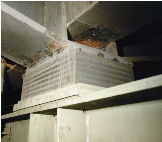
Typical Elastomeric Bearing;
