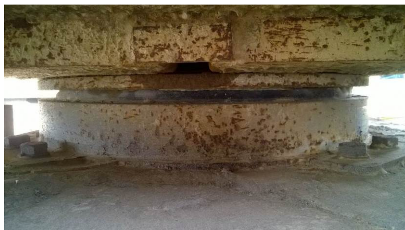
A bearing with corrosion initiated
