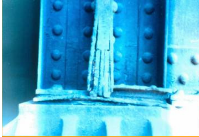
Corroded and bulged sliding bearing and bearing stiffener – cracks may also be there
