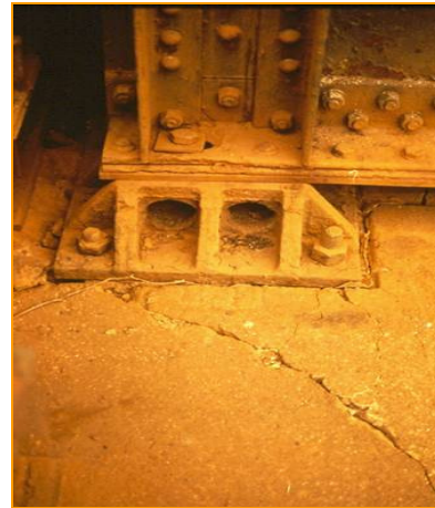
Bed plate missing holding down bolt; Cracked bed block with stool sunk
